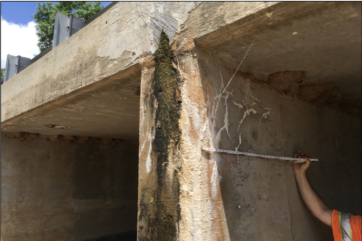
Division wall #3 has map cracking with efflorescence.
