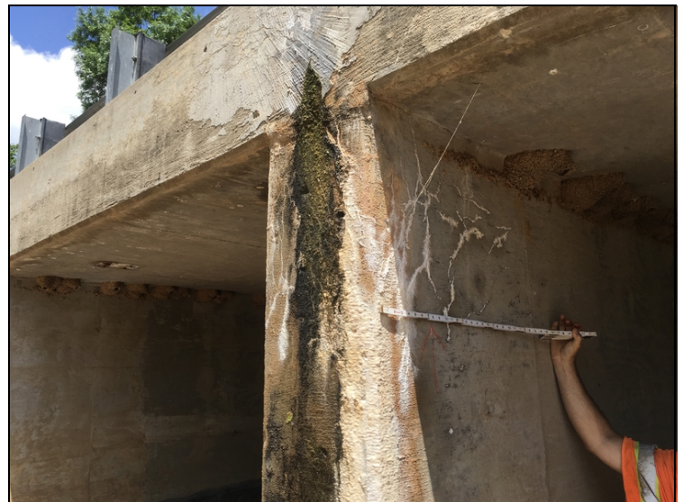
Division walls #3 on the down stream side have map cracking with efflorescence leaching.
