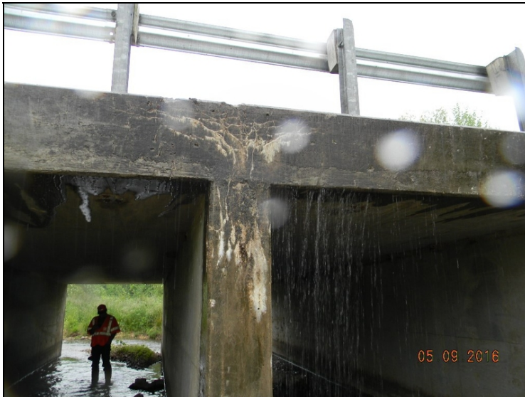
Headwall between barrels 5 & 6 - Cracking and leaching.
