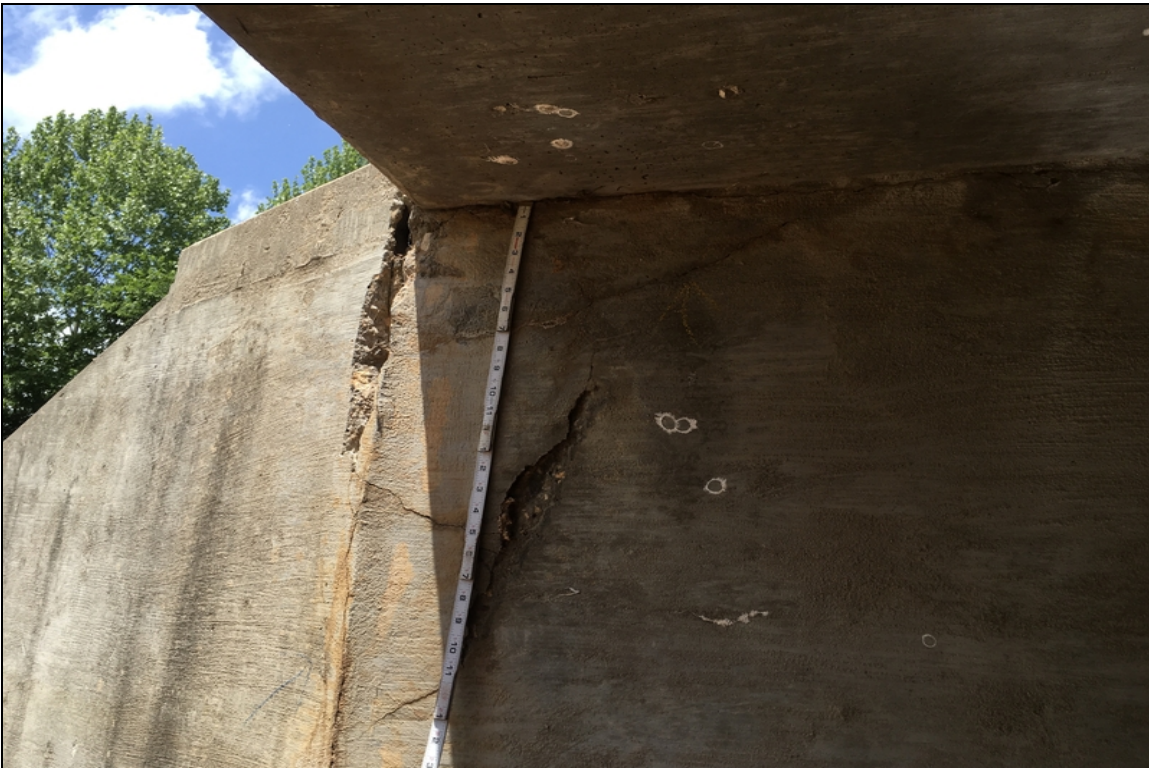
2' x 1' delamination in the backwall of barrel #1 at the outlet end.
