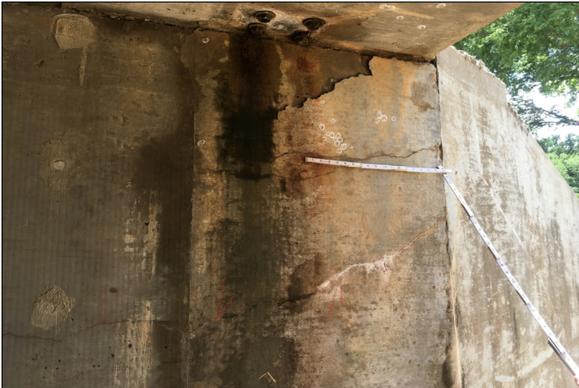
2'x 1' delamination at inlet and outlet end of barrel #12 backwall.
