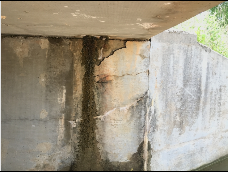
Barrel #12 wall #13 right side at the southwest wingwall juncture large eliminated area.
