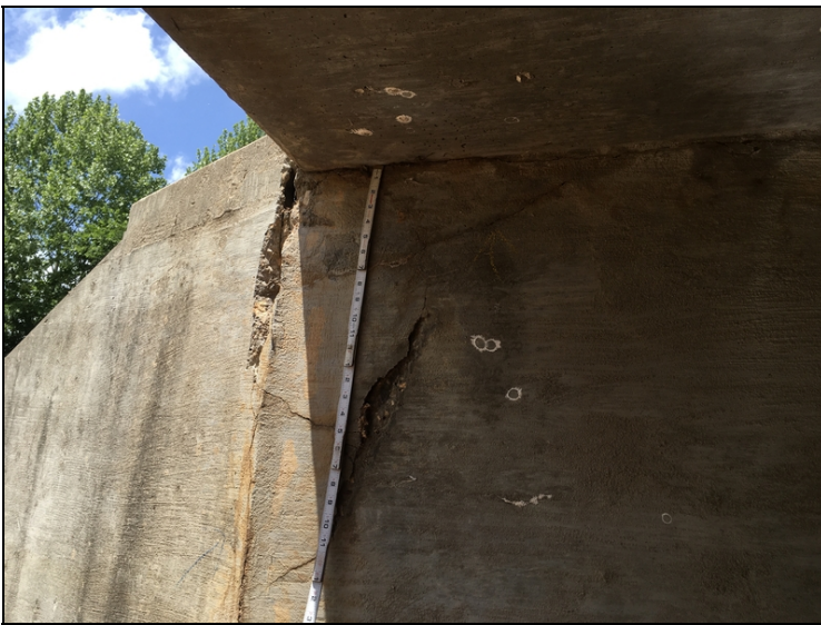
Barrel #12 has a delamination at the top corners at the inlet and outlet ends.
