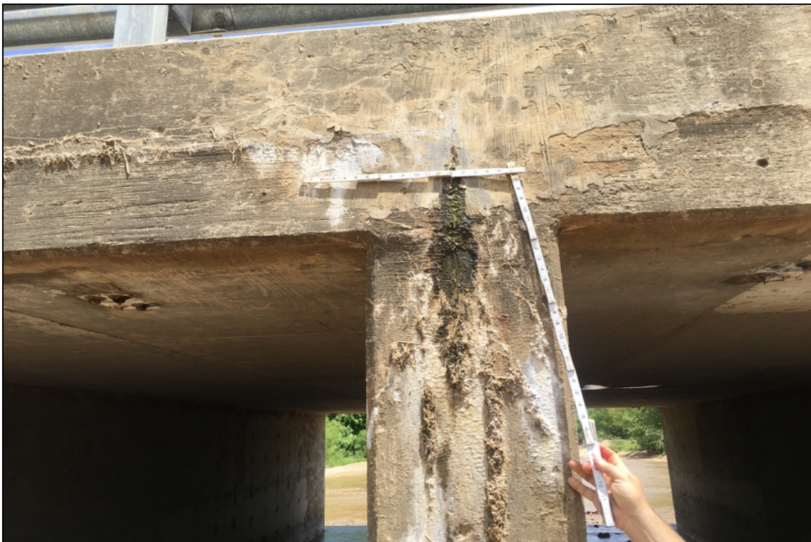
Division wall #6 has map cracking with efflorescence at the outlet end.
