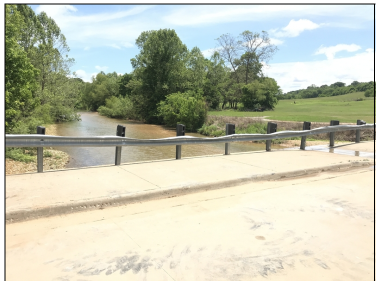
Railing left collision damage
