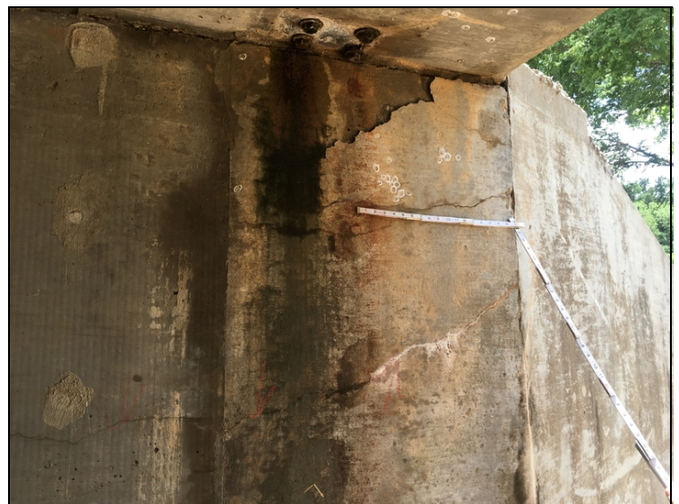
Barrel #1 has a delamination at the top right corner at the outlet end.
