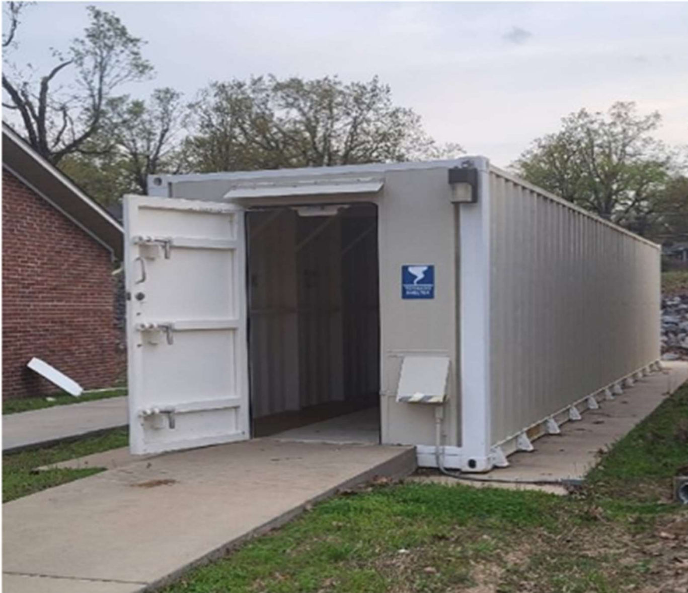
Community safe room funded through the HMGP program used in North Little Rock during the March 31 tornado.
