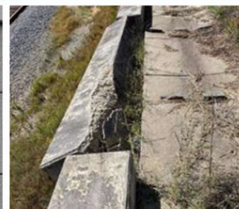
Coping deterioration
