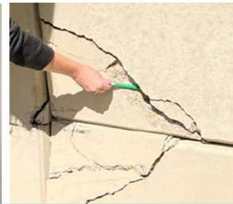
Structural cracking
