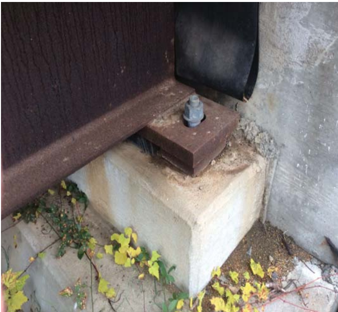
PHOTO 1 Description Abutment #1 left anchor bolt backed out.
