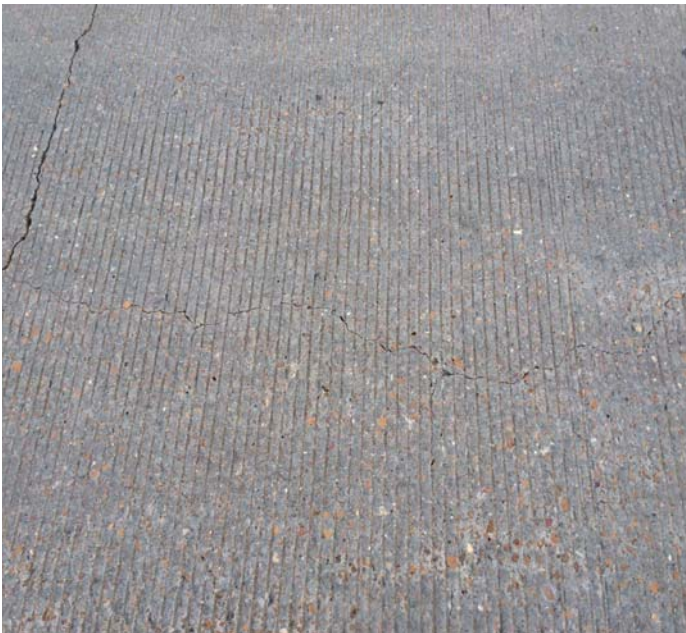
PHOTO 1 Description Abutment #1 approach slab typical transverse and longitudinal cracks.
