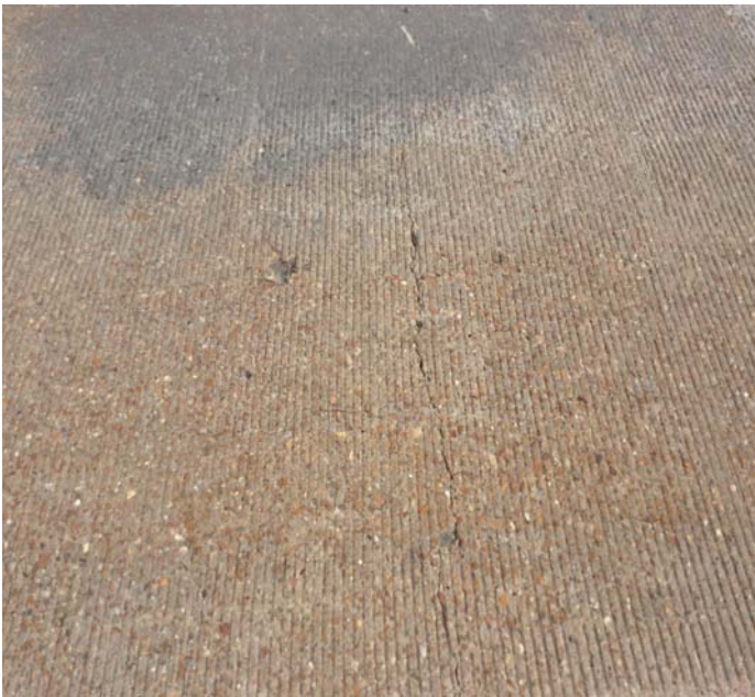
PHOTO 1 Description Typical transverse deck crack
