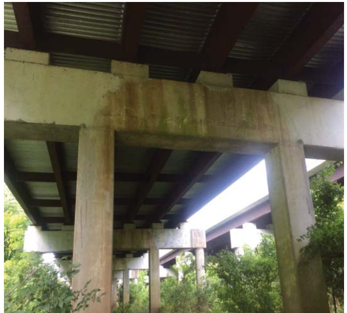
PHOTO 2 Description Bent #12 cap and column 2&3 cap condition typical for other caps in report
