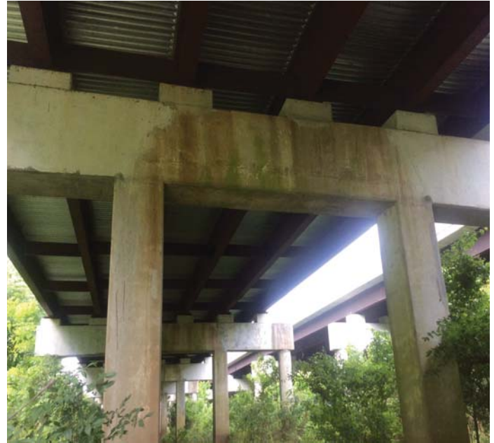
PHOTO 5 Description Bent #12 cap and column 2&3 cap condition typical for other caps in report
