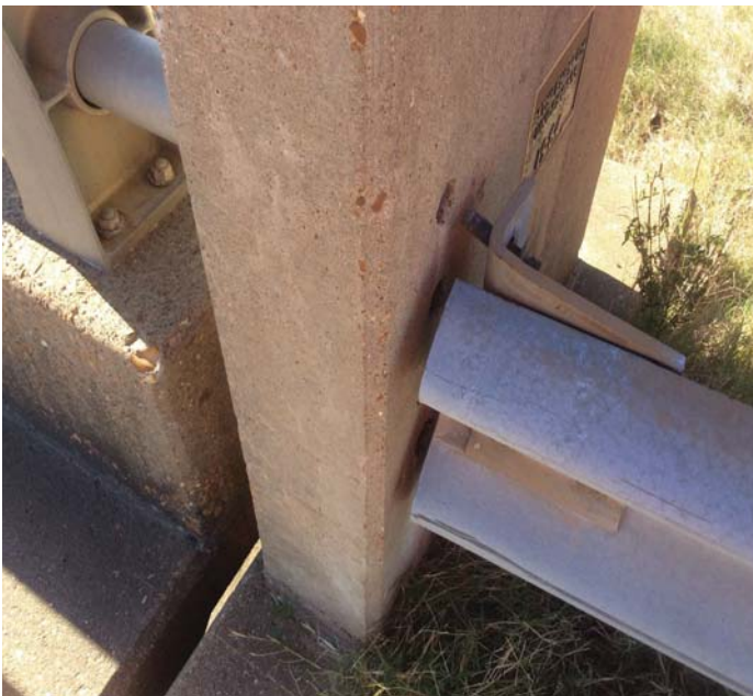
PHOTO 1 Description Abutment #1 right approach rail loose at bridge end
