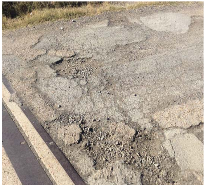
PHOTO 2 Description Holes in abutment #1 approach roadway
