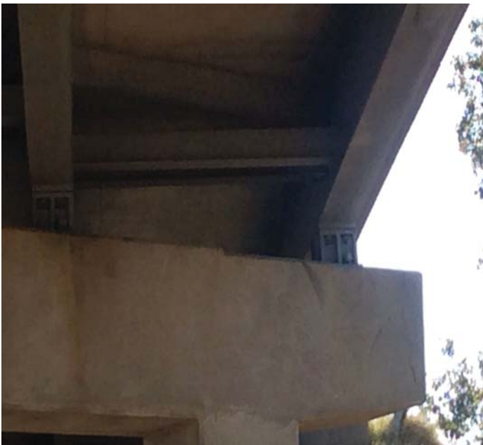
PHOTO 1 Description BENTS #2&4 FIXED BEARINGS ANCHOR BOLT NUTS ARE LOOSE
