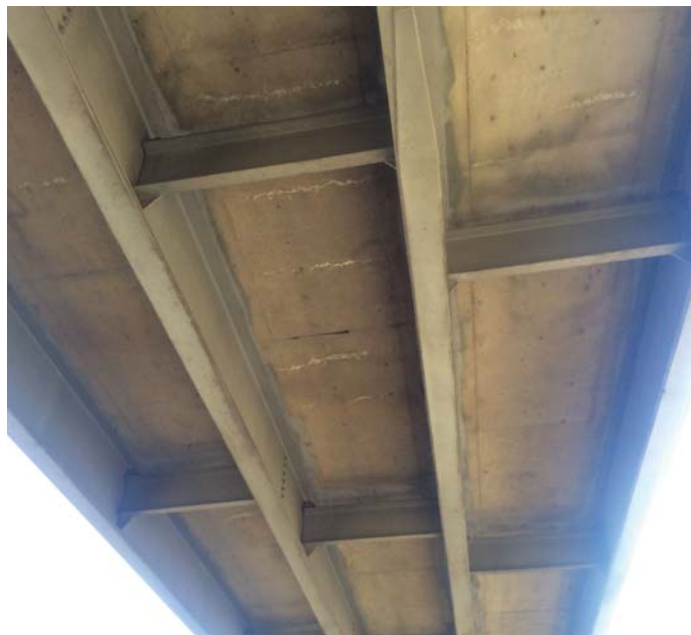
PHOTO 1 Description Transverse deck cracks reflecting through to soffit with efflorescence spaced 3'
