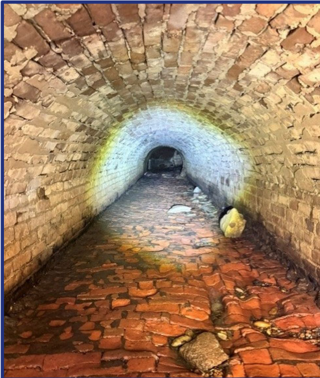
Brick Drainage Culvert
