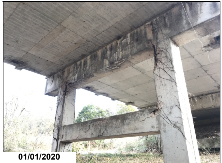
Bent 3 back side Cap, Columns & Diaphragm have large spalls with rebar exposed, Large areas of delaminations, & efflorescent cracks with rust stains.
