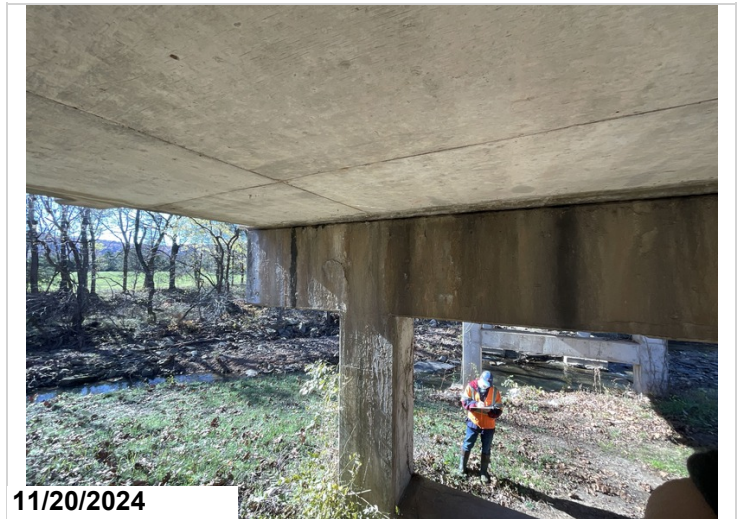
Bent 4: Back and Ahead sides: Vertical and horizontal efflorescent cracking. 6' CS3
