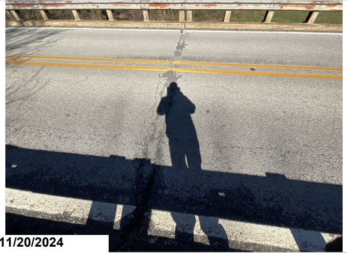
The wearing surface has cracks at all joints. 144SF CS3
