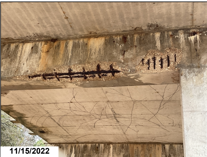
Bents 2 & 4 - Large spalls with rebar exposed. Rebar has 100% section loss.
