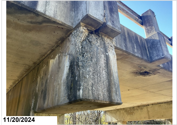
Bent 4: Bottom: Spall with corroded reinforcing steel exposed. 1' CS3
