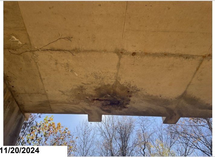
Span 4 :Left and Right drains: Spalls with corroded reinforcing steel exposed. 6' CS3
