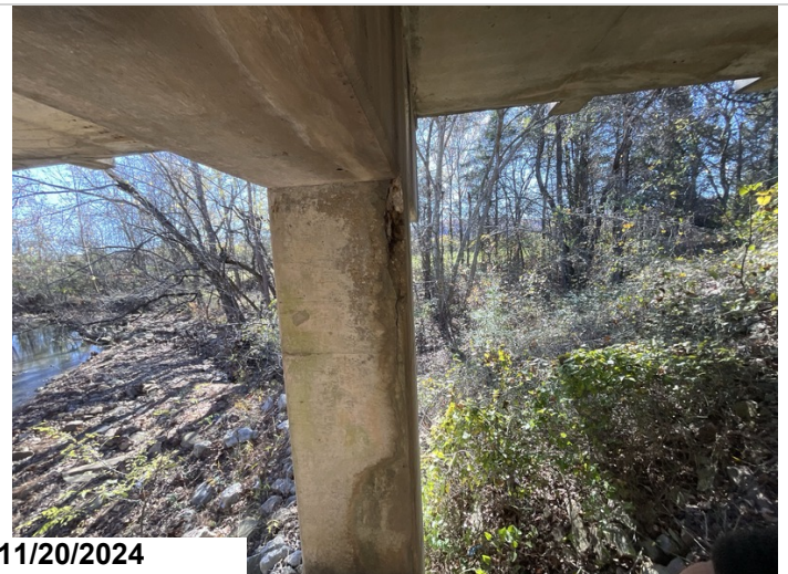
Bent 1, column 2: exposed rebar. 1EA CS3
