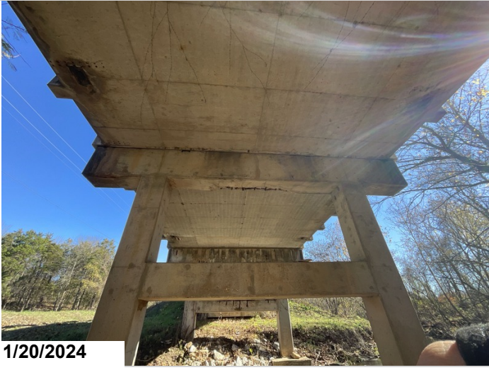
Bent 2: Ahead: Horizontal efflorescent cracking. 3' CS3
