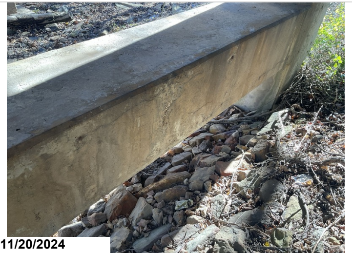
Bent 1, back: horizontal cracking. 6LF CS3
