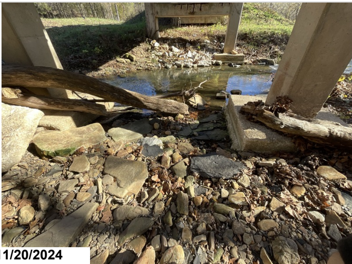
Bent 2, both footings exposed.
