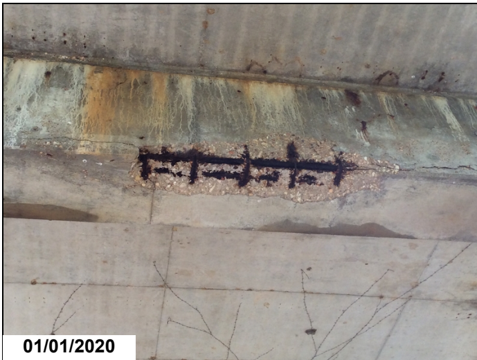
Spalls with rebar exposed to bottom of cap @ Bent 2.
