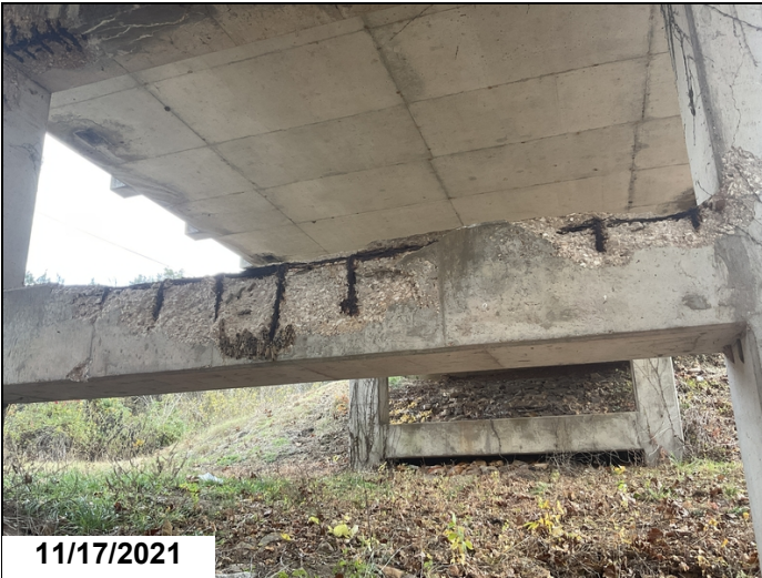
Bent 3 - Large spall w/ 3' of rebar exposed and efflorescent map cracking w/ rust stains to cap & Lt. & Rt. columns and diaphragm.
