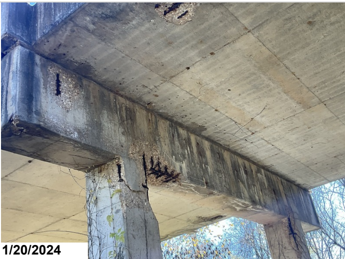
Bent 3: Backside/bottom: Efflorescent map cracking. 10' CS3
