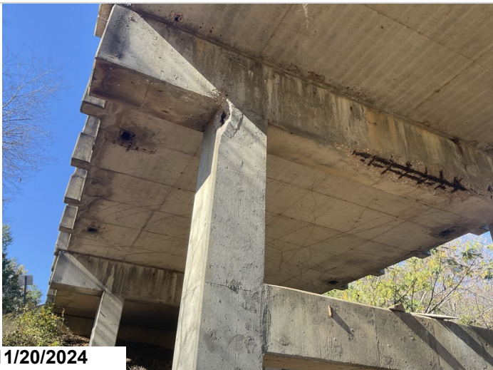
Bent 2, column 1: has exposed rebar. 1EA CS3
