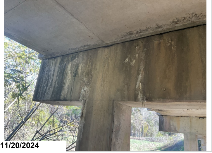
Bent 1: Back and ahead sides: Efflorescent cracking. 13' CS3
