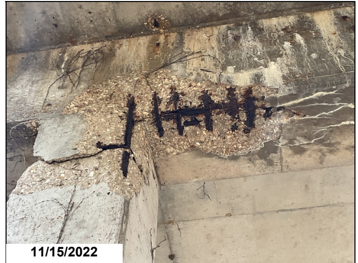
Bent 3 - Large spall w/ 3' of rebar exposed and efflorescent map cracking w/ rust stains to cap & Lt. & Rt. columns and diaphragm.
