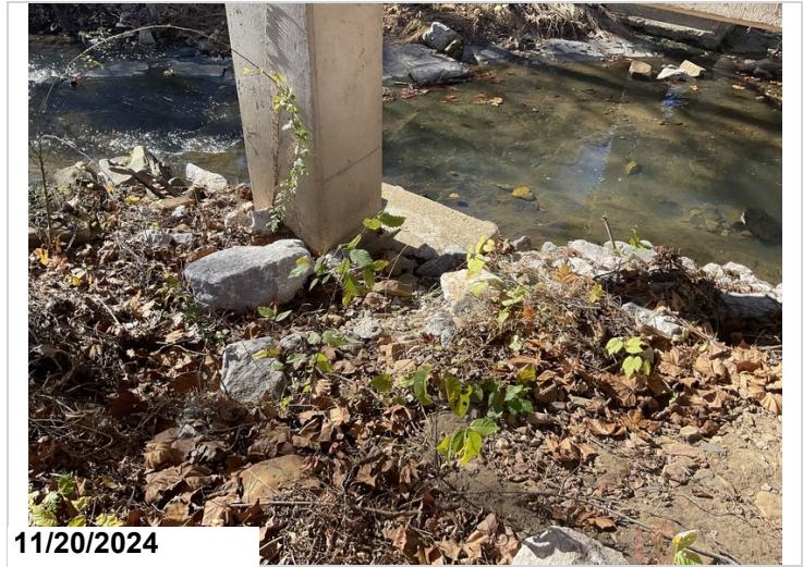
Bent 3, right: has an exposed footing.
