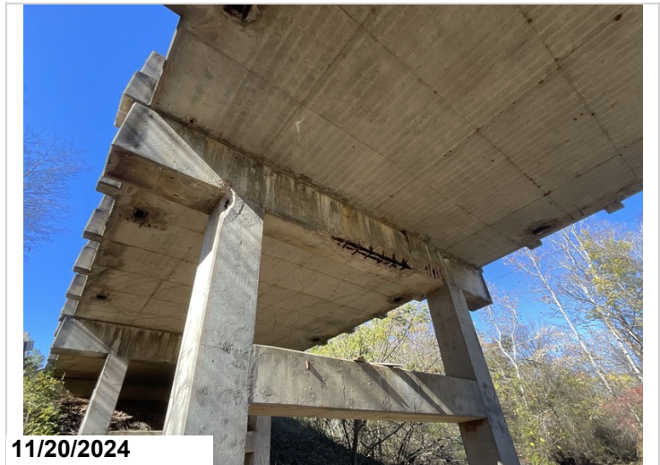
Bent 2: Ahead: Spalls with corroded reinforcing steel exposed, some with 100% section loss. 10' CS3
