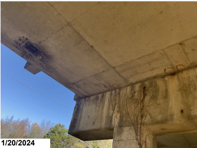
Span 4: Efflorescent cracking. 5' CS3 4' CS2
