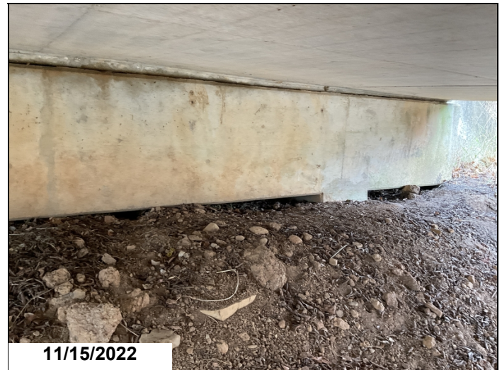
Abutment 1: Scour 1' down and 2.5' back under exposing 1 column.
