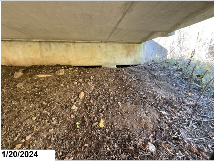
Abutment 1, left: has scour under the cap with a column exposed. 1' down, 2.5' back under. 25LF CS2
