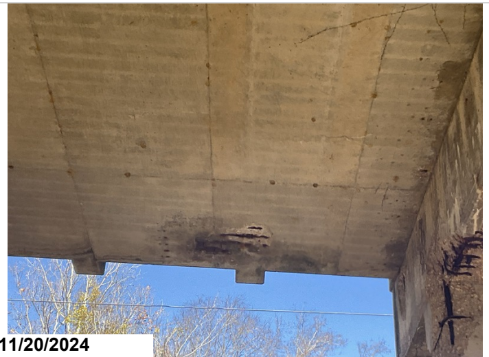
Span 3: Left drain: Spalls with corroded reinforcing steel exposed. 4' CS3
