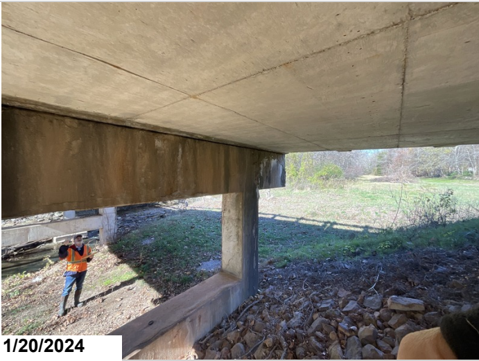
Bent 4: Ahead Left: Spall. 1' CS3
