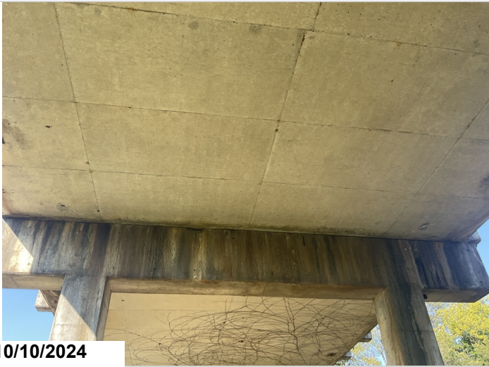
Span 6, ahead of bent 5: typical efflorescence in the undersurface.
