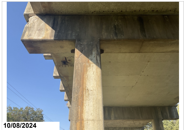
Bent 6, ahead, column 2: has large delams and vertical cracks. Column 1 is similar 2EA CS3
