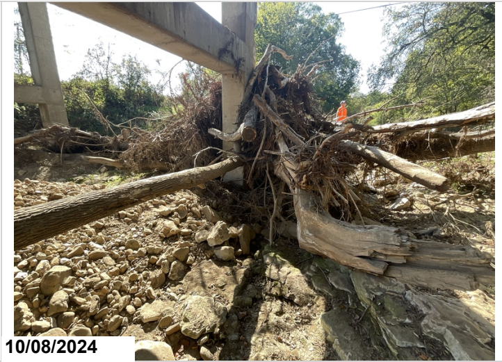
Bent 2, column 2: has a large pile of accumulated debris that is creating a scour hole.
