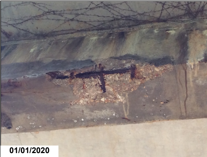
Spalls with rebar exposed to bottom of Cap @ Bent 3.
