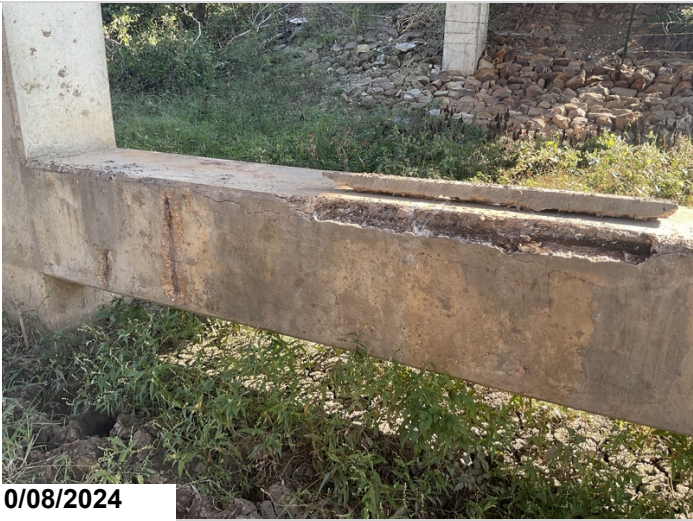
Bent 6, back, pier wall: has exposed rebar typical of this element.
