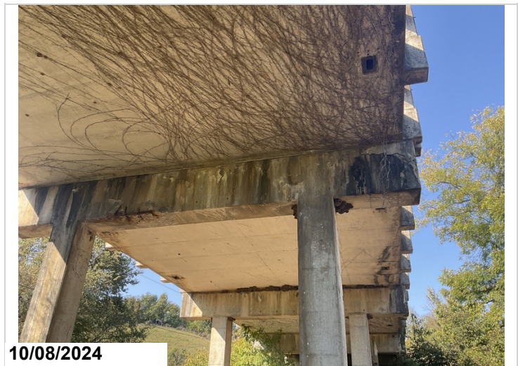
Bent 3: has a large spall with exposed rebar. 5LF CS3
