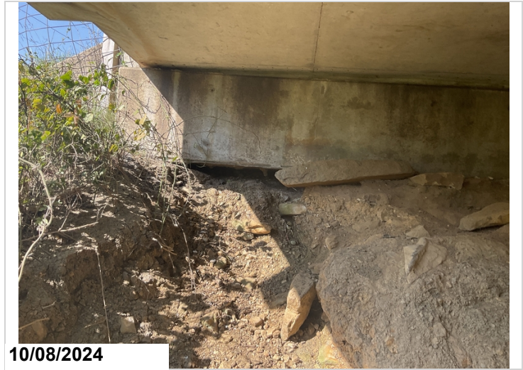
Abutment 1, right: has scour with undermining. 8LF CS2
