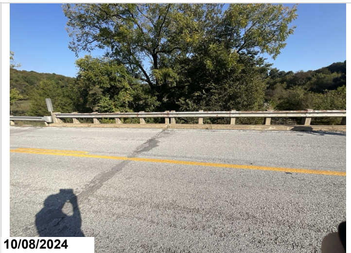
Typical rail is in satisfactory condition with surface corrosion.
