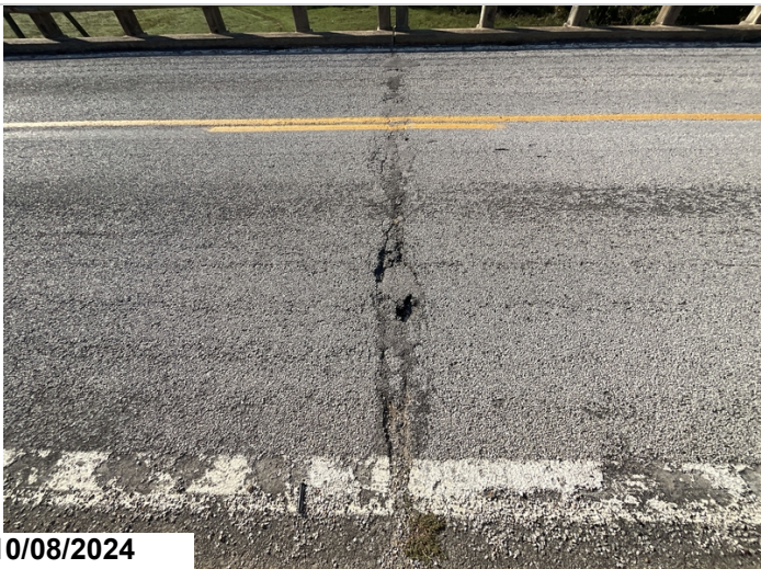
Bent 5, left: has a spall in the wearing surface typical of joint locations. CS3
