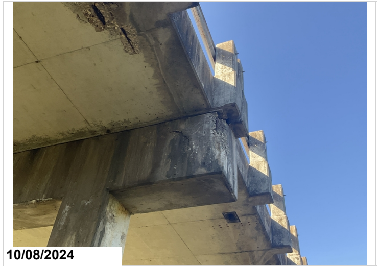
Bent 6, left: has a spall with exposed rebar. 1LF CS3
