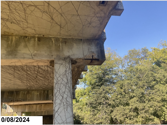
Bent 4, left: has exposed rebar. 3LF CS3
