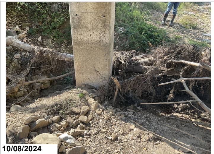
Bent 3, column 2: has drift accumulation and minor scour. 1EA CS2
