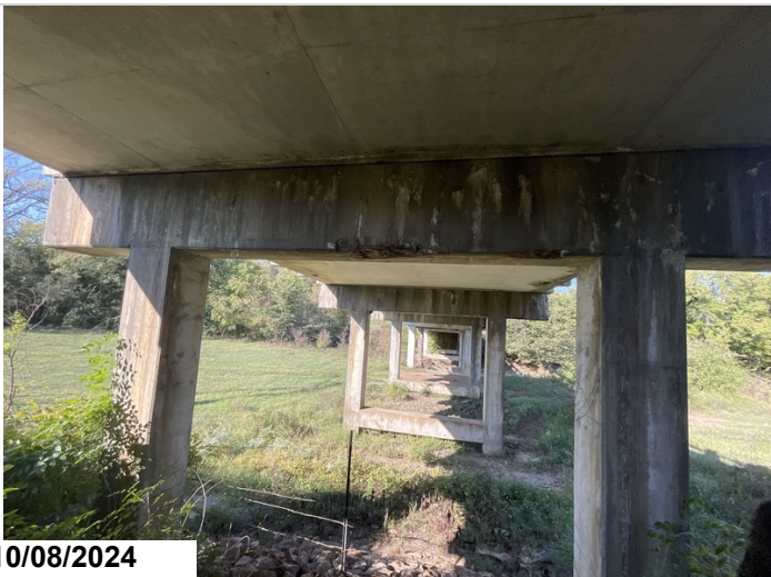
Bent 7: has a spall with exposed rebar on the underside. 6LF CS3
