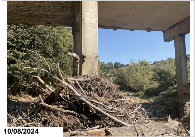
Bent 2, column 2: has 2 deep spalls with exposed rebar. 1EA CS3
