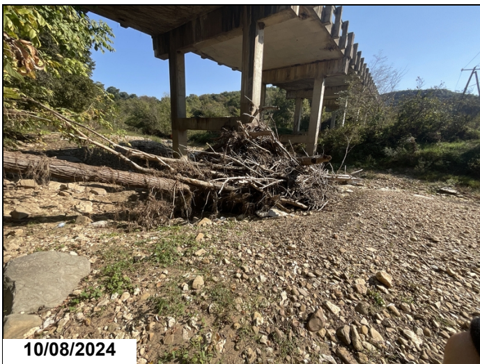
Bent 2: typical debris.
