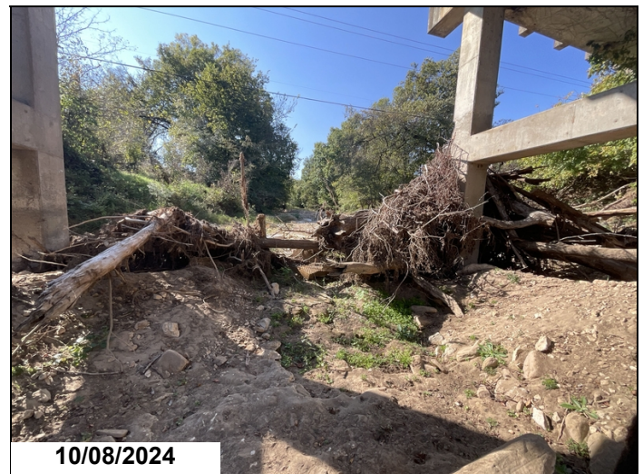
Bents 1 2 and 3 have excessive debris causing scour
