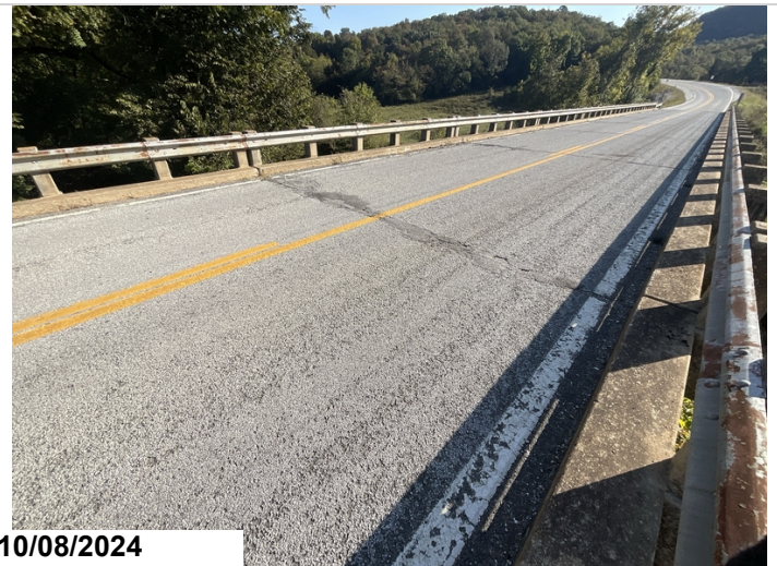
Typical wearing surface has cracks and patches over joints.
