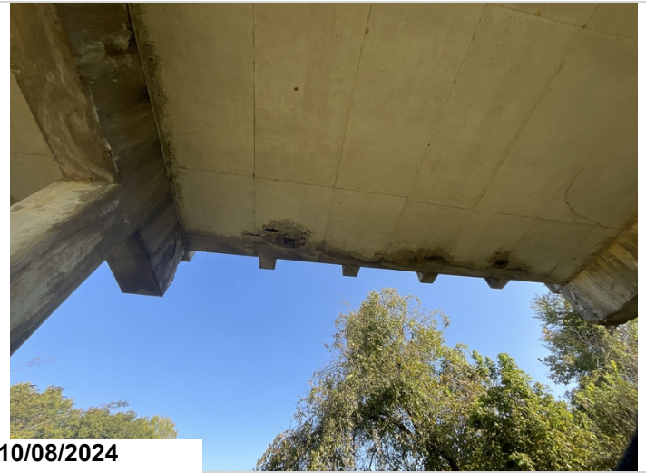
Span 7, left, first drain: has spalling with exposed rebar typical of drain locations throughout. 3SF CS3
