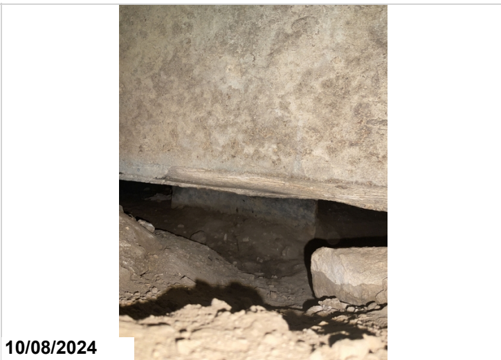
Abutment 1, center: has scour with undermining and an exposed pile. 2LF CS2
