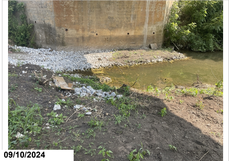
Rip rap has been placed at abutment #2 as a work platform.
