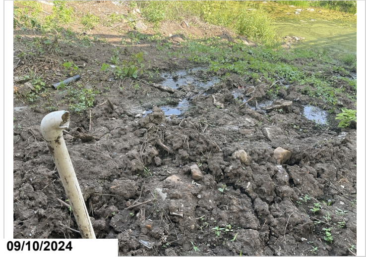
Possible sewage leak at abutment #1.
