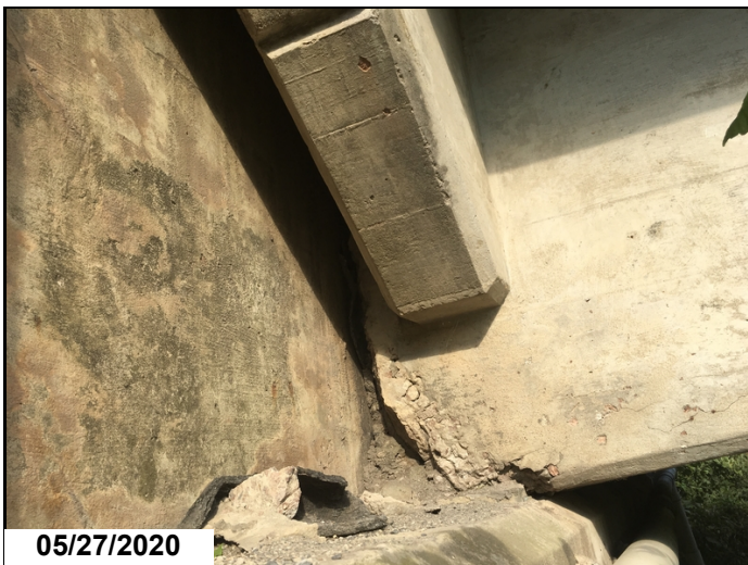
View of the exterior bearing area of beam #2 over abutment #1. Showing deterioration and crushing. The bottom edge of the tee is nearly in contact with the top face of the abutment
