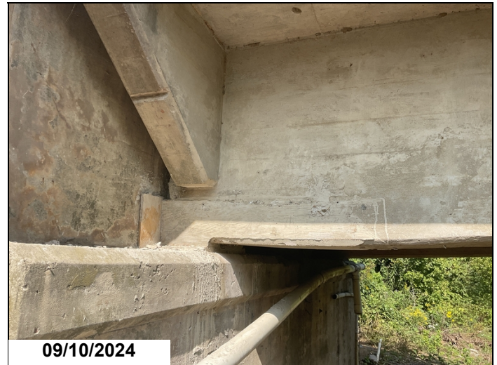
Tee beam #2 over abutment #1 has been repaired.
