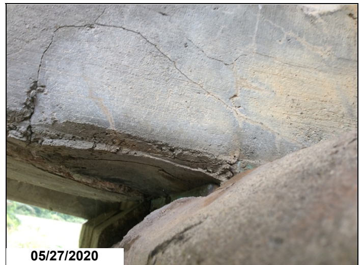
Small amount of Crushing at girder#2 at abutment #2.
