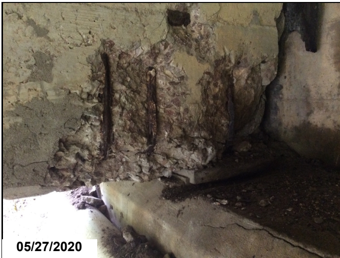
Inside view of girder #2 over abutment #1
