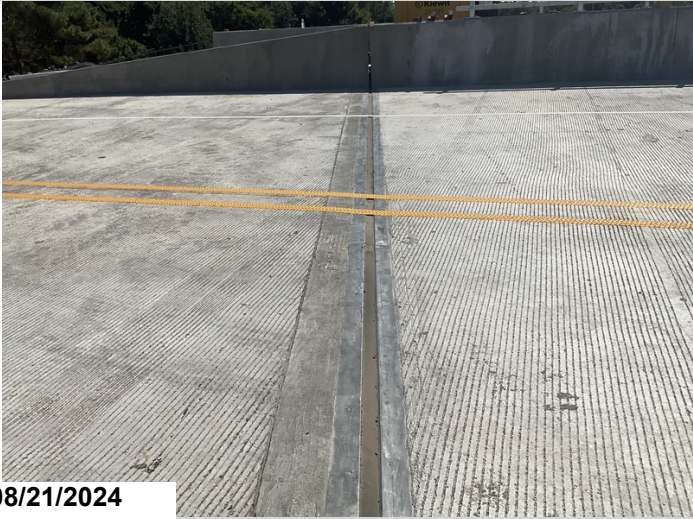
Bent 3 pourable joint seal.
