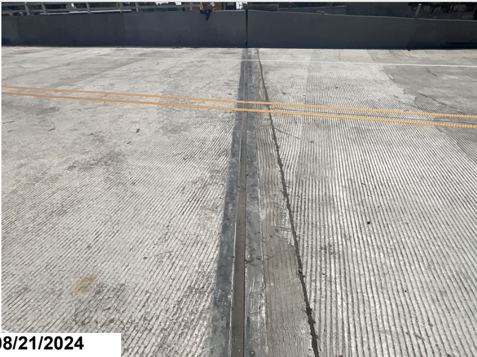
Bent 1 pourable joint seal.
