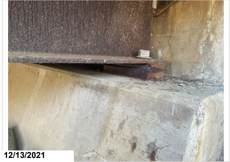
Bent 1 bearing 1 laminated rust
