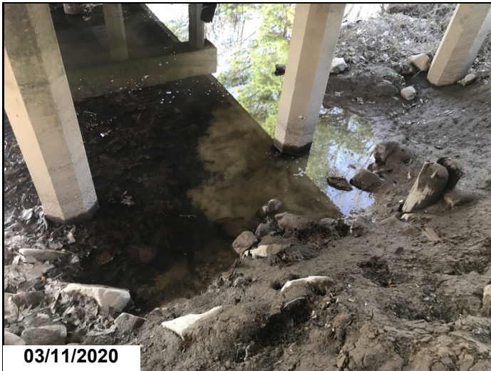
Bent 3, piles 2 & 3: local scour at this location
