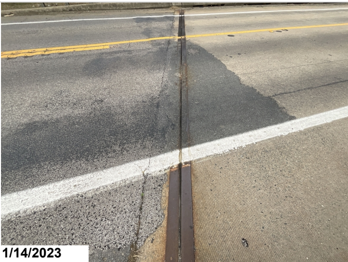
Bent 1 joint seal
