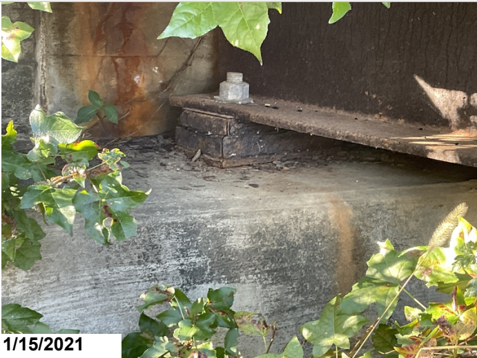
Bent 1 laminated rust on bearing 5
