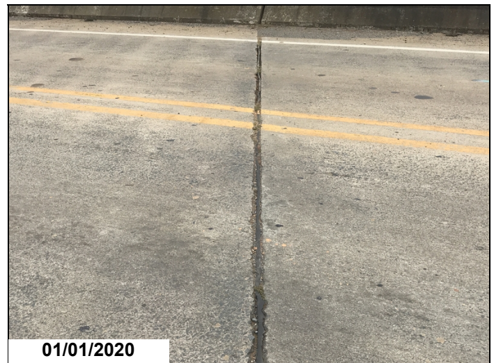
Bent 4: joint seal has lost bond and is full of non compressible material
