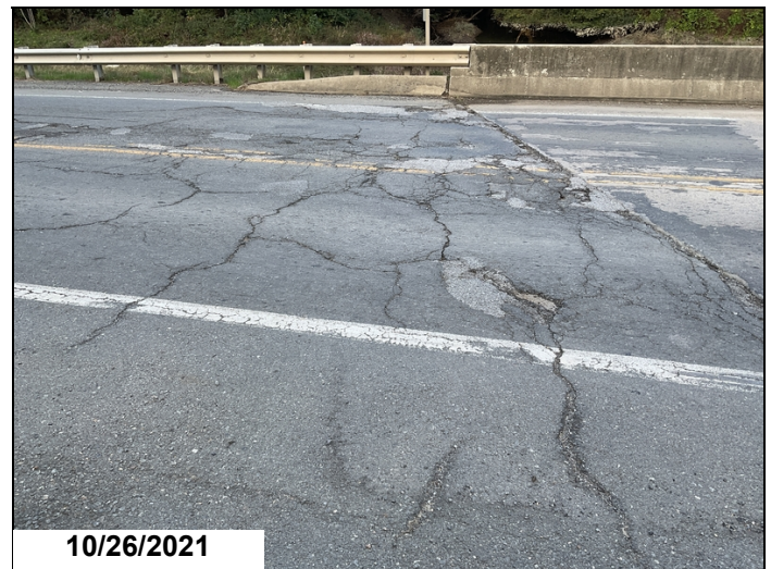
Approach roadway on south end of bridge has settled and has pot holes.
