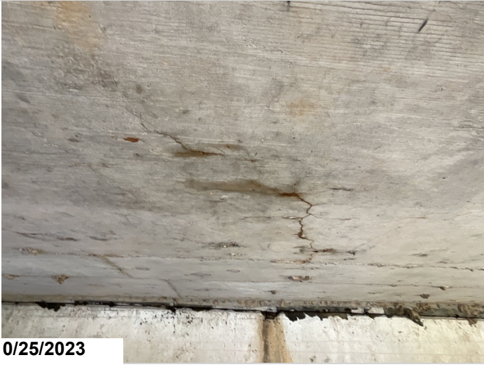
Cracks in the soffit with rust staining
