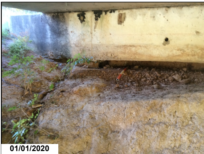
Bent 1, looking back at the right side. Erosion has begun to undermine the abutment.
