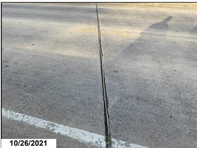
Bent 4, looking left. The joint has opened and begun to fill with non-compressible material.
