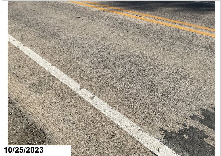
Sealable deck cracks
