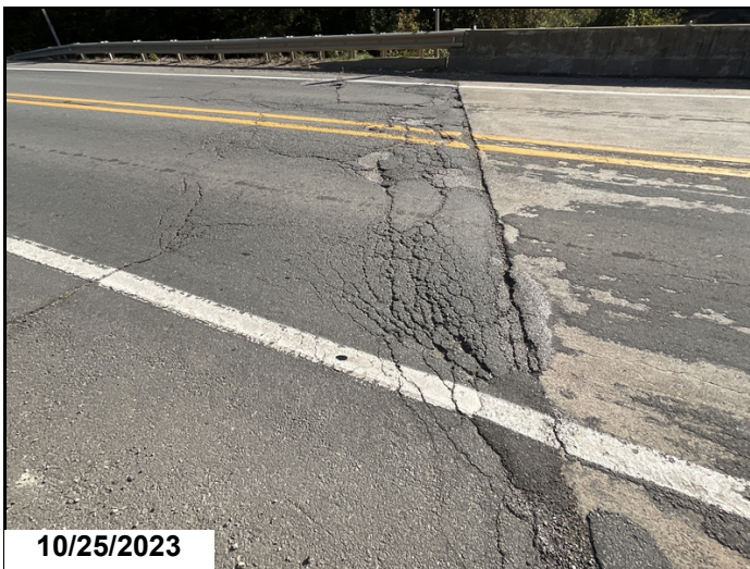
Potholes at bent 6
