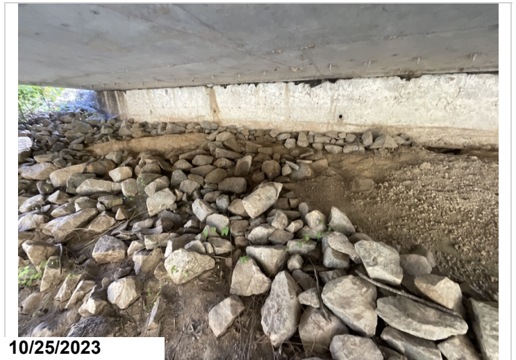
Rip rap placed at bent 1
