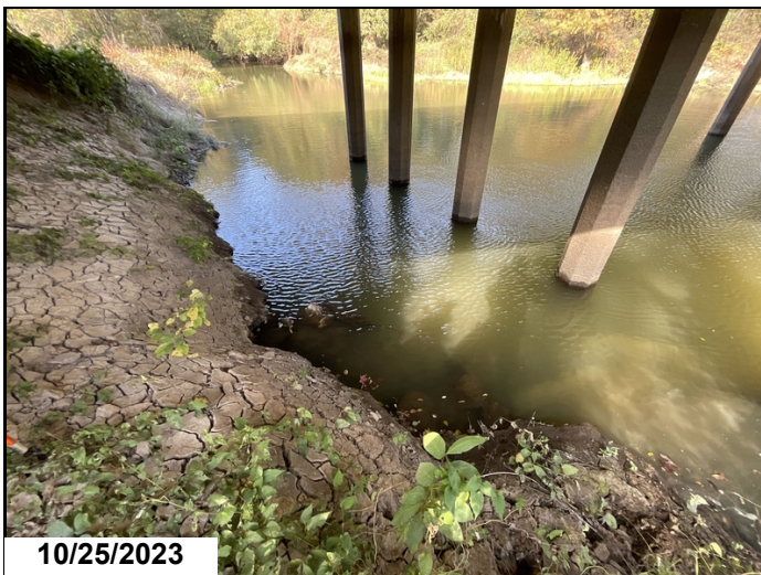
Scour hole at bent 2
