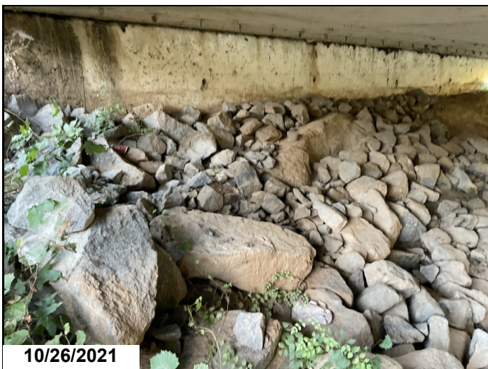
State forces have placed rip rap at bent 1.
