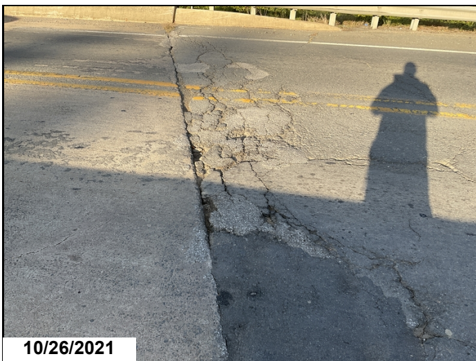
Potholes at bent 6
