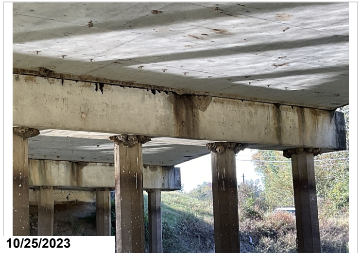
Bent 3 ahead face, spall with exposed rebar between pile 2&3 1'x2'x4"
