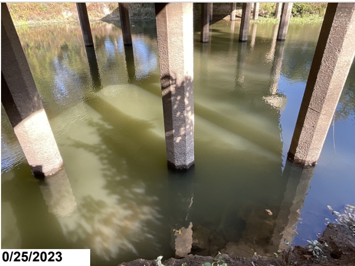
Abrasion to piles at bents 2,3 and 4
