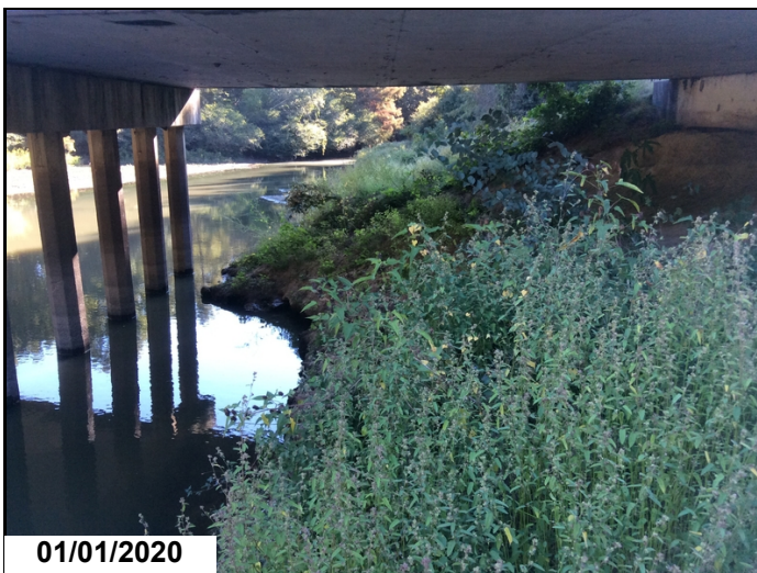
Under Span 1, there is a scour hole beginning to develop, causing the embankment to slide downward.
