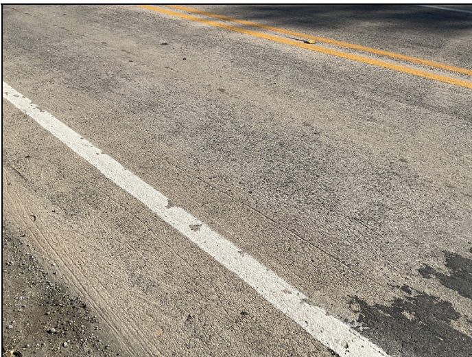
Sealable deck cracks
