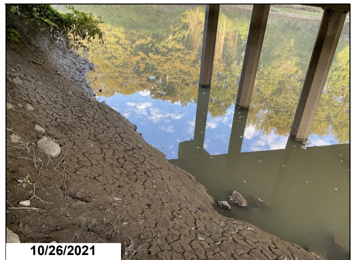
The embankment under span 1 has a scour hole beginning to develop, causing the embankment to slide.
