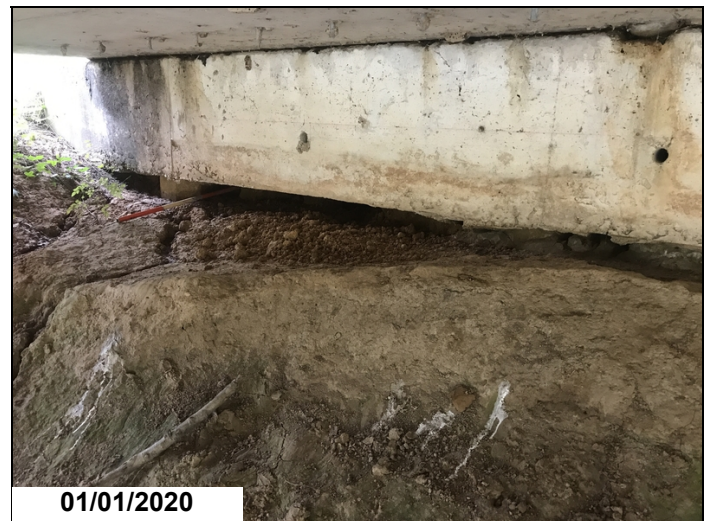
Bent 1: erosion action has undermined abutment exposing pile
