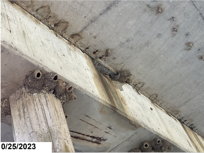
Bent 2 ahead side above pile 4 has a 1'x2'x7" deep spall with rebar exposed
