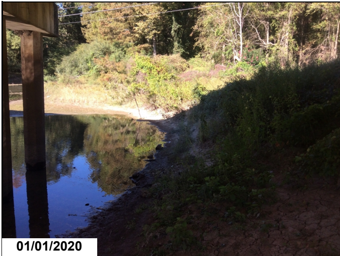
Near and under span 4 the stream bank is beginning to scour.
