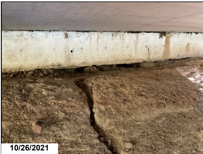
Erosion at Bent 4 has undermined the abutment and exposed two pile.
