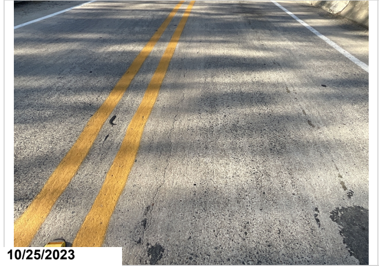
Longitudinal cracks center of bridge
