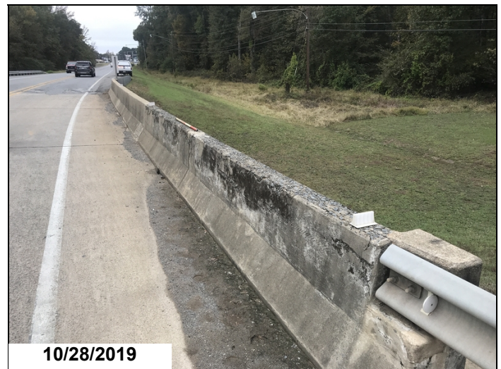
Span 3, Left concrete rail is deteriorating with aggregate losing bond.
