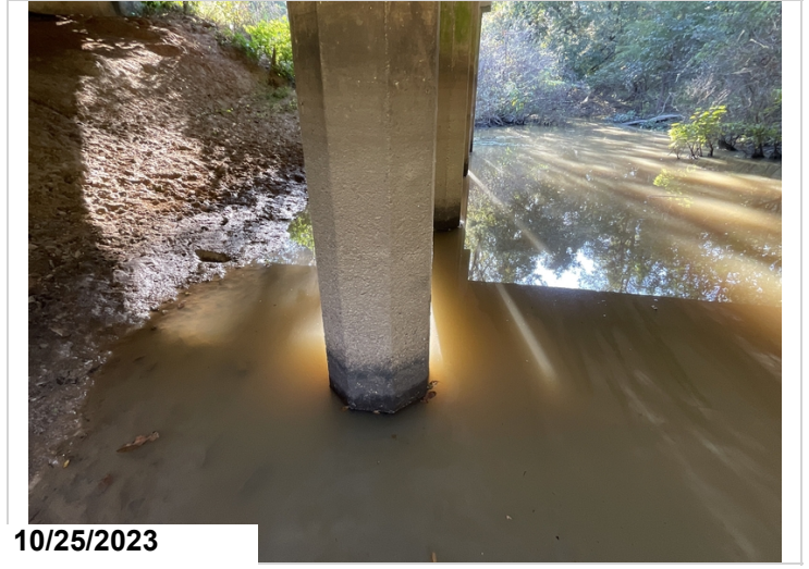
Abrasion to pile at bents 2 and 3
