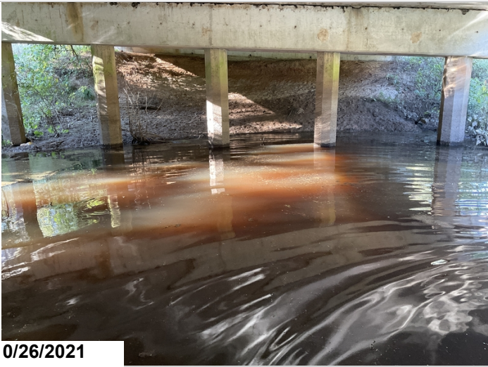
Bent 2 Abrasion on bottom of piles.
