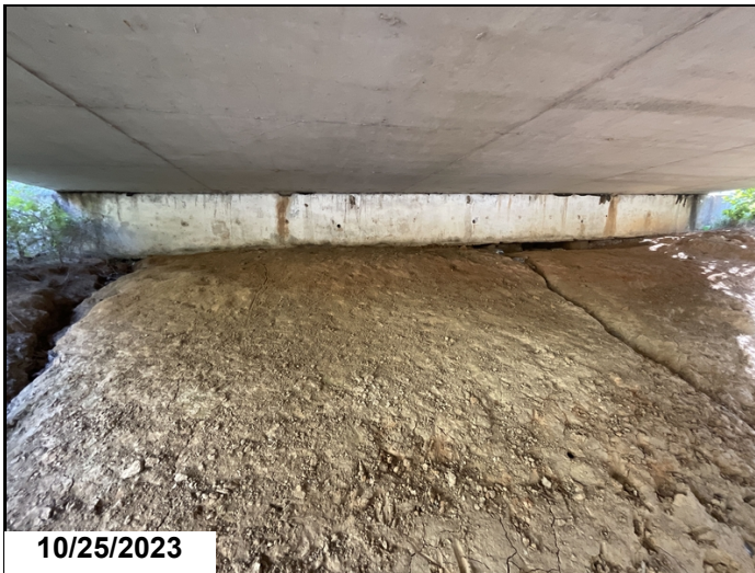
Bent 4 abutment erosion exposing two pile
