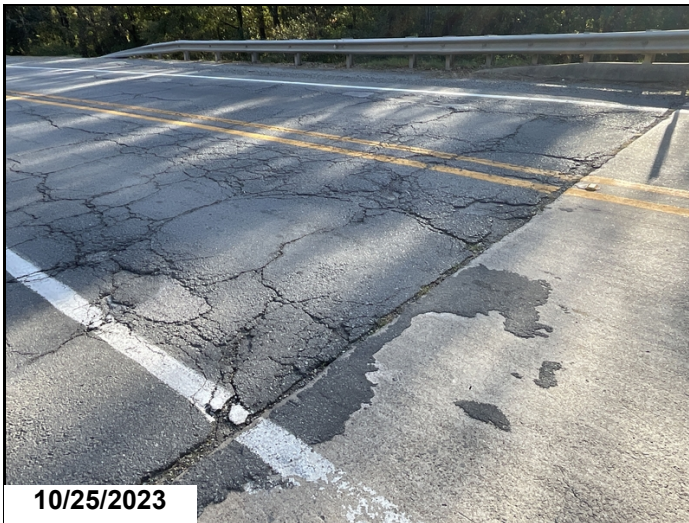
Bent 4 cracks and potholes in roadway
