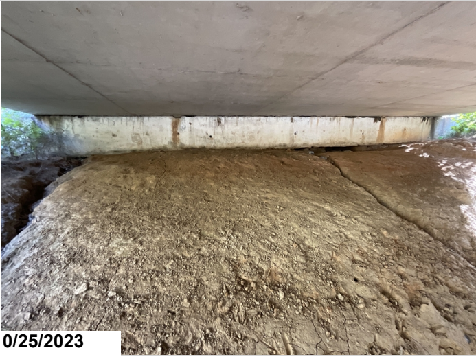
Bent 4 abutment erosion exposing two pile
