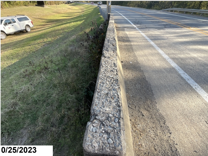
Scaling left bridge rail span 3
