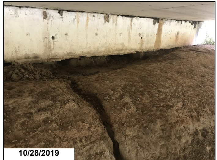
Bent 4: erosion action has undermined the abutment exposing 2 pile
