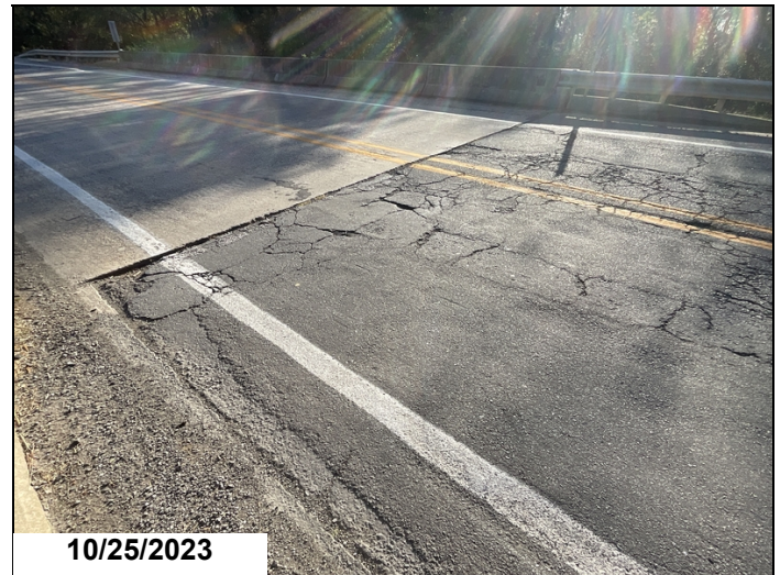
Bent 1 cracks and potholes in roadway
