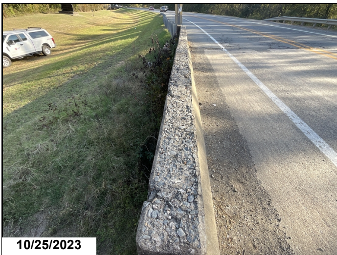
Scaling left bridge rail span 3
