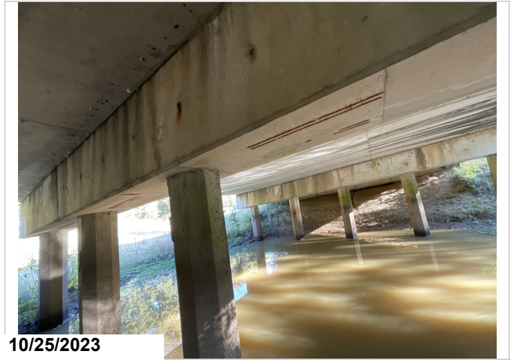
Bent 2 exposed wire
