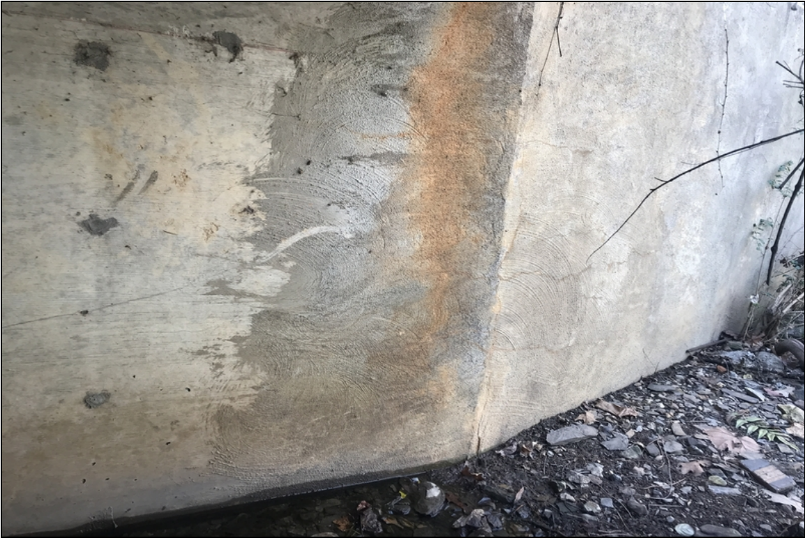
Barrel #1 Lt horizontal cracking at the wing wall juncture.
