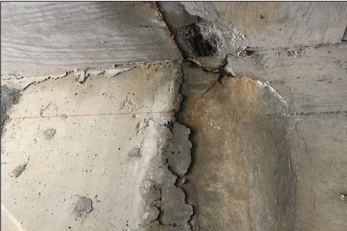
Barrel #1 Rt top slab spalling with exposed reinforcing steel.
