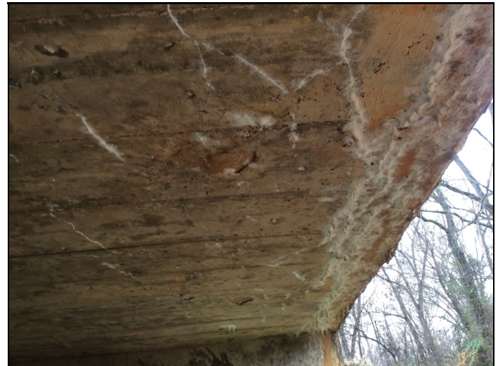
Barrel # 2 top slab cracking with efflorescence.
