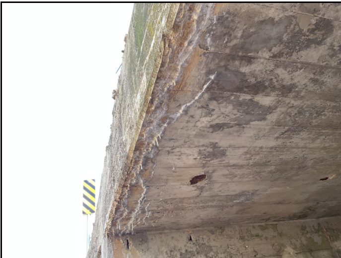
Barrel # 1 top slab, left side-Mapcracking with efflorescence.
