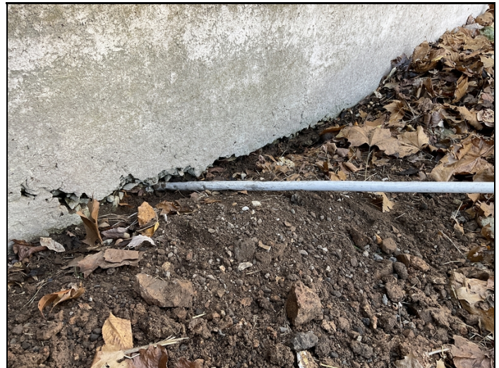
The base of the left wing wall at barrel # 1 has a 5' long area of concrete deterioration with up to 4" of concrete section loss.
