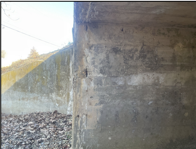
Wall # 2 Lt spalling with exposed reinforcing steel.
