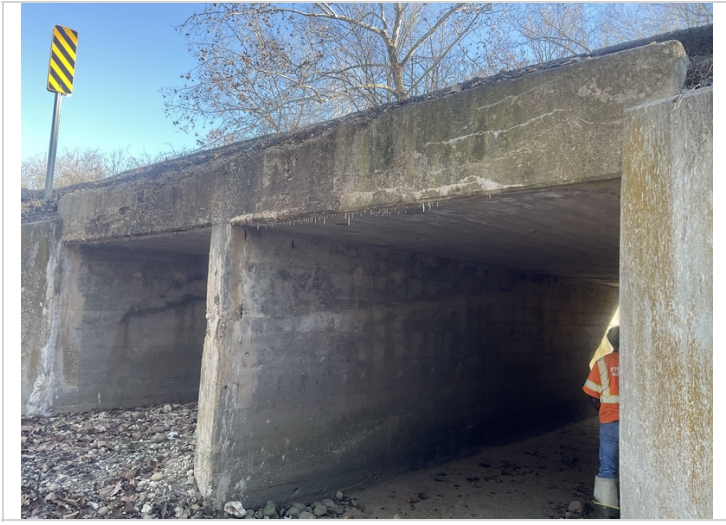
Left head wall concrete deterioration with efflorescence buildup.
