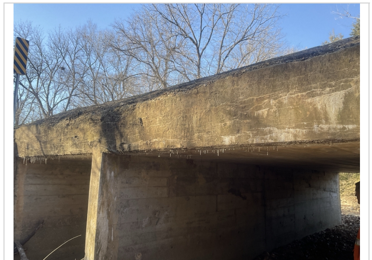
Right headwall concrete deterioration with efflorescence buildup.
