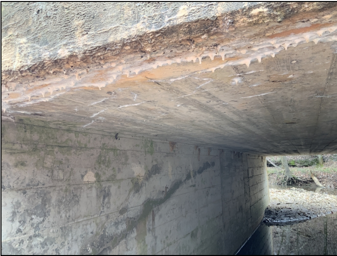
Barrel # 2 map cracking with efflorescence on the outlet side (typical for both barrels at the outlet and inlet sides)
