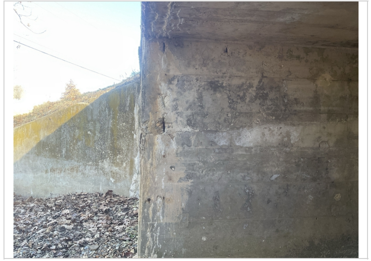
Wall # 2 Lt spalling with exposed reinforcing steel.
