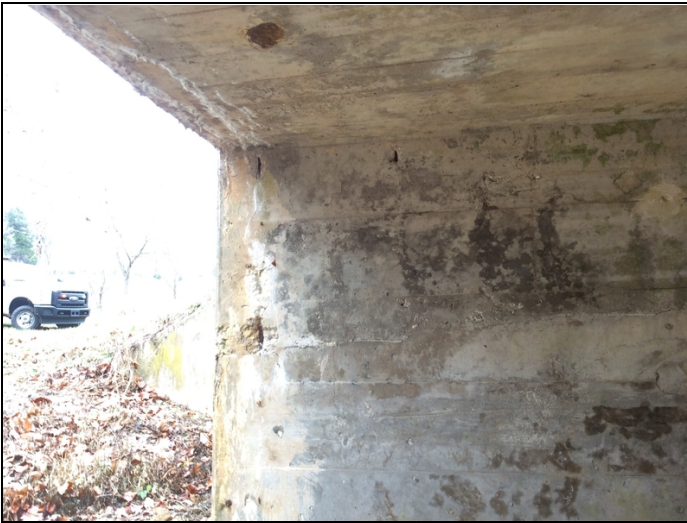
Spalling at the outlet end of the center wall that exposes reinforcing steel.
