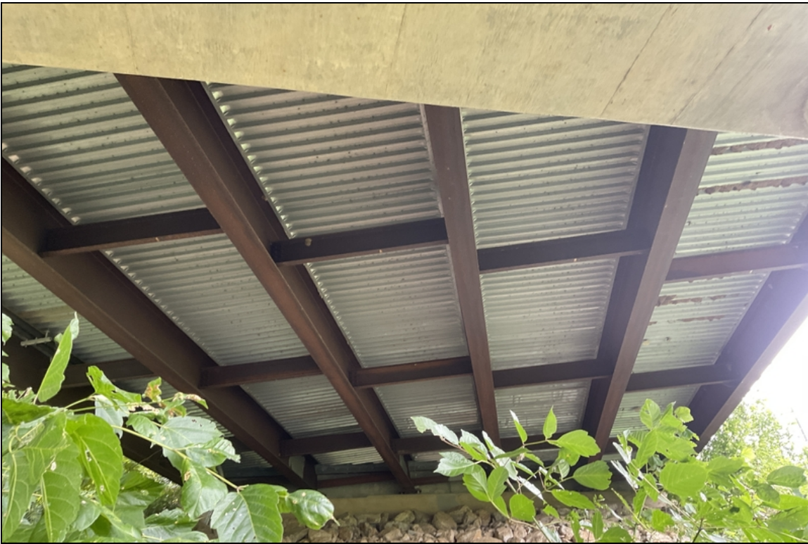
Span #1 typical undersurface of the deck.
