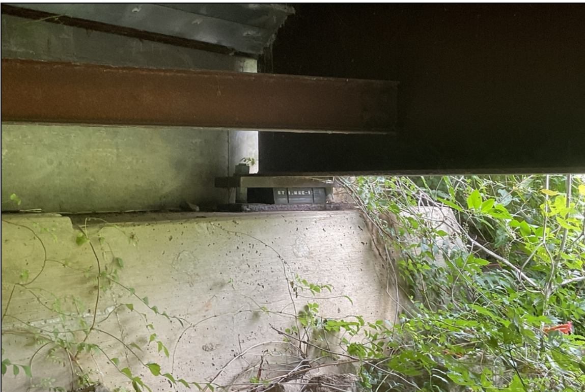
Abutment #1 bearing #1 active corrosion with pack rust.
