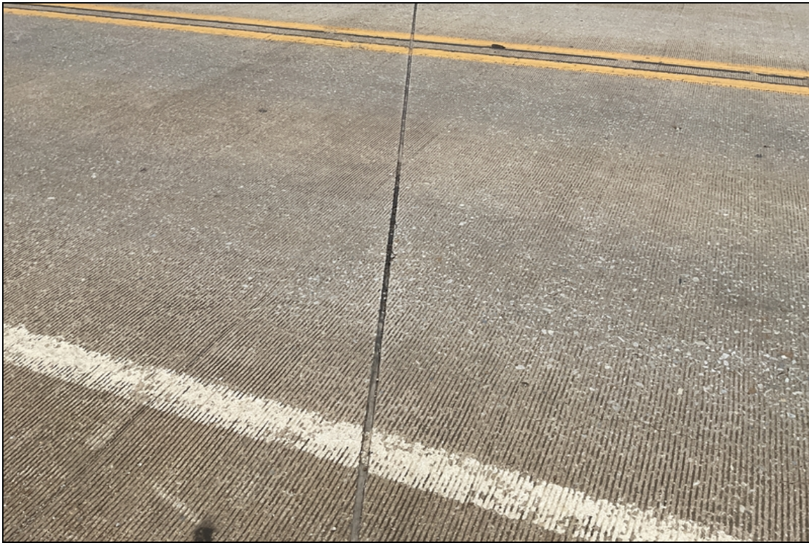
Deteriorating saw joint sealant.
