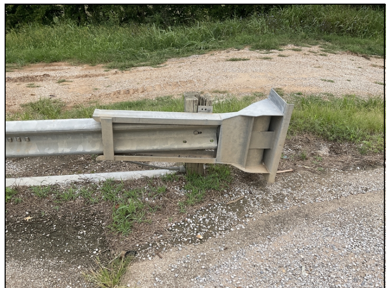
Northeast approach guardrail fractured post.
