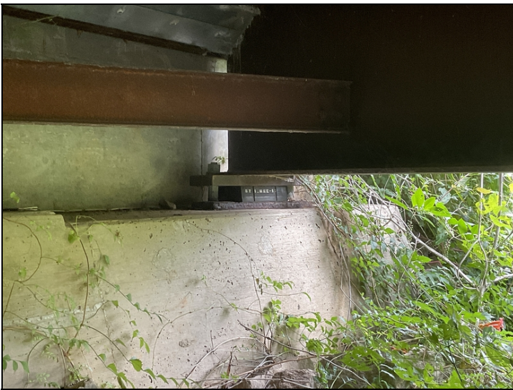
Abutment #1 bearing #1 active corrosion with pack rust.
