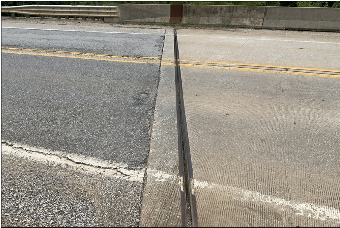
Abutment #2 strip seal.
