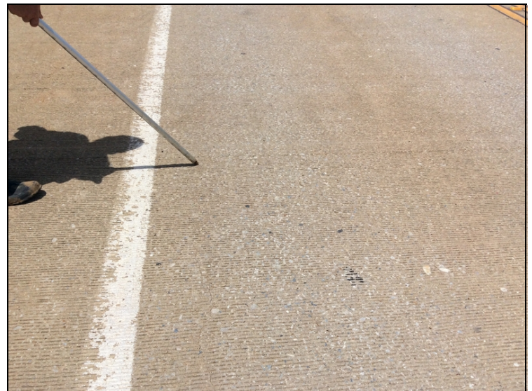
Longitudinal crack in the Right lane of Span # 4.
