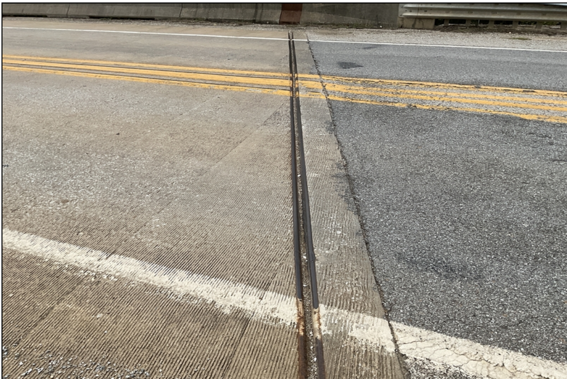
Abutment #1 strip seal.
