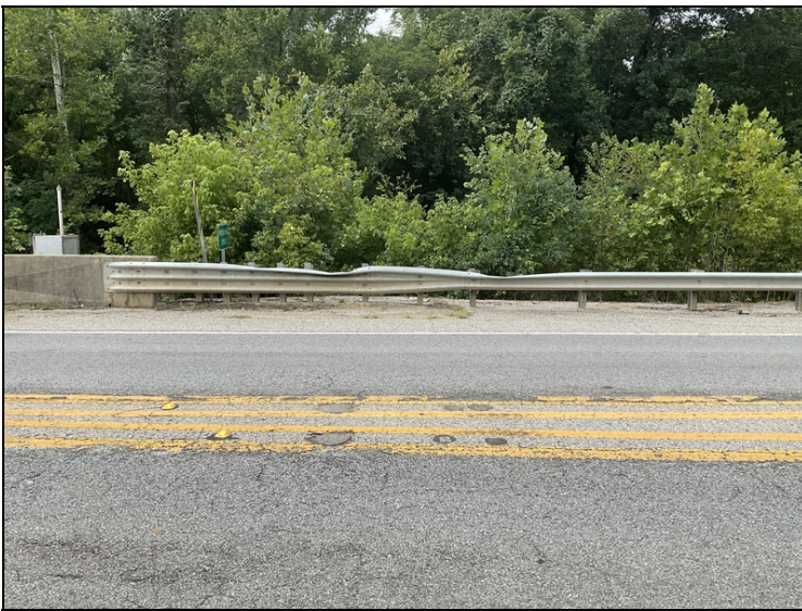
Southwest approach guardrail collision damage.
