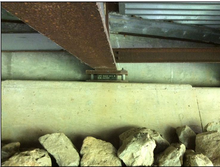
Bent # 1, Beam # 3. Missing anchor bolt nut.
