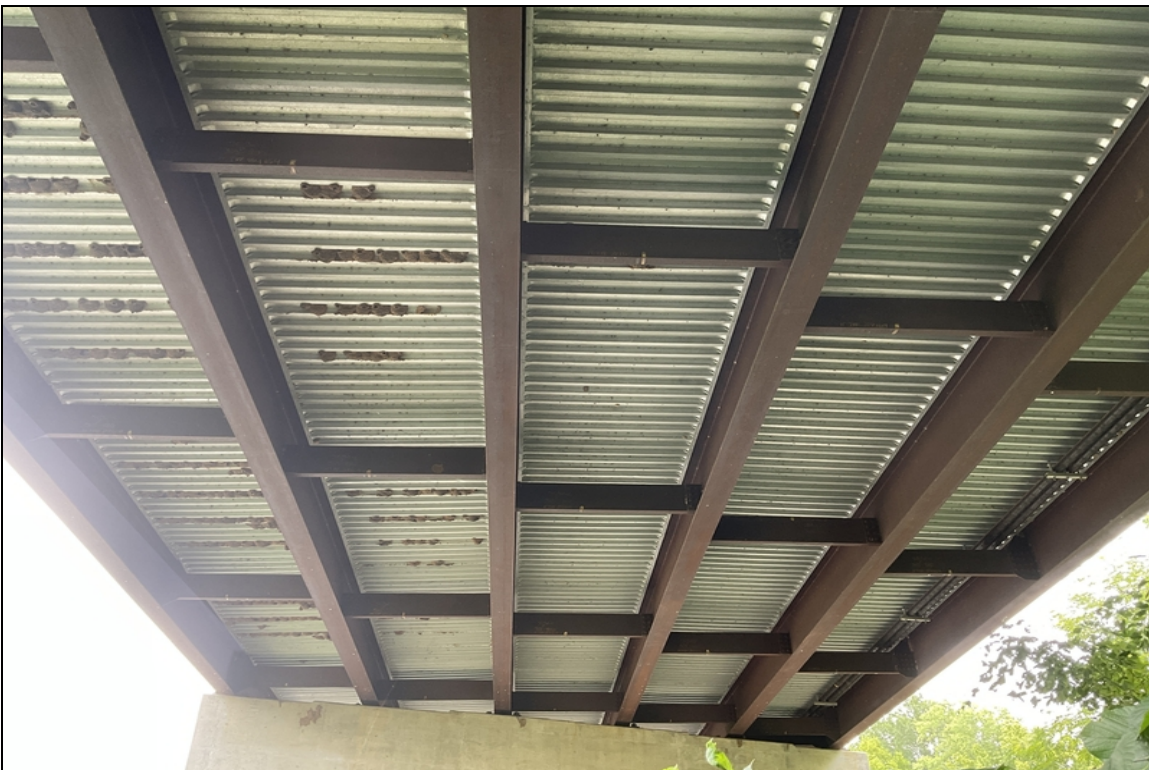
Span #2 Typical undersurface of the deck.
