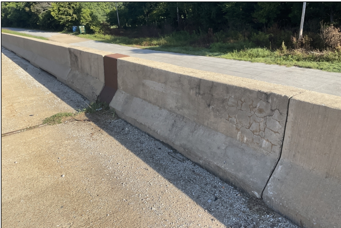
Bridge rail map cracking.
