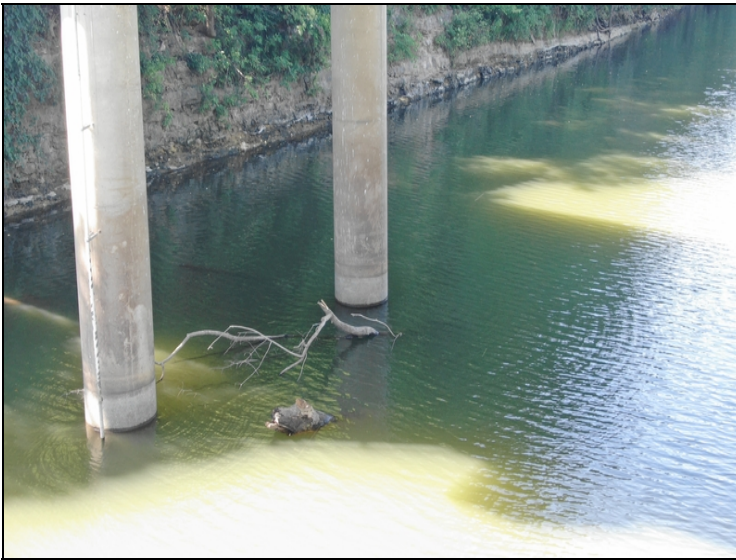
Drift and debris at bent 8.
