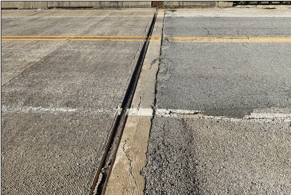
Abutment #1 wide cracking in the top of the backwall.
