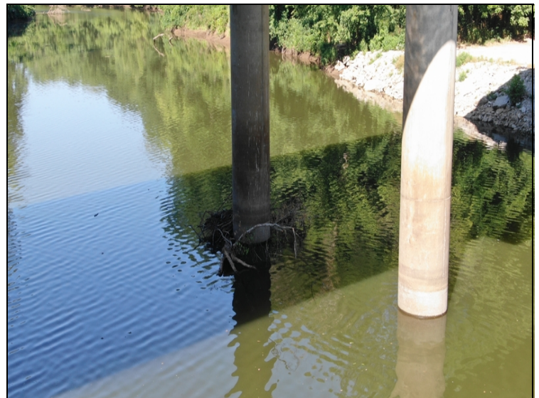
Drift and debris at bent 7.
