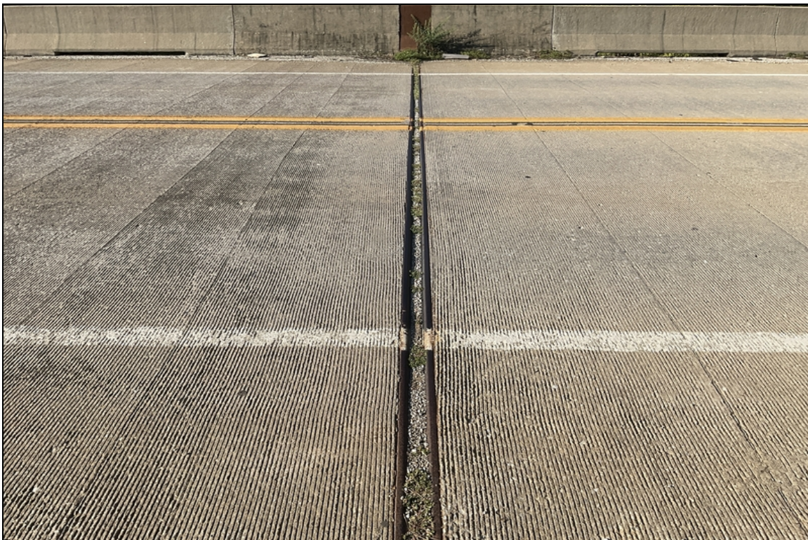
Bent #6 strip seal expansion joint.
