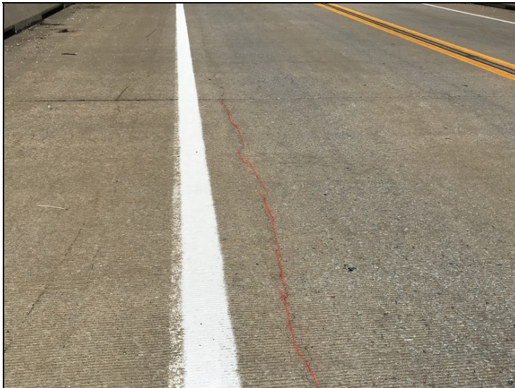
Span 7, right lane-Longitudinal cracking.
