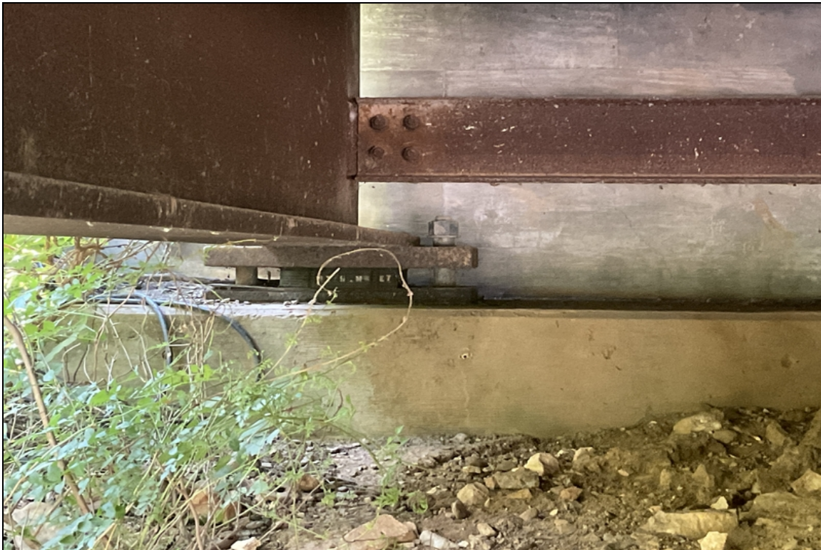
Abutment #2 exterior bearings with active corrosion and pack rust.
