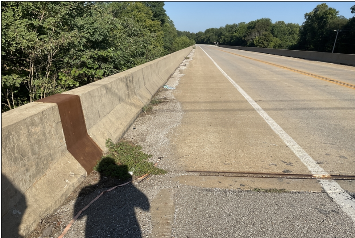
Debris accumulation in the gutters.
