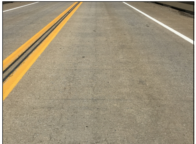
Span 6, left lane longitudinal cracking.
