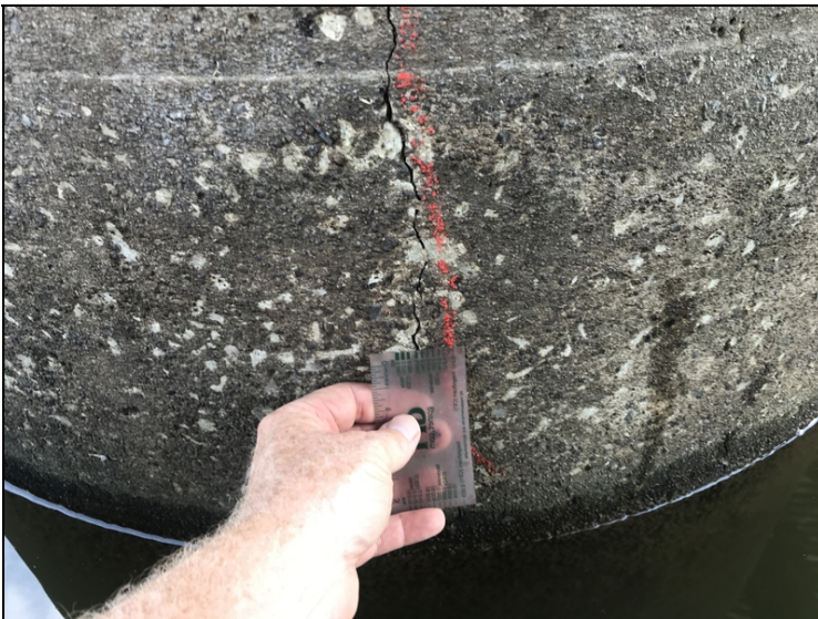
Bent 7, left column-Vertical cracking.
