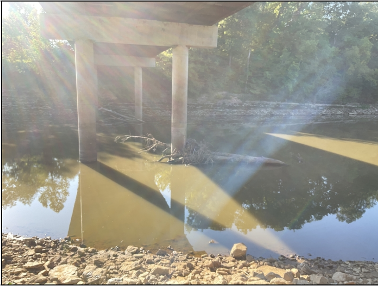
Bent # 7 & 8 drift accumulation.
