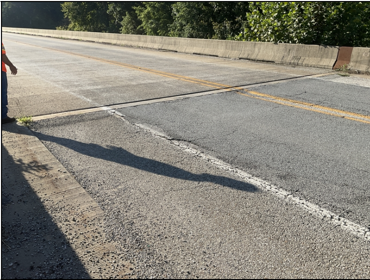
West approach roadway asphalt settlement at abutment #1.
