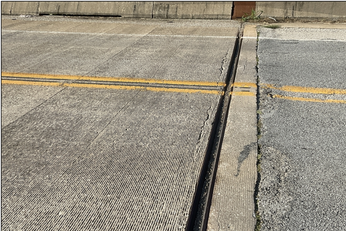
Span #1 wide cracking adjacent to the strip seal expansion joint.
