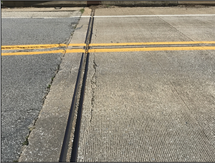
Span 1-Transverse cracking / spalling adjacent to abutment # 1 expansion joint assembly.
