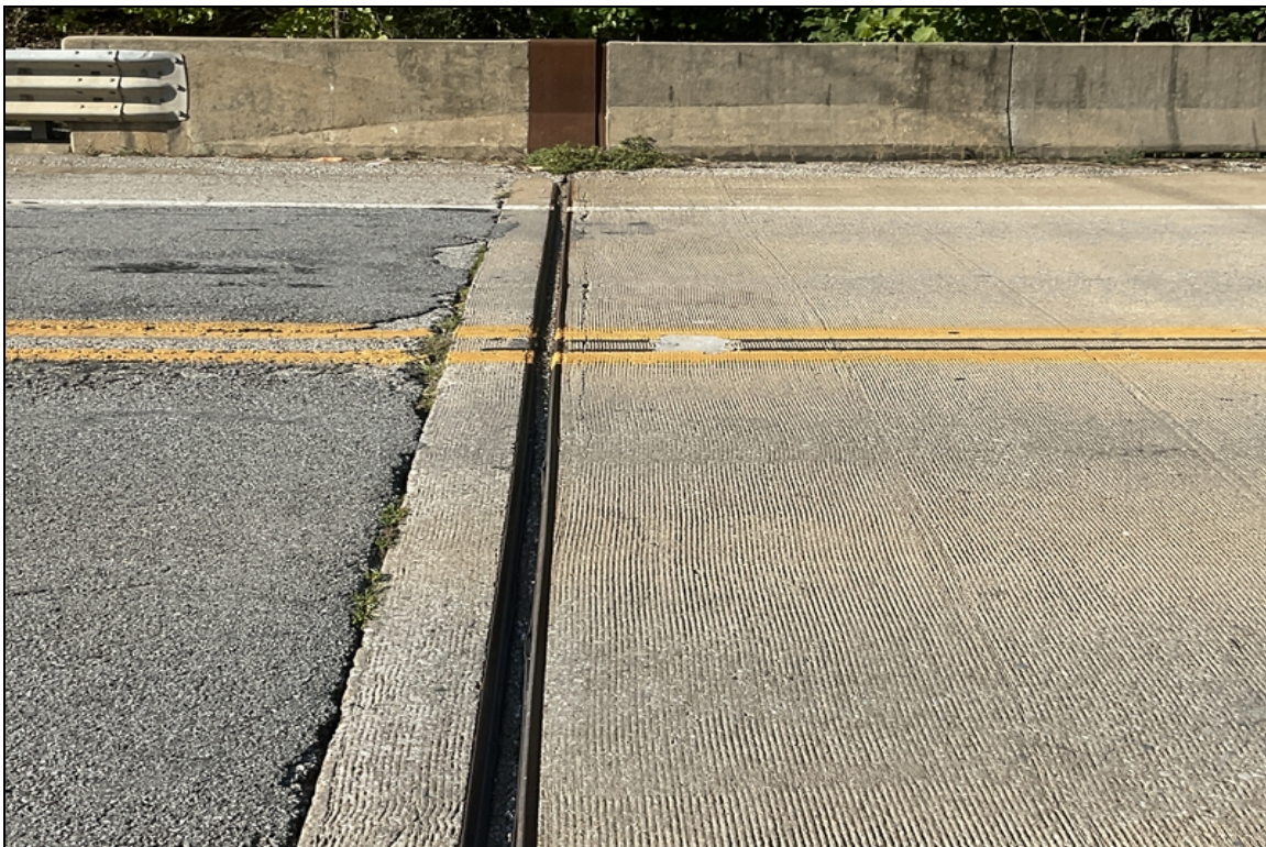
Span #8 cracking adjacent to the strip seal expansion.
