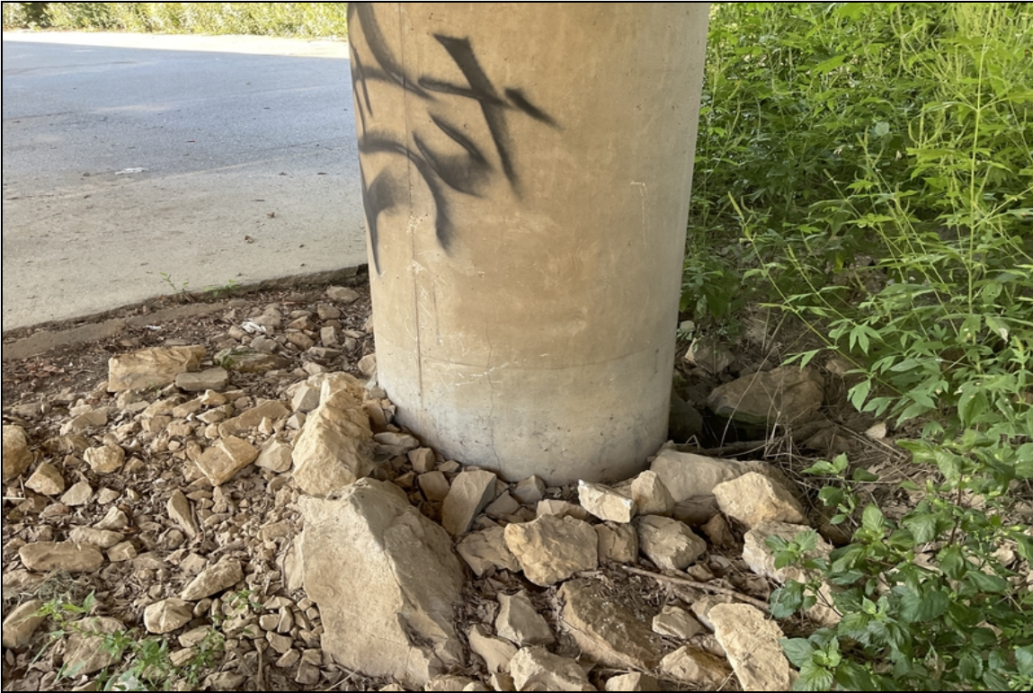
Bent #2 column #2 vertical cracking.
