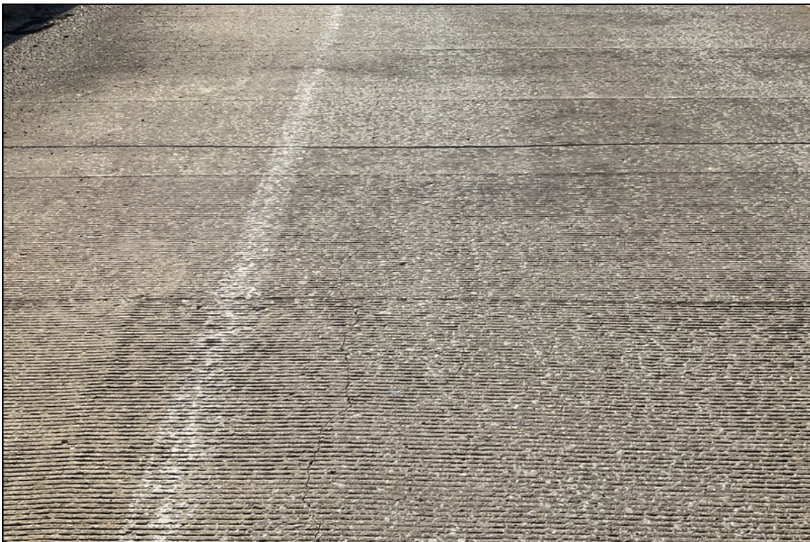
Sealable deck cracking.
