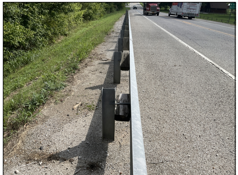
Northeast approach guardrail with fractured wood spacer blocks.
