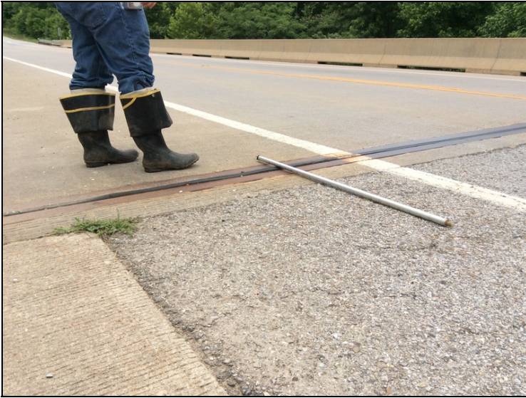
Expansion joint seal. Right side of Bent # 5.
