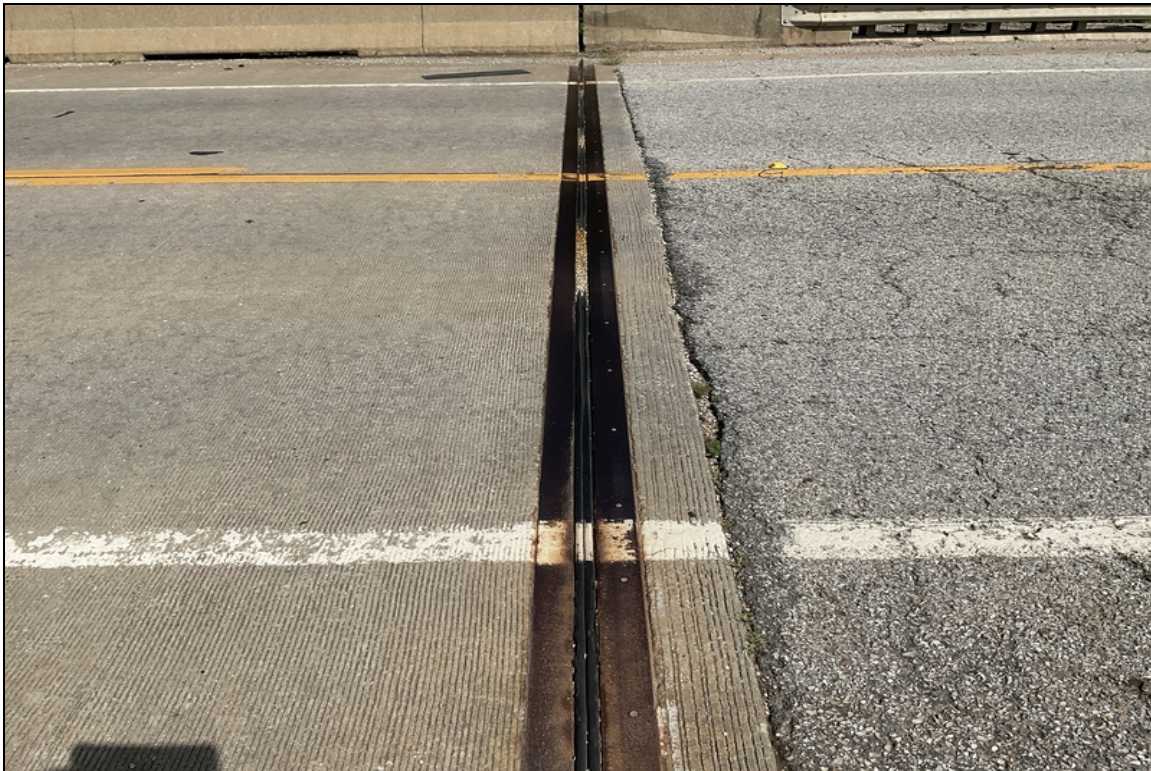
Abutment #2 compression joint seal.
