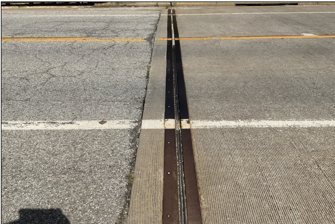
Abutment #1 compression joint seal.
