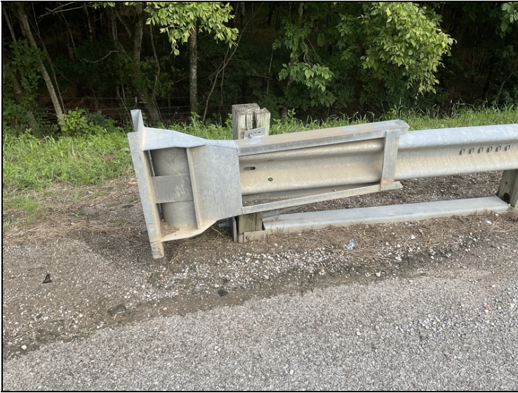
Northwest approach guardrail collision with a damaged post.
