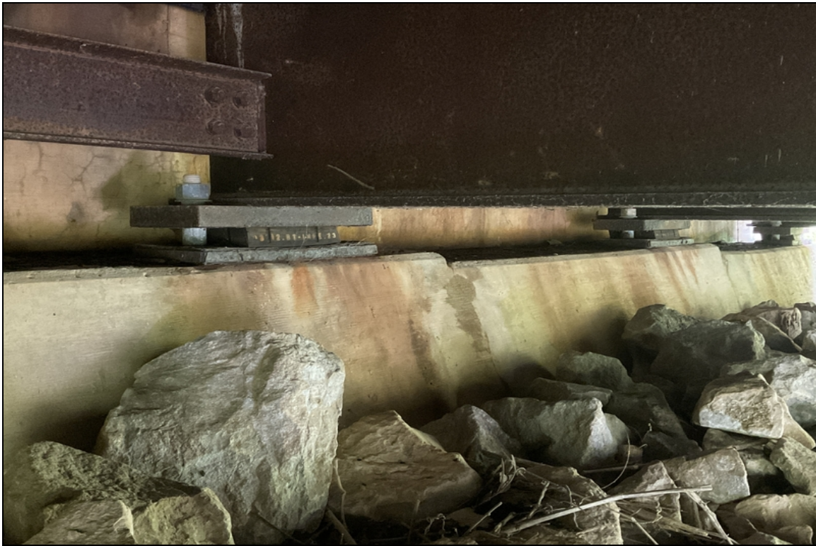
Abutment #1 typical elastomeric bearings.
