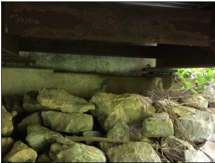
Right side of Bent # 5. Leaking expansion joint seal.
