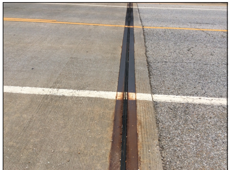
Bent # 5 expansion joint.
