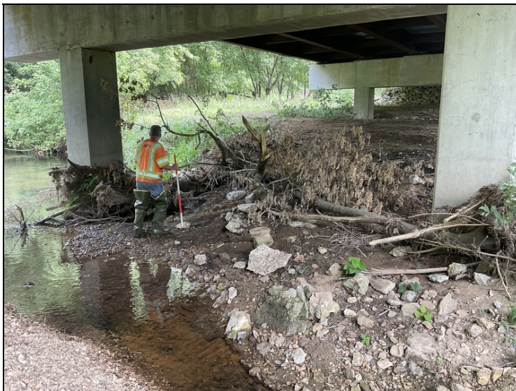
Bent #3 drift accumulation.
