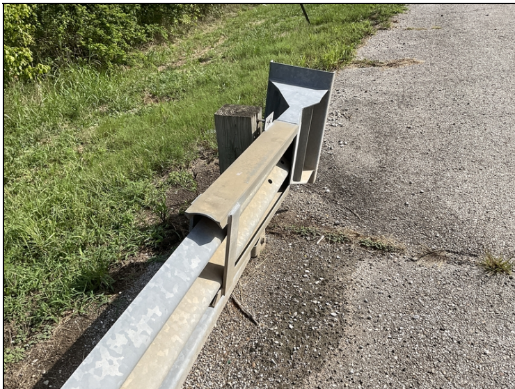
Northeast approach guardrail end terminal.
