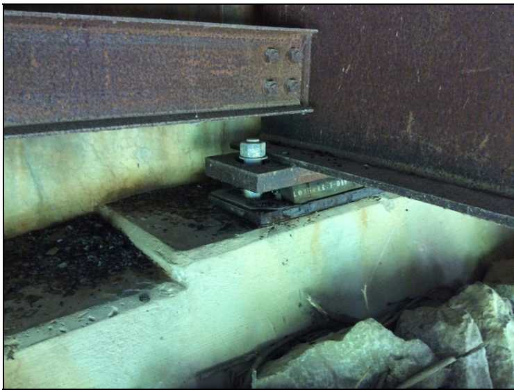
Bent # 1. Beam # 5. Active corrosion in the masonry plate.
