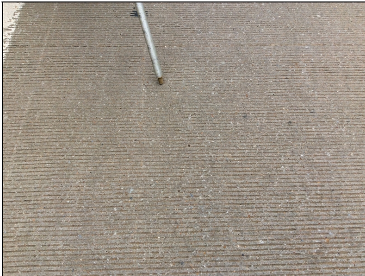
Deck. Sealable longitudinal crack.
