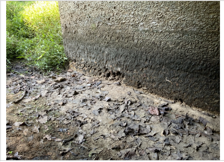
Moderate abrasion at bottom of divider wall.
