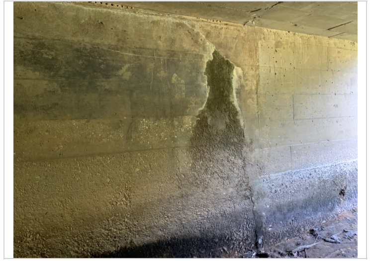
Barrel 2 cracks
