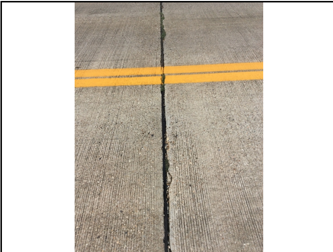
Joint - Bent 2 : Loss of adhesion
