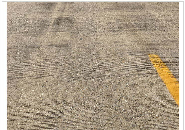
Deck cracking span 1 left.
