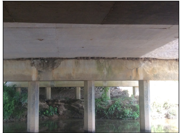
Bent 3 ahead spall with exposed rebar and delamination.
