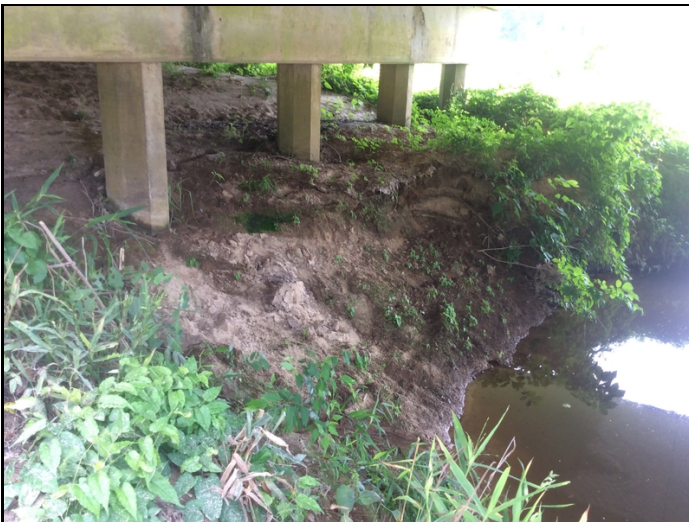
Bent 2 endslope erosion.
