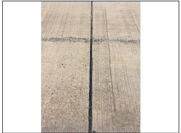
Joint - Bent 3: Loss of adhesion
