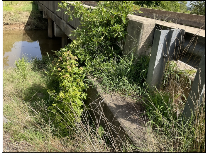
Trees, vines and vegetation tree growing at Bent 5 right side of abutment.
