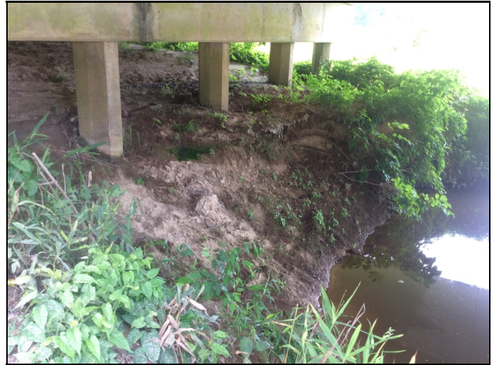
Endslope - Bent 2: Erosion / Scouring
