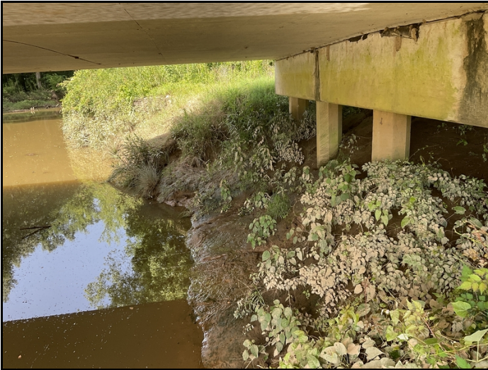
Bent 2 endslope erosion.
