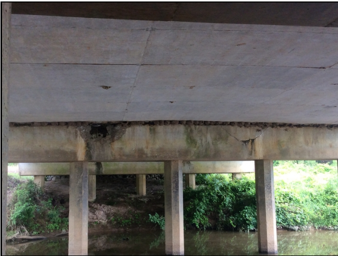
Cap - Bent 3 : Spalls and delaminations
