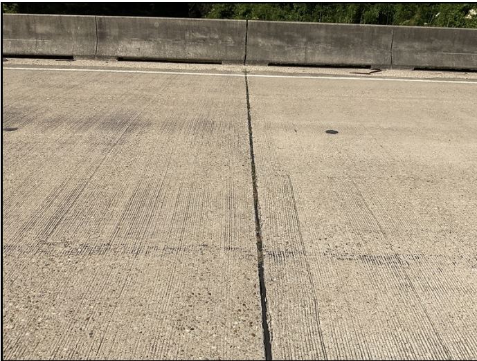
Bent 3 joint seals have loss of adhesion.
