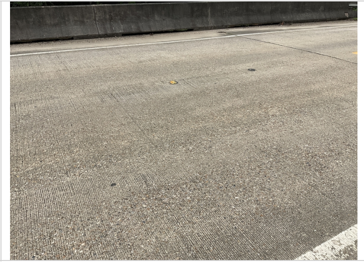
Deck - Span 2: Abrasive wear
