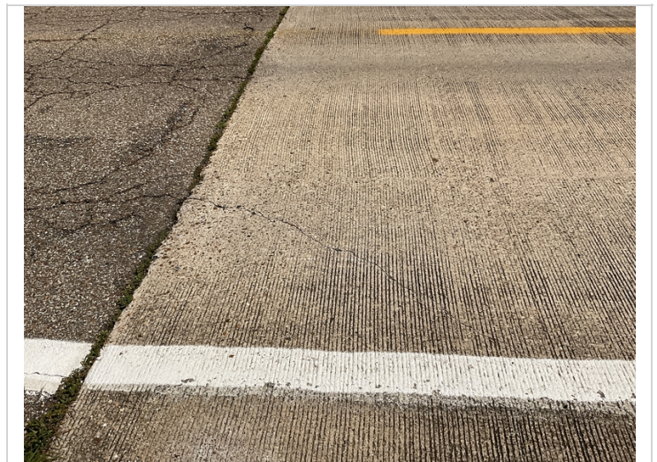
Span 1 right Shear cracking on corner of deck. And cracking has efflorescence on under side of deck same area.
