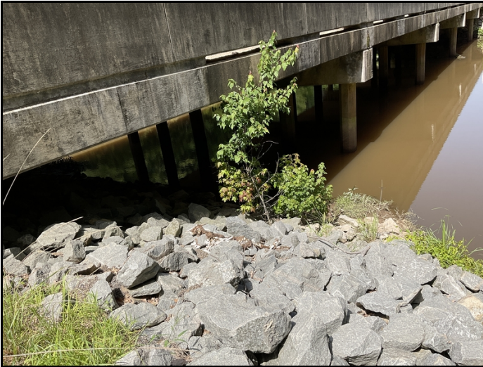
Span 5 left tree growing onto soffit of deck.
