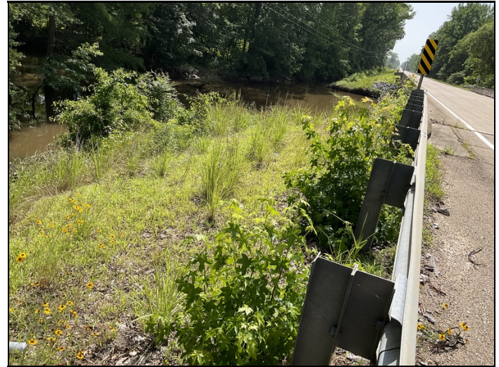
Trees, vines and vegetation on approach under railing and endslopes.
