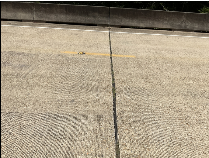
Bent 4 joint seals have loss of adhesion.
