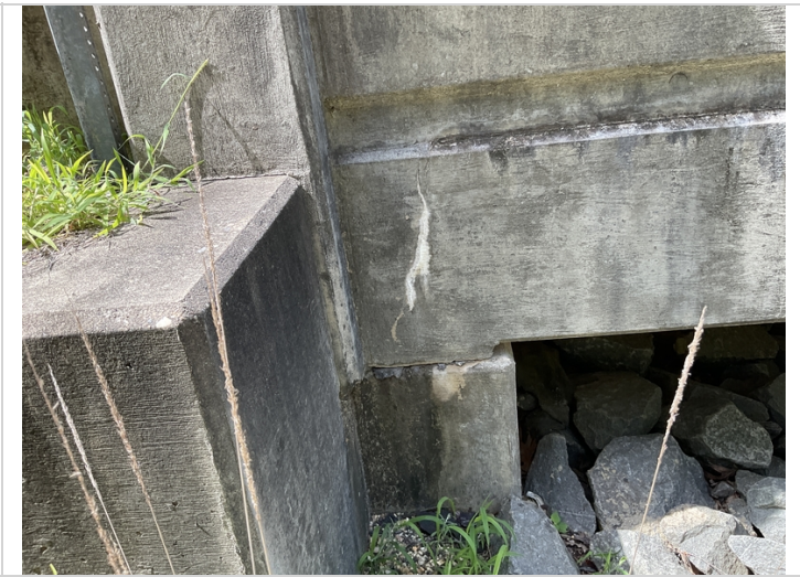
Bent. 6 Shear crack with efflorescence. Common most bents at ends of deck.
