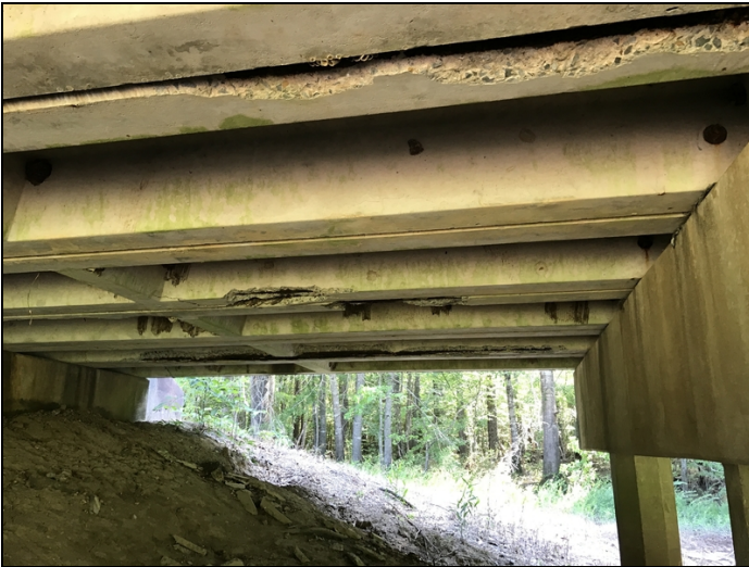
Span 1 units 2,3,4,5,& 7, girder have spalls with exposed rebar.
