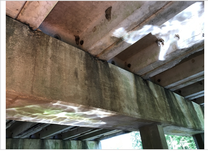
Bt. 6, back side, spalls below girders.
