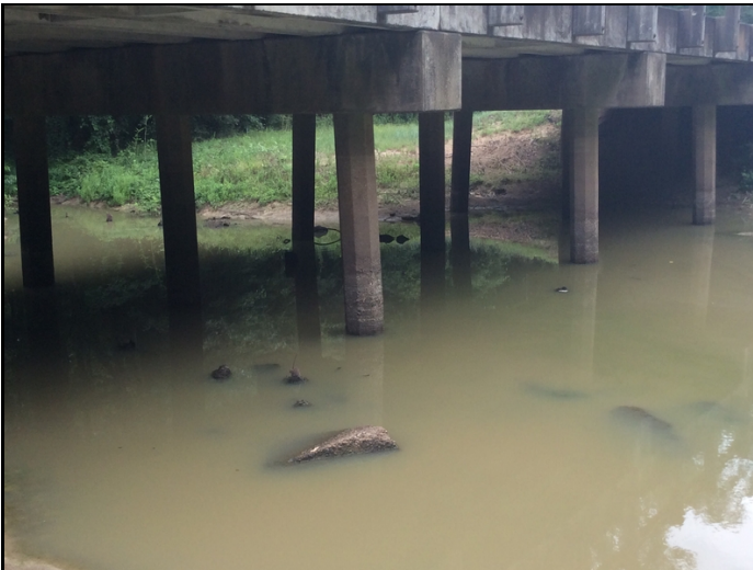
Abrasion and wear on piles
