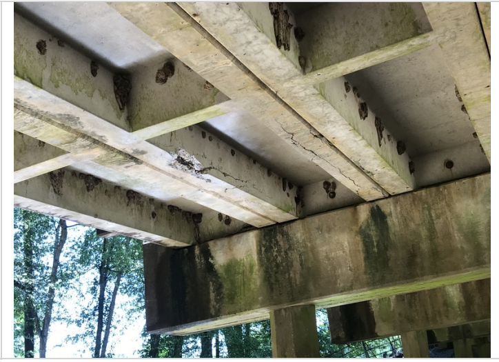
Span 2 unit 2, cracked and spalled with exposed rebar
