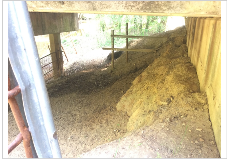
Abutment 2 slope has eroded and cattle are using this to get back & forth from one side of the road to the other & have beaten the abutment slope down at the abutment.
