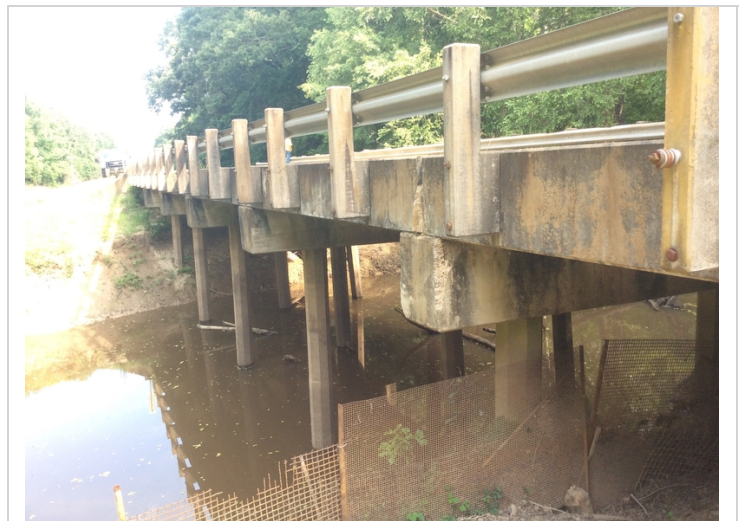
Bent 6 cap has spall on both ahead & back corners of Rt. End of the cap. Also grout between spans 5 & 6 on Rt. end is coming out.
