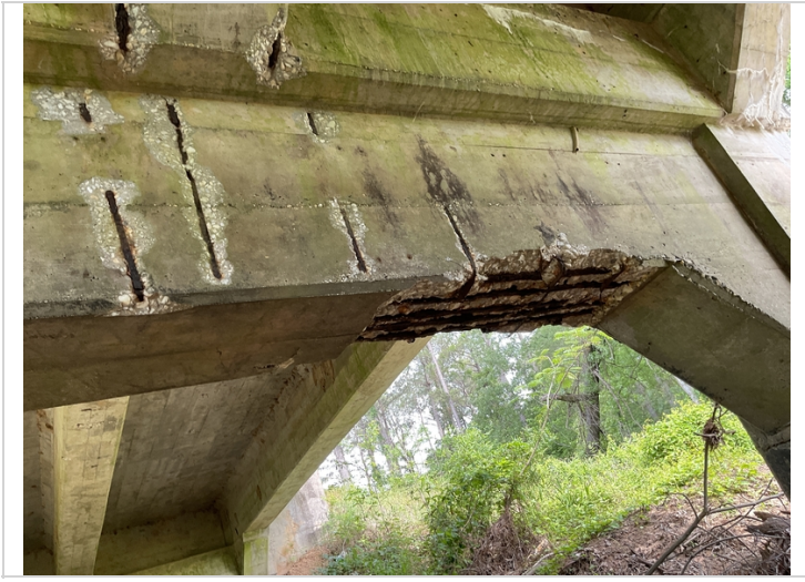
Bent 2 pier wall, exposed rebar
