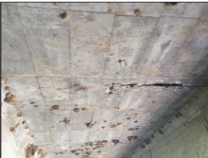
Span 1, mid-span between girders 2 & 3 there is a spall on Soffit of deck with exposed steel with section loss.
