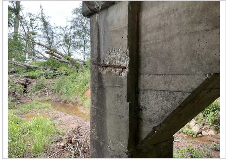
Column 2 exposed rebar
