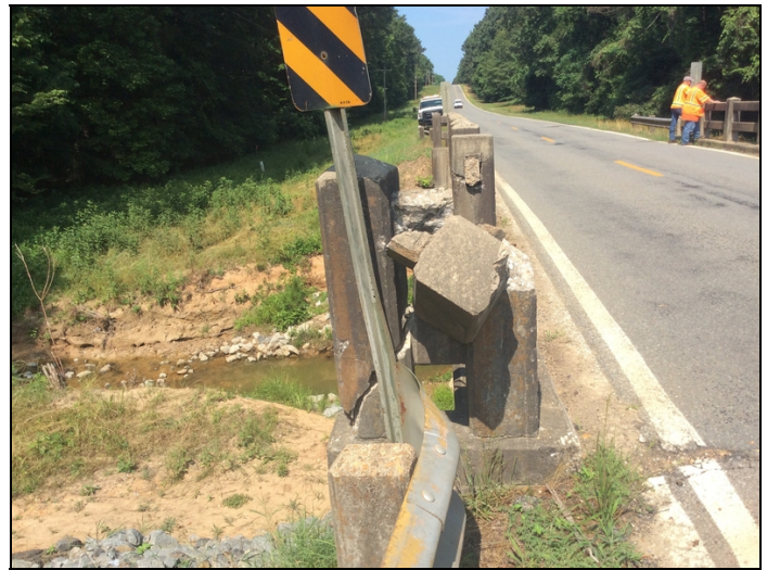
Abutment 2 Rt. BR end post & top rail in last section before the BR end post, has collision damage.
