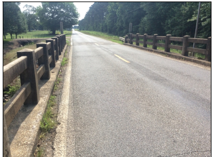
Abutment 2 Rt. BR end post & top rail in last section before the BR end post, has collision damage.
