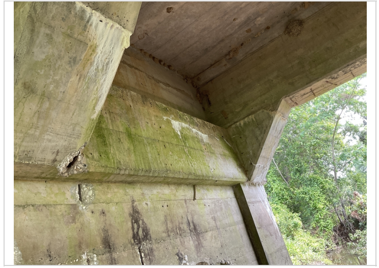
Bent 2 efflorescence in cap
