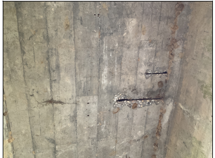
Span 2 bay 2, exposed rebar in soffit
