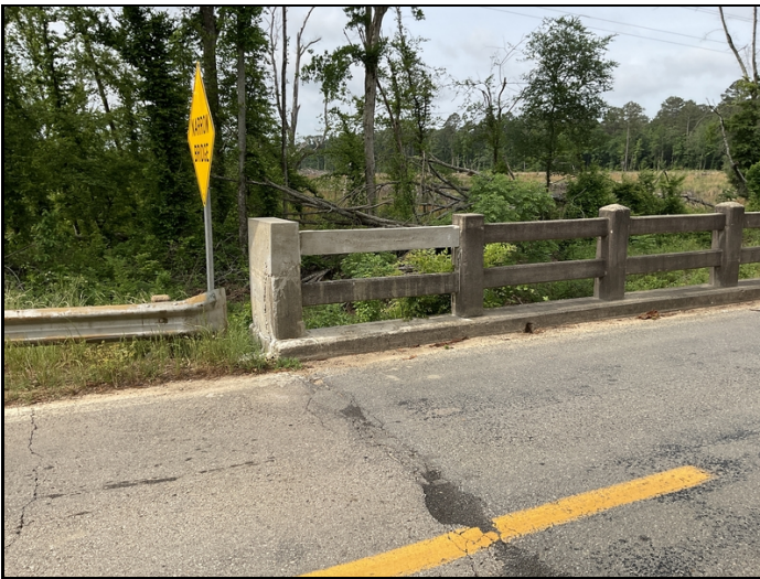
Repaired bridge railing.
