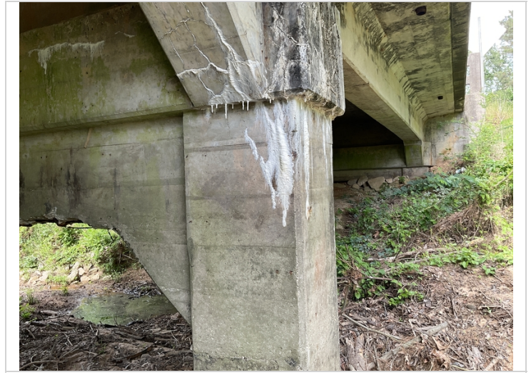
Bent 2 column 1, build up of efflorescence
