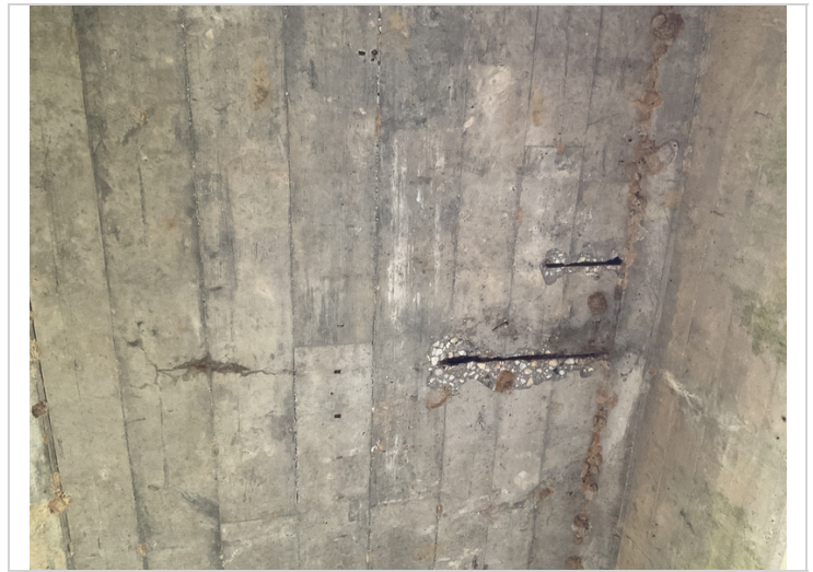
Span 2 bay 2, exposed rebar in soffit
