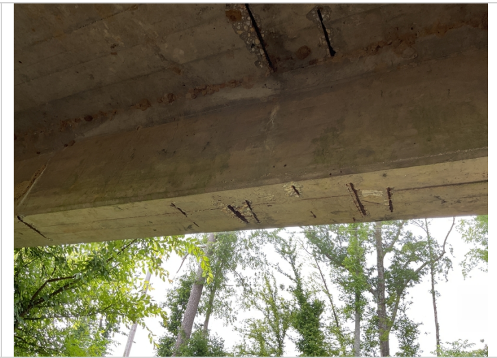
Span 2 girde 3, exposed rebar
