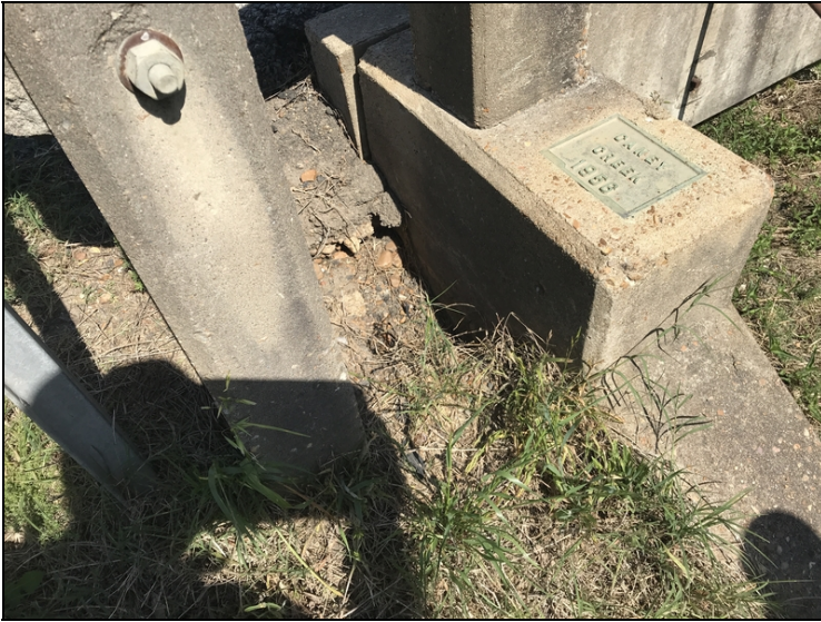
Erosion at abutment #2 left side.
