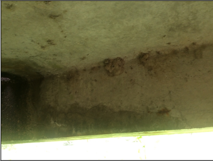
Span #2 unit #1 left and right leg cracked with efflorescence last half of span.
