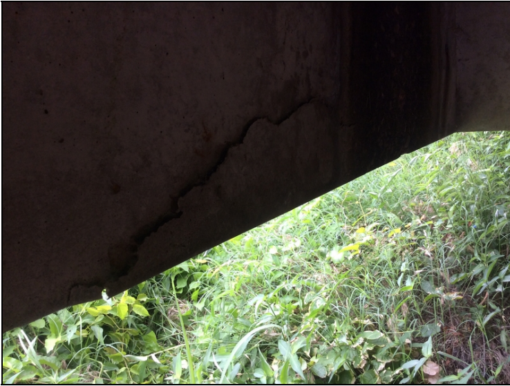
Span #4 unit #1 left leg 2' delamination.
