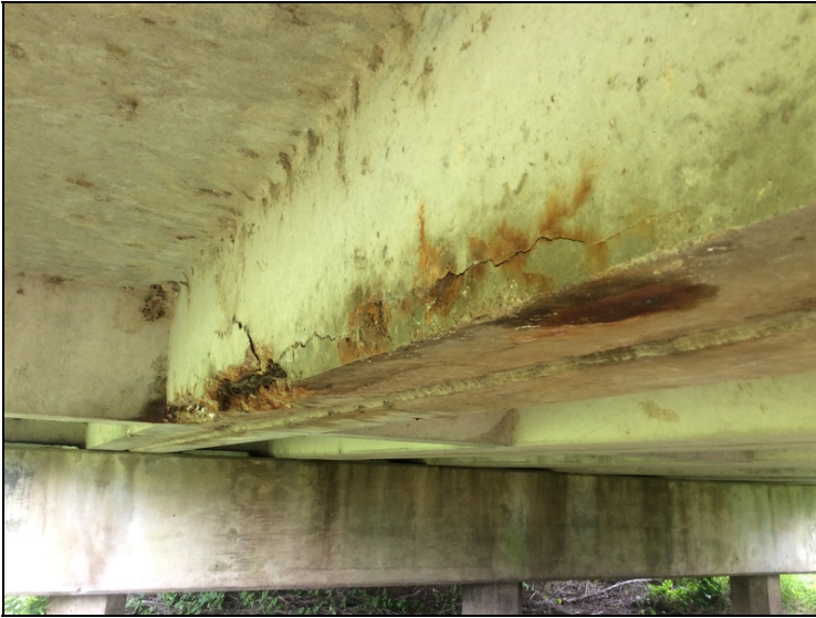
Span #2 girder #7 left leg mid span 4' spall with exposed rebar large section loss. Remaining section of last half of span left leg cracked with rust stains.
