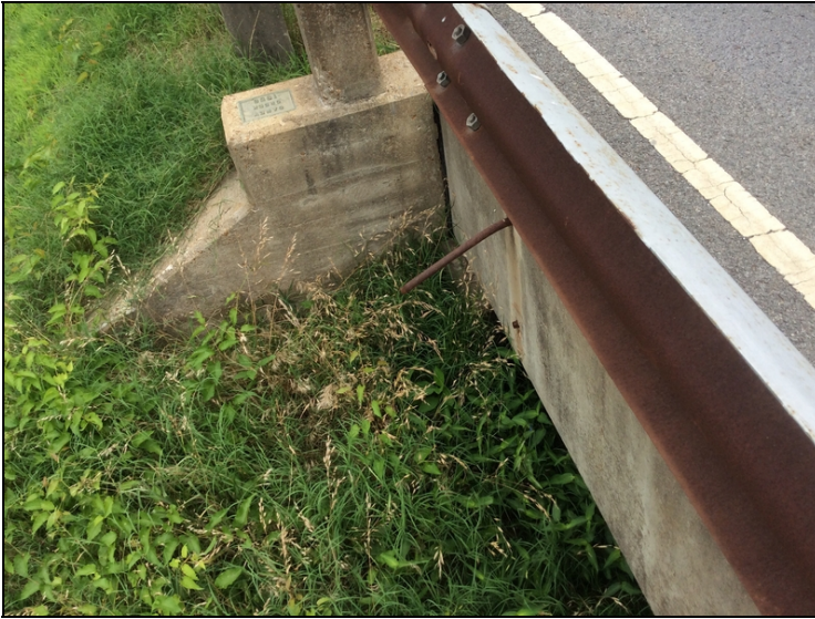
Span #3 left side next to last post gone.
