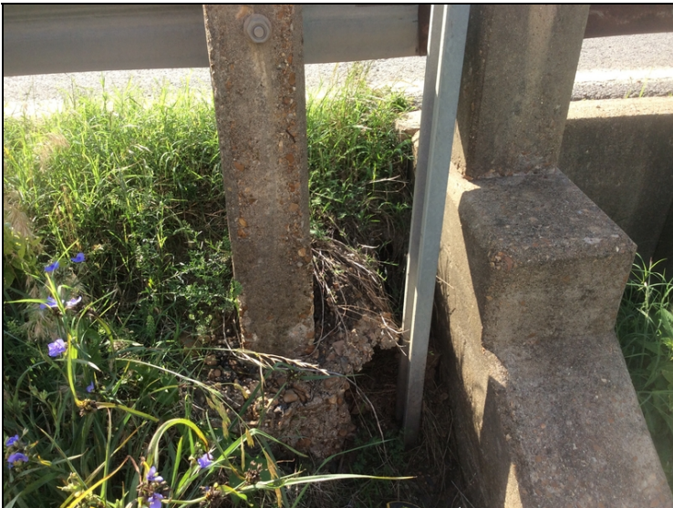
Abutment #1 right shoulder at bridge is eroded one foot deep behind head wall.
