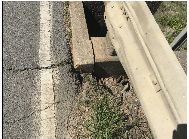
Erosion at abutment #1 right side.
