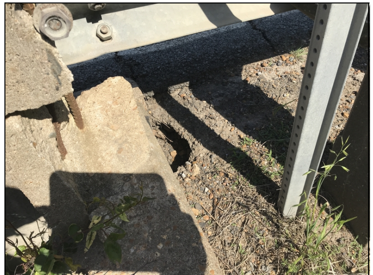
Minor erosion at abutment #1 left side.
