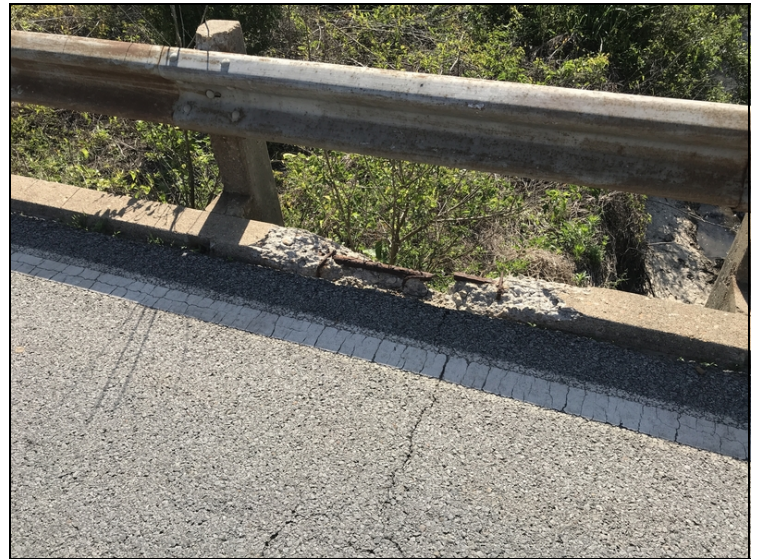
Left curb spalled at bent #3.
