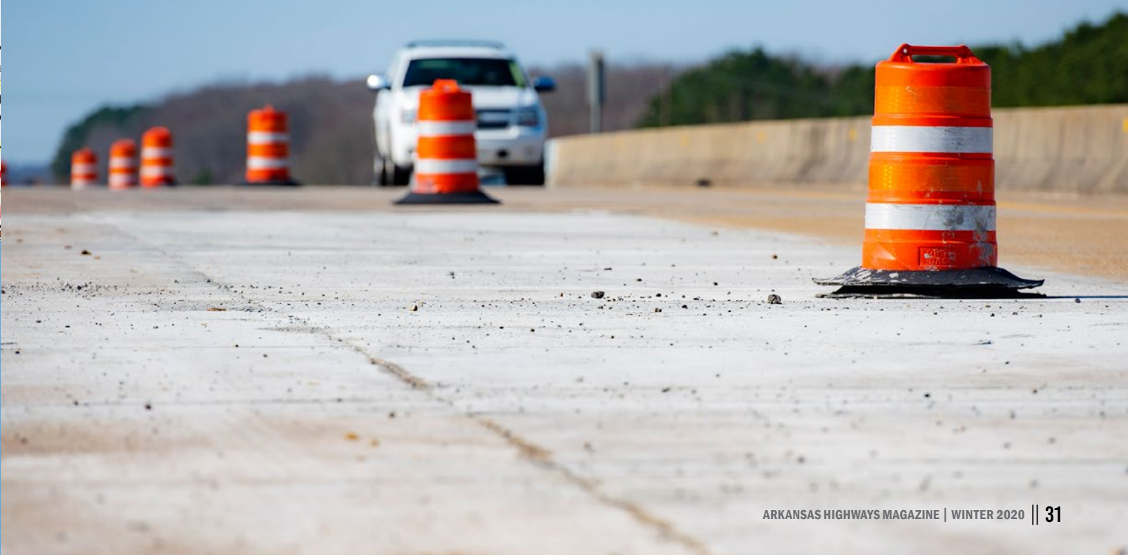
Improvements under way on U.S. Highway 67
