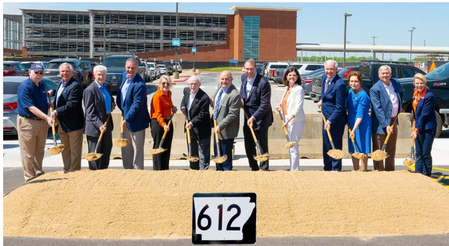
In April, ARDOT officially broke ground on a new XNA Connector Road and a new section of the Springdale Northern Bypass.
