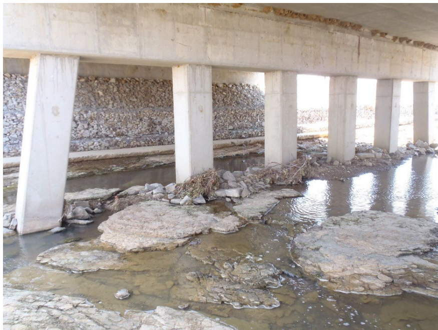
Figure 2. Good example of drift that does not need any maintenance need associated. Document in the channel notes.
