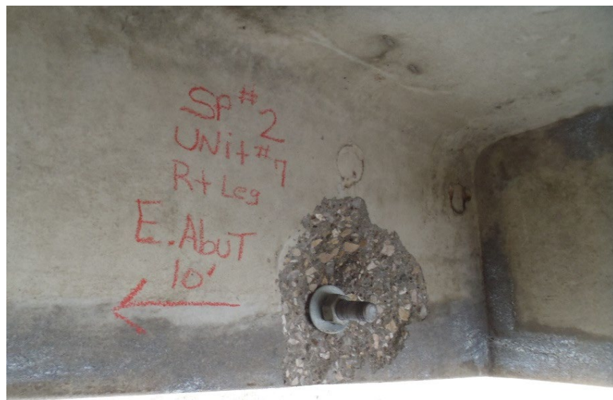
Figure 3. Good example of minor exposed steel in RCBC that does not need a maintenance need.
