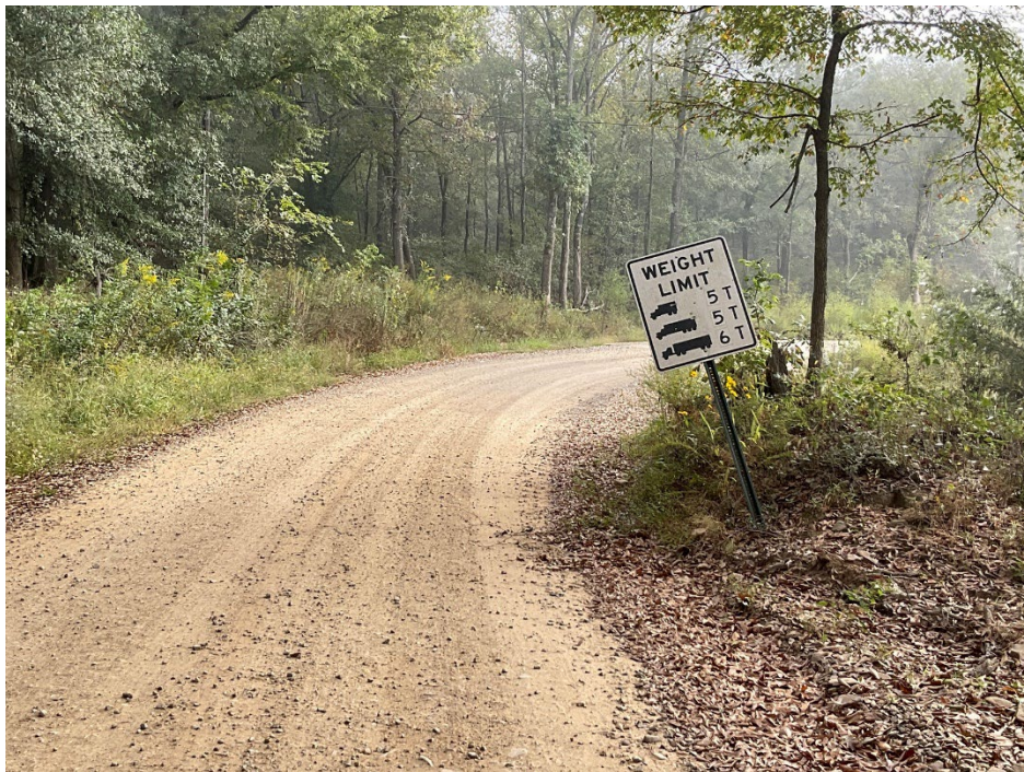
Figure 47. A leaning posting sign that is stable – should not be a maintenance need as long as it still conveys message to traveling public
