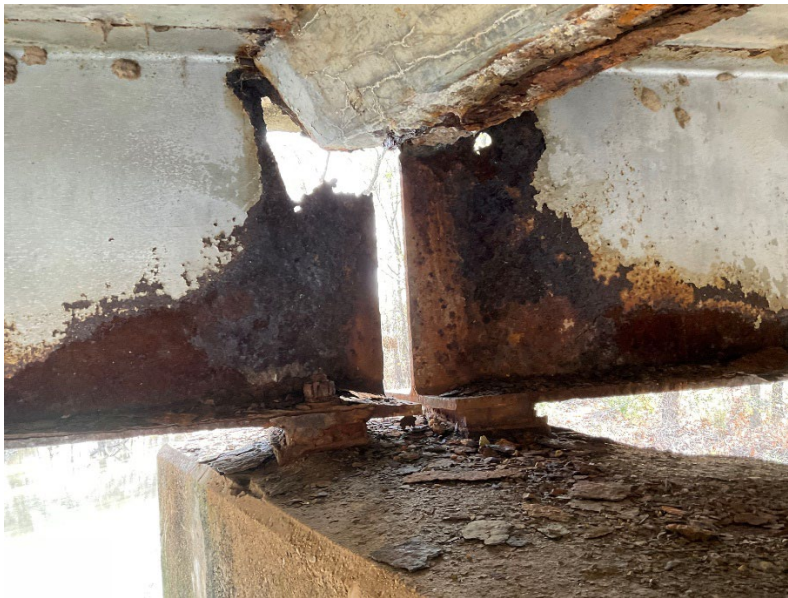
Figure 33. CF of Steel girder end (on the left)
