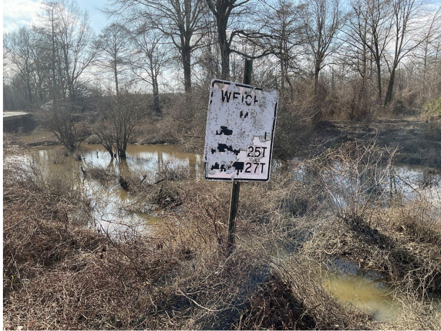
Figure 50. A priority maintenance item for sign that is unreadable due to code 4.
