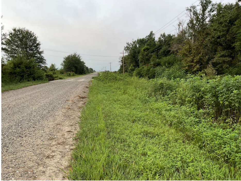
Figure 46. A priority of missing or knocked down load posting sign that should read “10,10,10”
