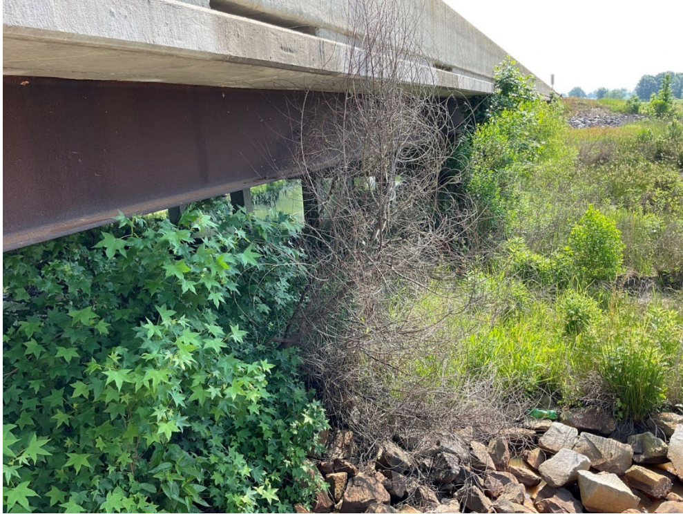
Figure 9. D priority maintenance item for vegetation if limiting inspection or impeding traffic.
