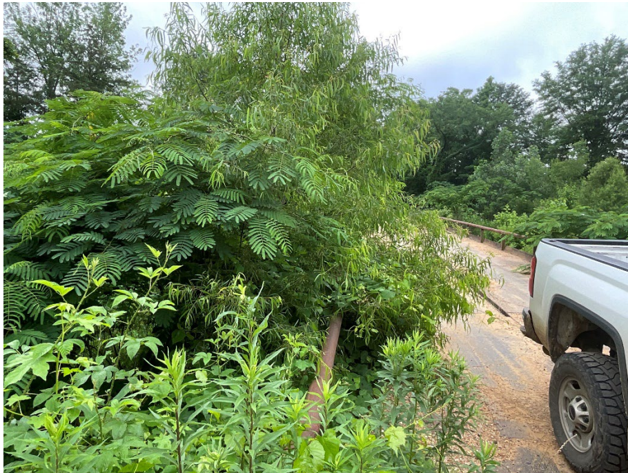
Figure 1. C/D priority maintenance item for vegetation.
