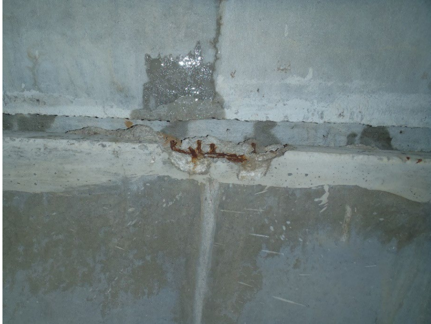
Figure 3. Good example of minor exposed steel in RCBC that does not need a maintenance need.
