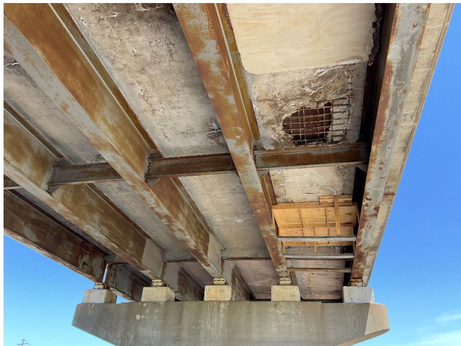
Figure 38. B priority since the plate is in place (underside view)
