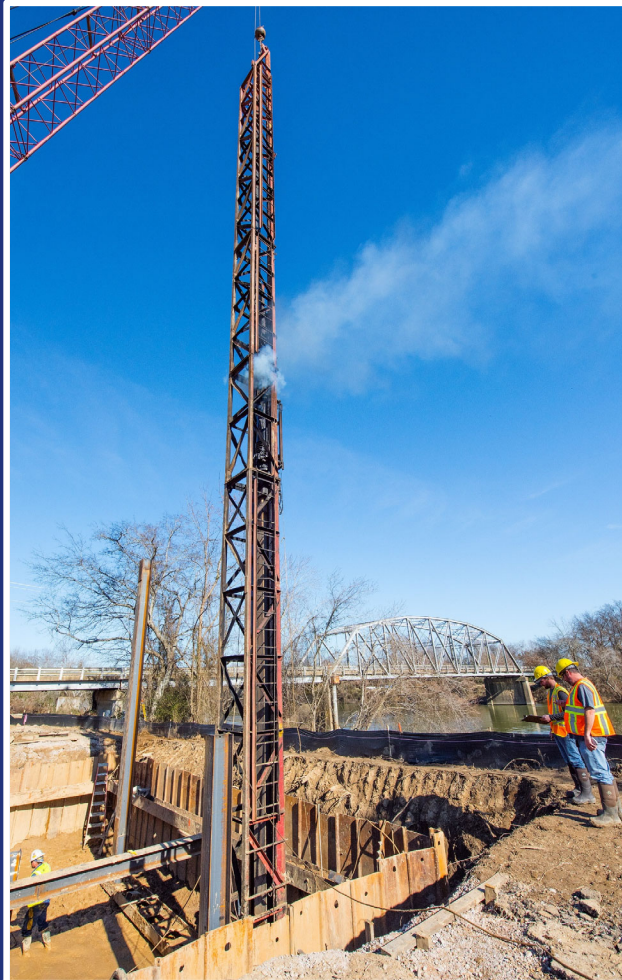
Pile driving operation
