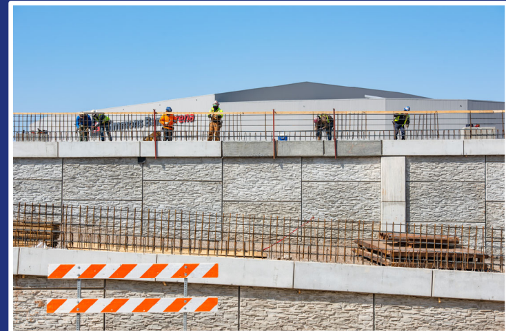
Mechanically stabilized earth wall construction
