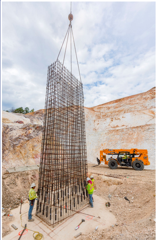
Excavated bridge footing
