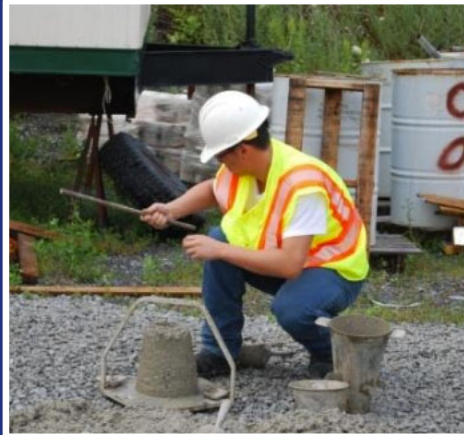
Concrete slump test
