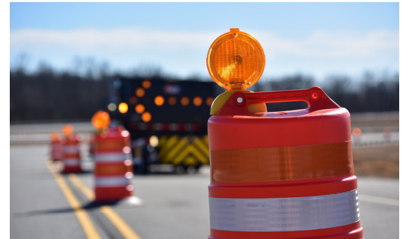
Work Zone Safety in Arkansas Driver's Manual
