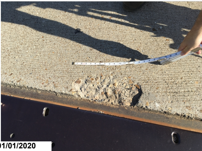
Spall in the left driving lane at the assembly joint seal.
