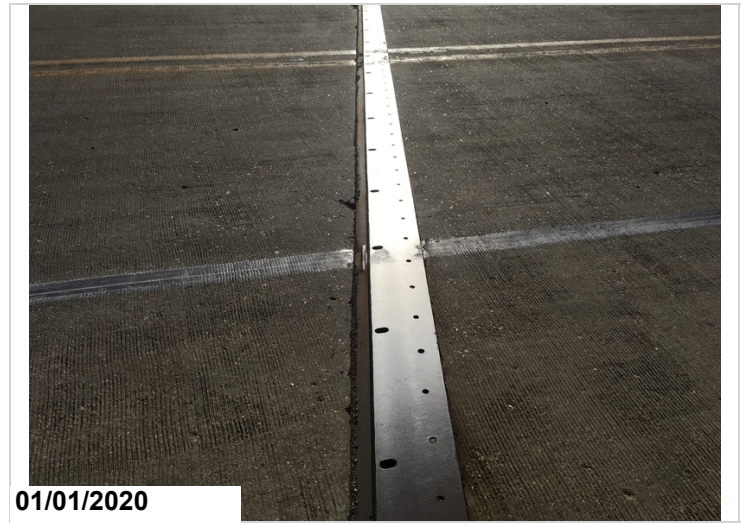
Condition of assembly joint seal.
