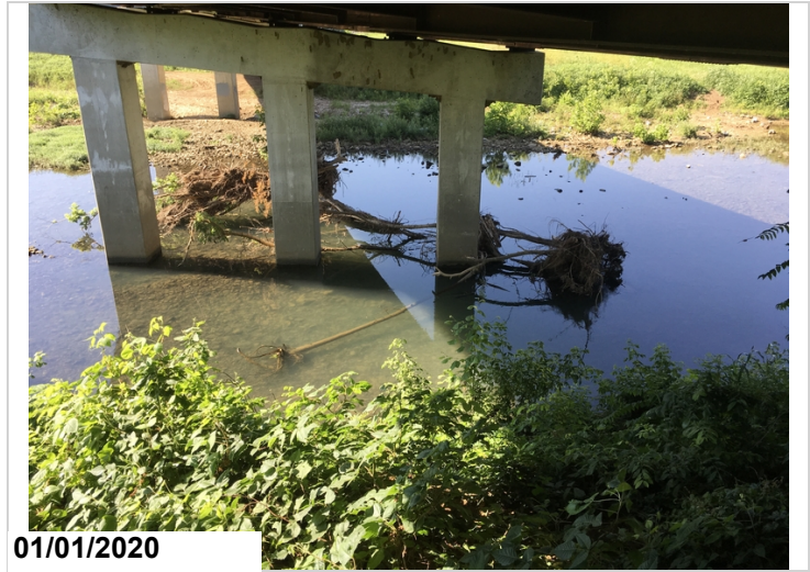
Minor drift accumulation on bent #1 is causing local scour at column #3.
