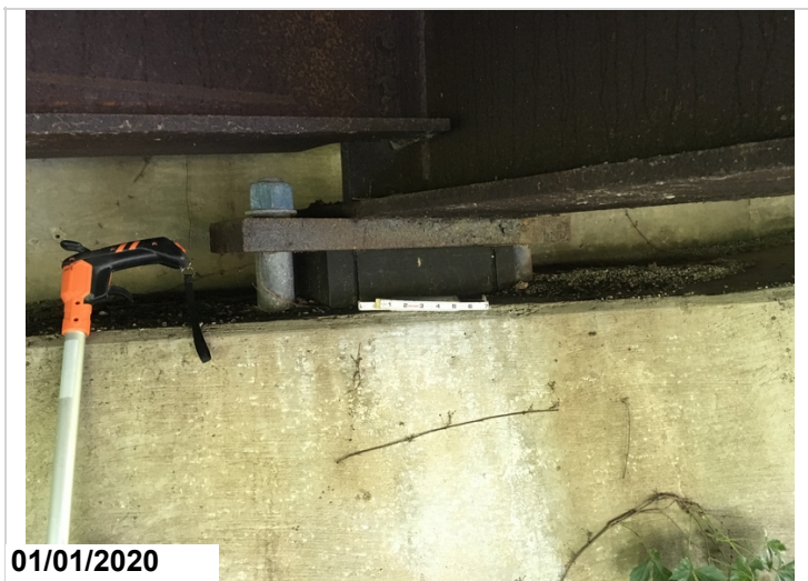
Bearing #4 at abutment #1 showing corrosion on the sole plate.
