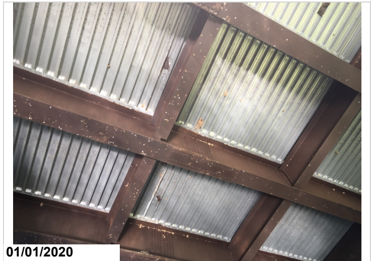
Corrosion in the sip forms in bays 2,3 in span #1 due to leaking construction joint seals. Typical of several locations
