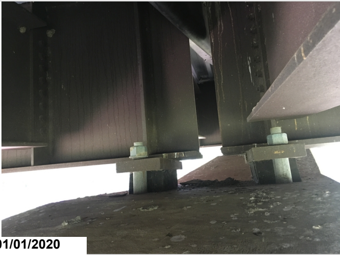
Elastomeric bearing condition at bent #3. Typical of all 10 at this location.
