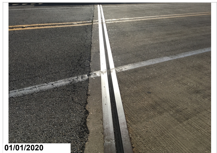
Condition of compression joint seal at abutment #1.
