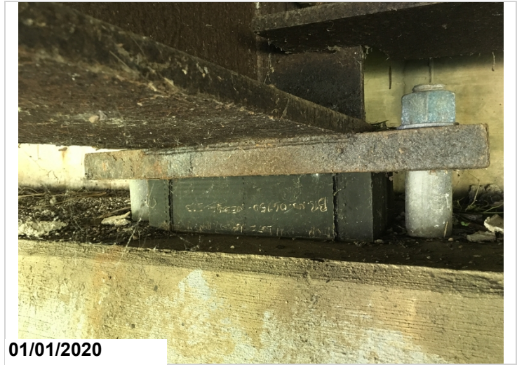
Bearing #3 at abutment #2. Showing minor corrosion with flaking rust.
