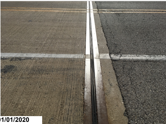
Condition of compression joint seal at abutment #2.
