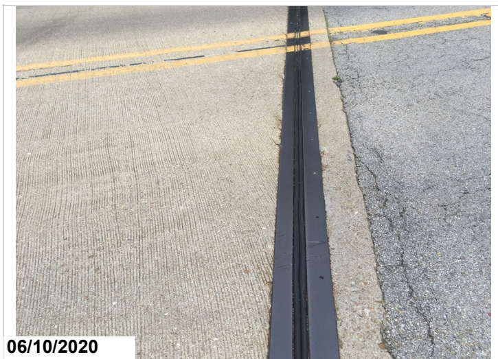
Joint seal condition at abutment 1.
