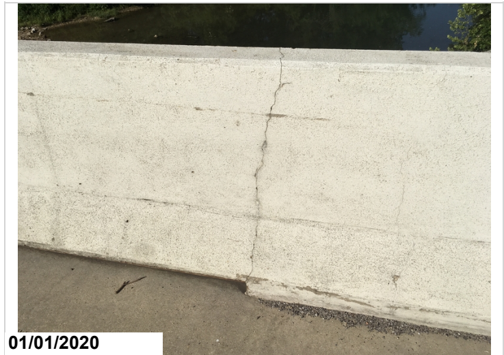
Typical vertical crack in the parapet walls.
