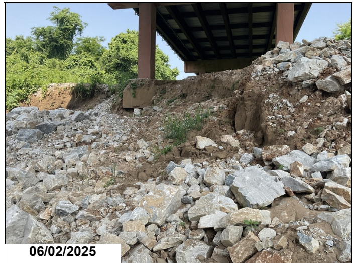
General view of the scoured area at bent #8.
