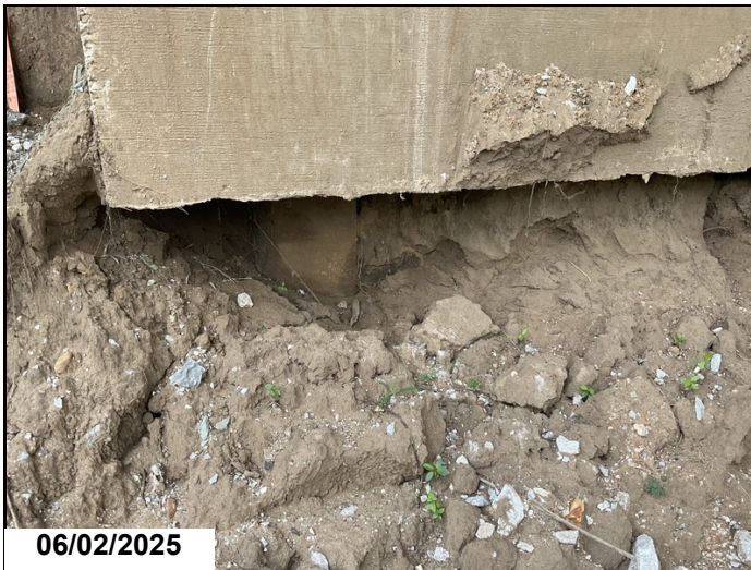
16" of the top of the H pile is exposed.
