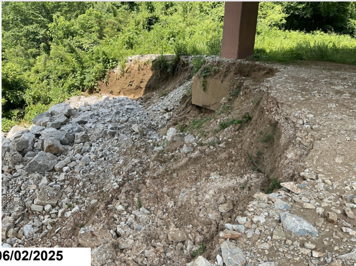
View of scoured area at bent #8.
