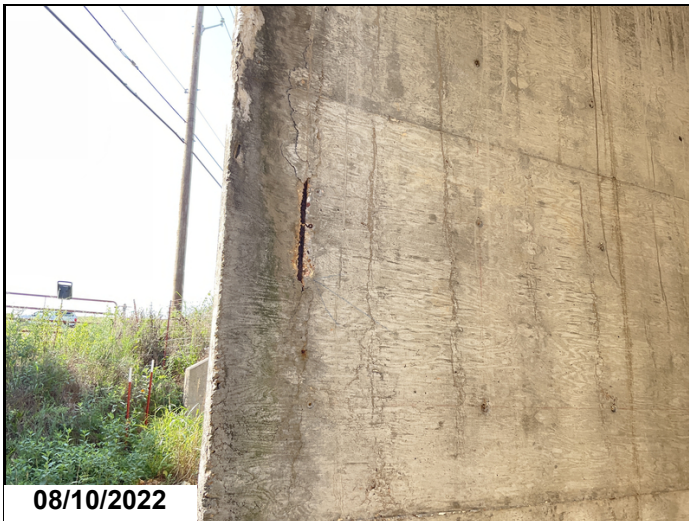
Barrel #4 spalling with steel exposed on the outlet end of wall #4
