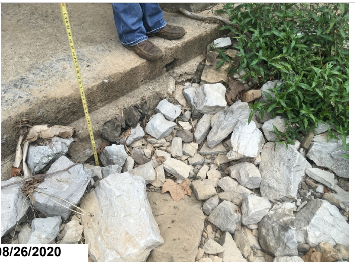
14" of the vertical face of the bottom slab exposed at the barrel 4 outlet. Typical of barrels 2-5.
