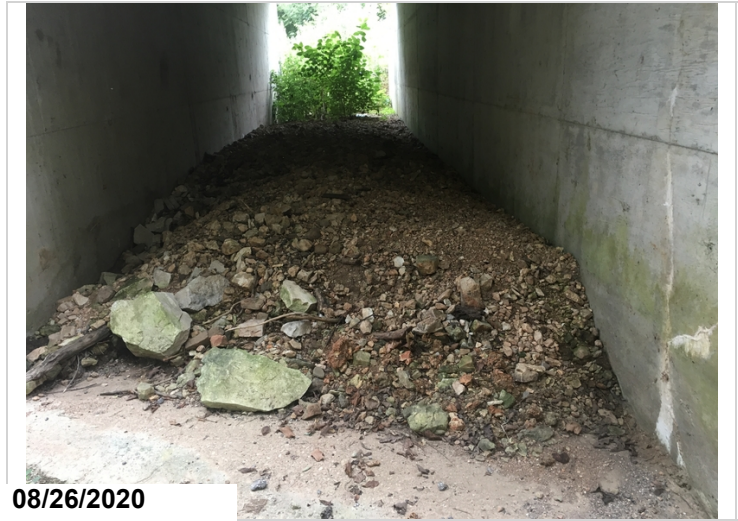
24" of stream bed material build up in barrel 1.
