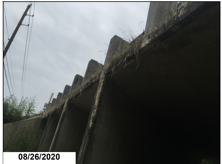
Efflorescence with concrete deterioration on the right edge of the top slab.
