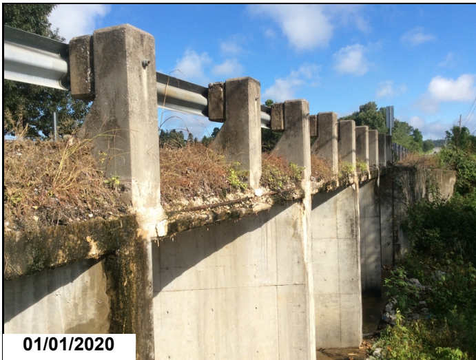
Deterioration on the right edge of the top slab.
