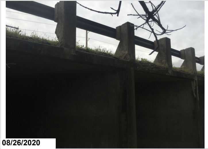
The left end of the bridge railing showing spalling and delamination on the concrete posts.
