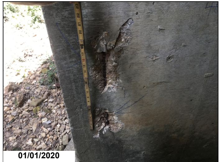
Barrel #2 has exposed rebar at the inlet end.
