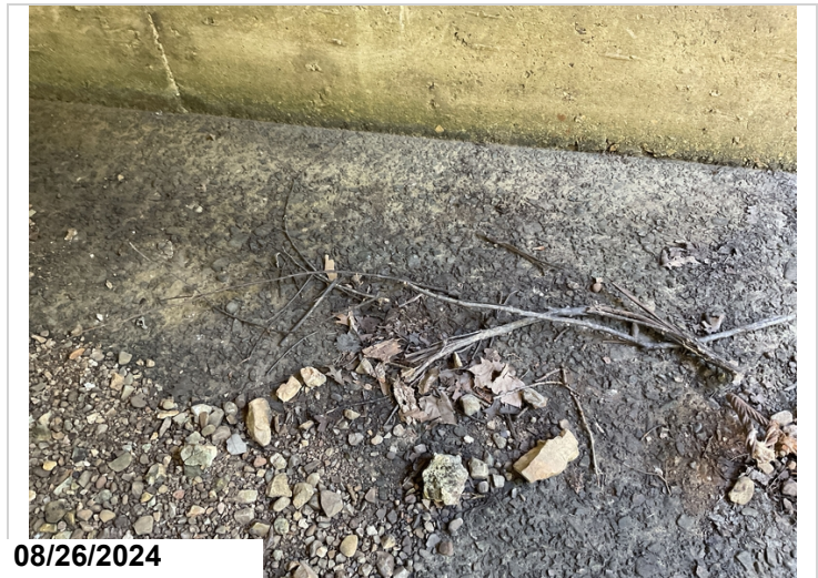
Barrel 1 - 5, Floor: Moderate abrasion.
