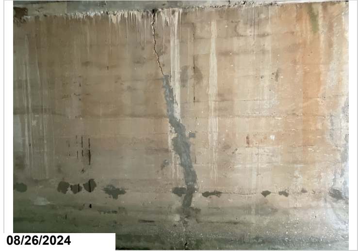
Barrel 5, Back Wall: Large open cracking. 1LF CS3
