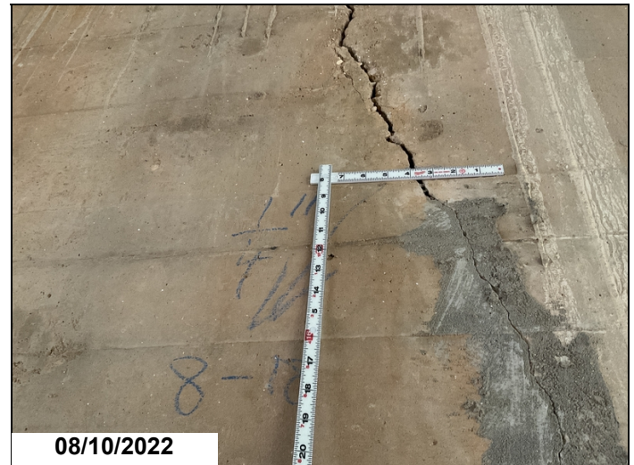
Barrel #5 vertical crack measurement 2022
