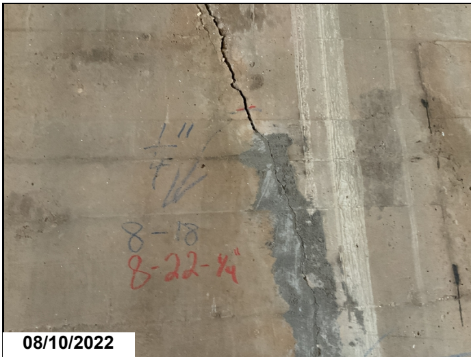
Barrel #5 vertical crack measurement 2022
