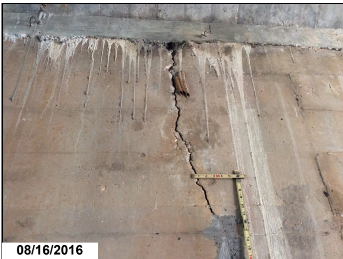
Crack in back wall of barrel #5 at mid section.
