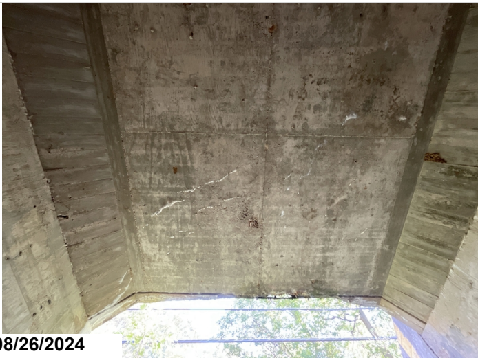
Barrel 5, Top: Cracking with efflorescence with build up. 6LF CS3
