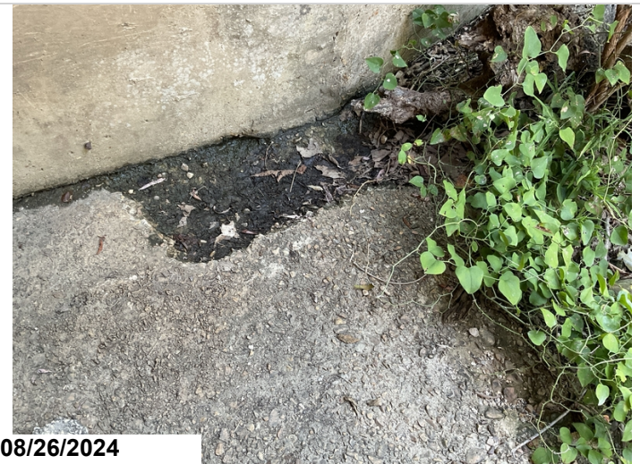
Barrel 5, Right, Floor: Spalling.
