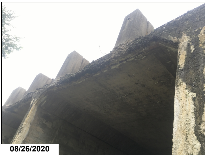
Top slab deterioration and spalling typical of both sides of the structure.
