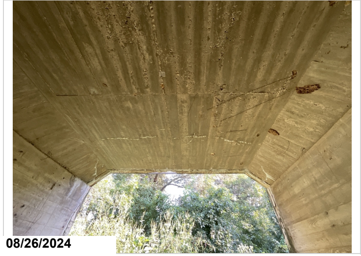
Barrel 2, Top: Cracking with efflorescence with build up. 6LF CS3
