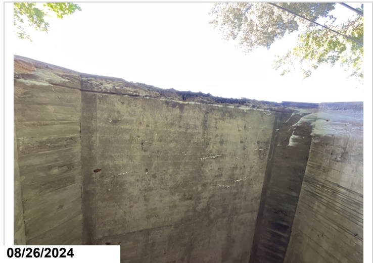
Barrel 4, Top: Cracking with efflorescence with build up. 6LF CS3
