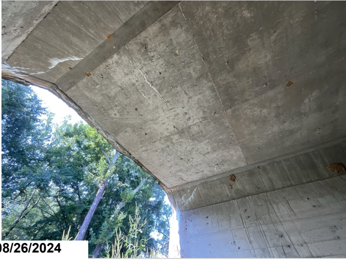
Barrel 2 & 3, Top: Cracking with efflorescence with build up. 12LF CS3
