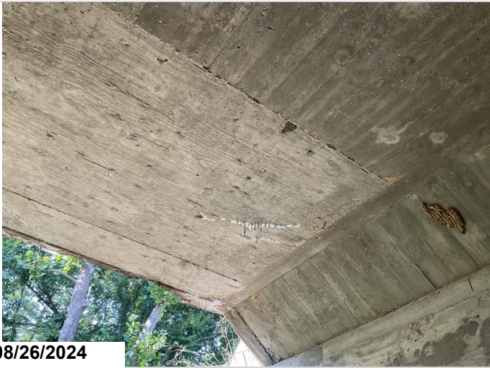
Barrel 1, Top: Cracking with efflorescence with build up. 6LF CS3
