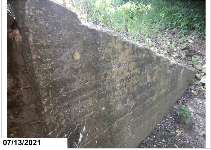
Spalling with no rebar exposed in the top edge of the barrel #3 right wing.
