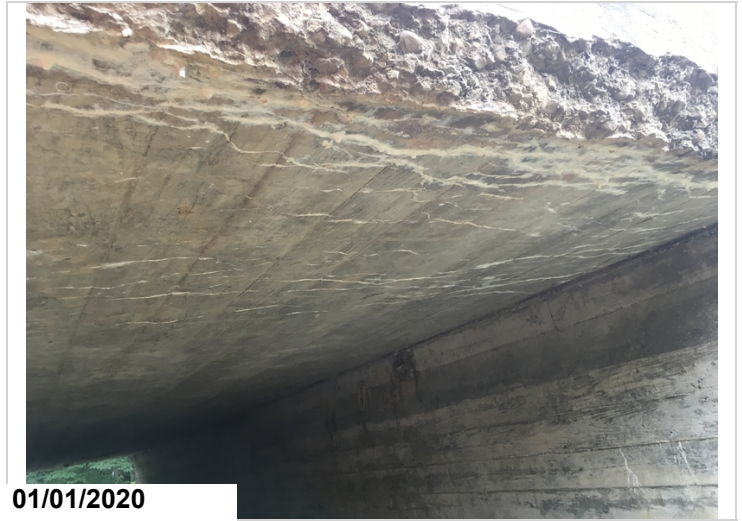
Top slab condition at the outlet end of barrel #3. Showing efflorescence map cracking. Typical of all 3 barrels.
