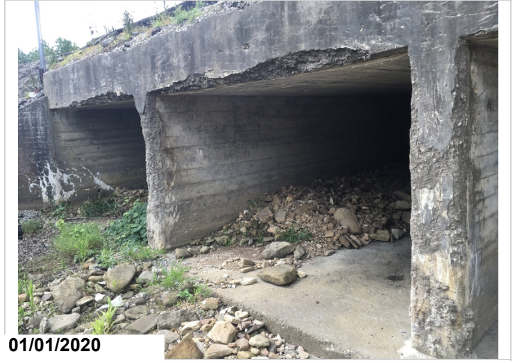
Concrete deterioration with map cracking and efflorescence at the outlet end of all 3 barrels.
