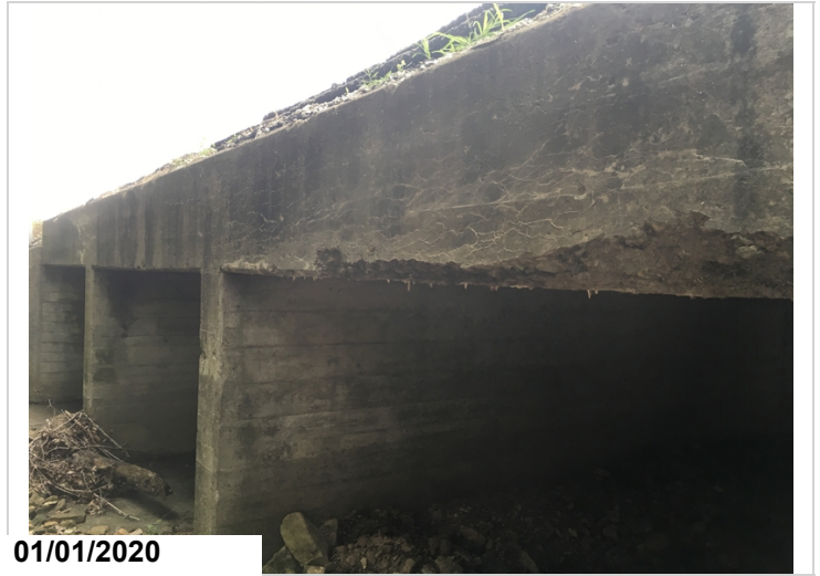
Concrete deterioration with map cracking and efflorescence on the right head wall.
