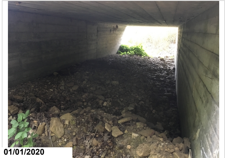
Stream bed material build up in barrel #3.
