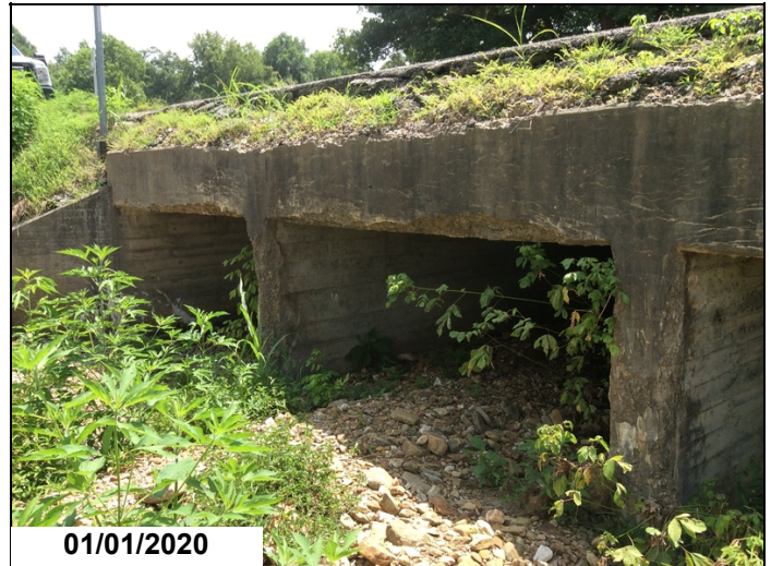
Barrel 2 and 3 soft deteriorated concrete located in head wall an interior wall of boxes outlet end
