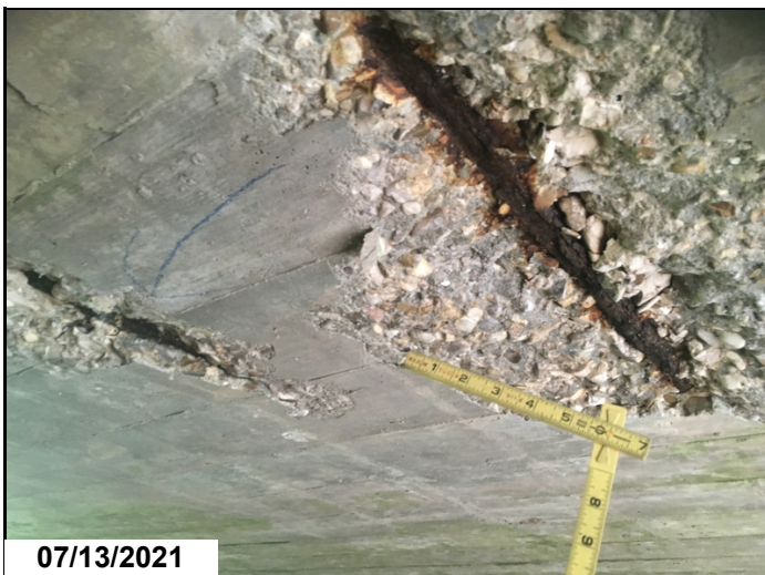
Spalling with rebar exposed in the top slab of barrel #3.
