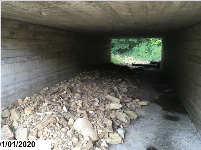
Minor amount of stream bed material build up in barrel #2.
