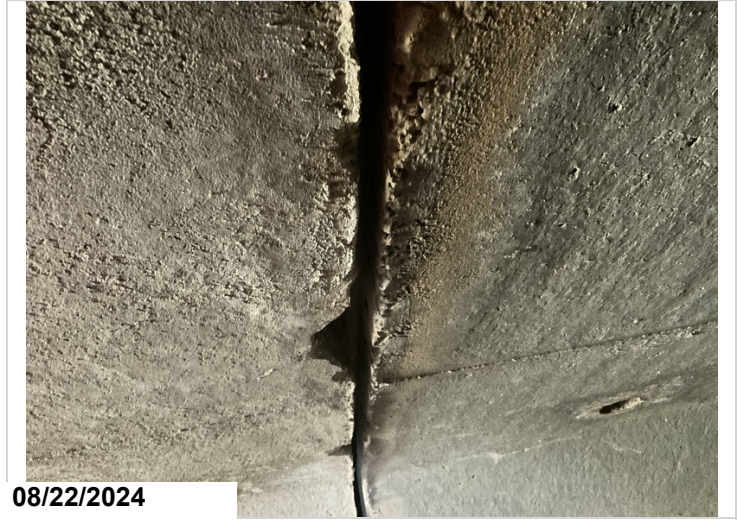
Barrel 2, Units 14, 17 & 18: Spalling. 3LF CS2
