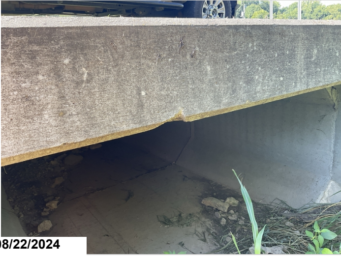
Barrel 2, Right, Head Wall: Spalling. 1LF CS2
