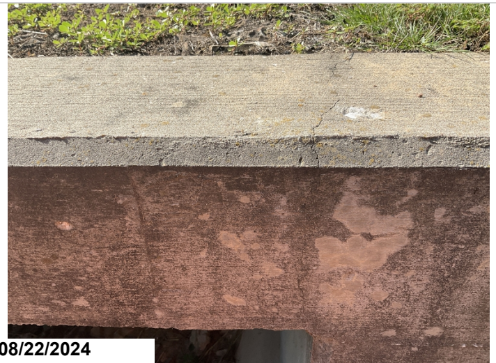
Barrel 3, Left, Head Wall: Cracking. 1LF CS2
