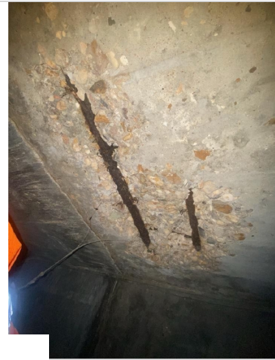
Barrel 3, Top: Spalling with exposed reinforcing steel with section loss. 1LF CS3
