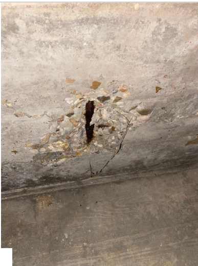
Barrel 3, Top: Spalling with exposed reinforcing steel with section loss. 1LF CS3
