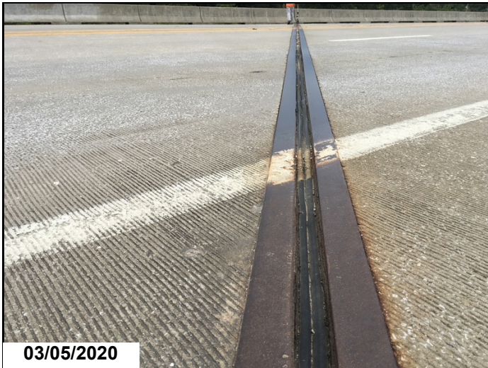
Condition of joint seal #2. Typical of joint seal # 2,3.
