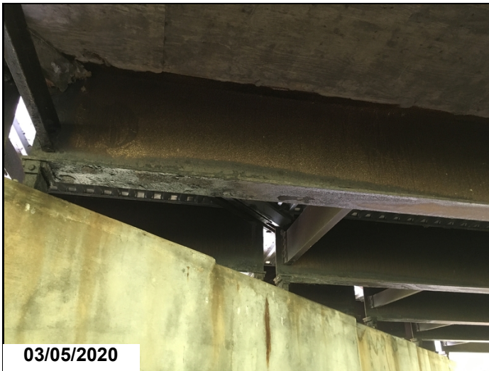
Typical bottom flange corrosion in span #1. Typical of many locations.
