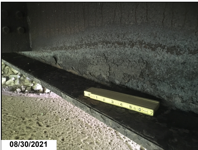
15' of Cs3 corrosion on beam #6 at the end of span #1.
