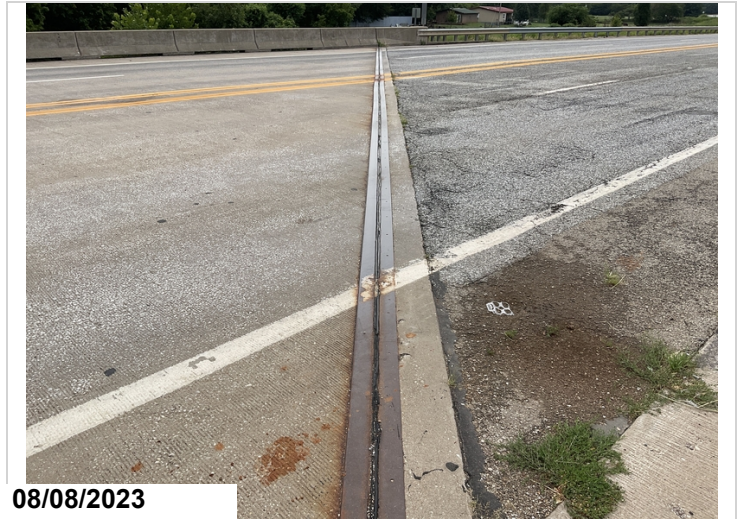
View of joint at abutment #2
