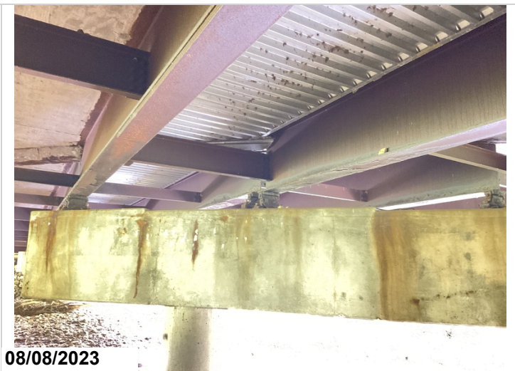
Bent #1 girders at bearing #7 have flaking rust adjacent to expansion joint
