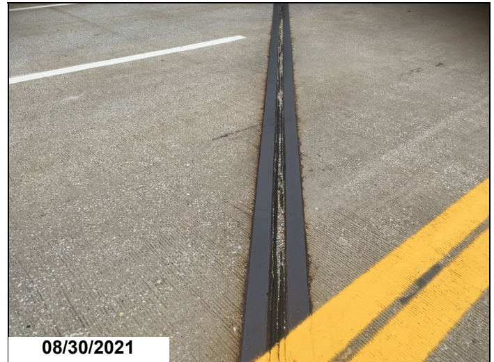
Seal condition at bent #1.
