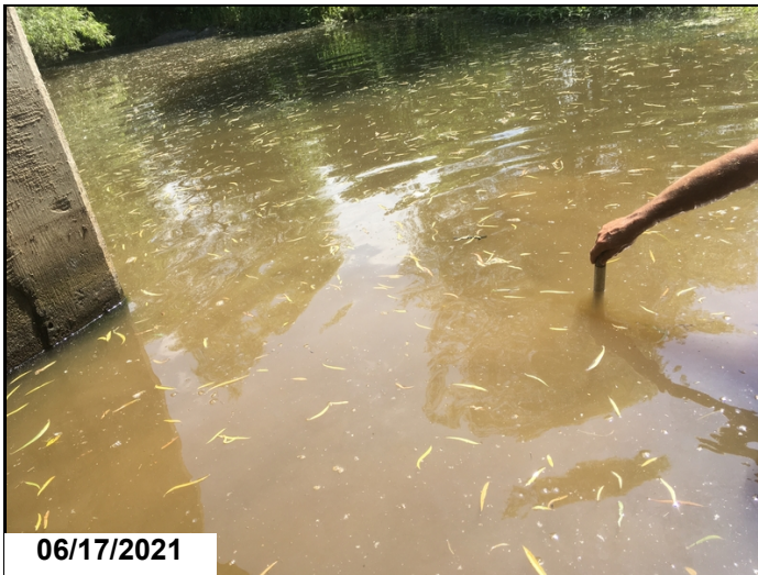
Barrels #2,3 have 3' of scour at the outlet end.
