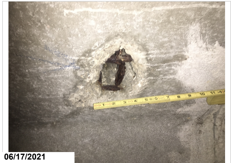
Unit #10 has a spall with rebar exposed in the top slab at a lifting lug area.
