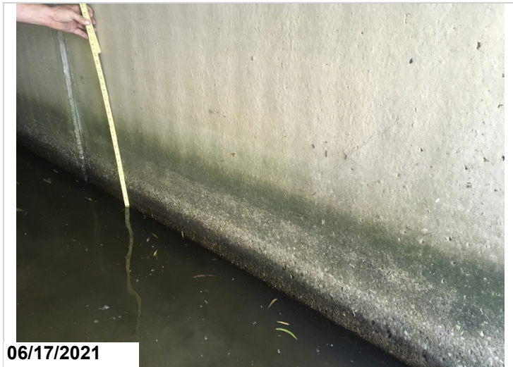
Abrasion on the lower 2' of all precast units in barrel #1.
