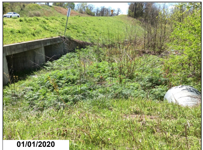
West channel has vegetation restricting water flow.
