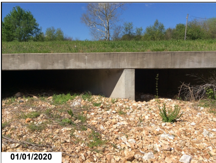
Barrels #1 & #2 have heavy gravel accumulation outlet end.
