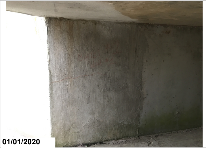
Barrel #3 wall #3 right has a short duration hairline horizontal crack.
