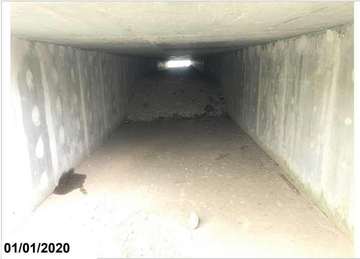
Barrel #1 has gravel accumulation restricting barrel by 60%.
