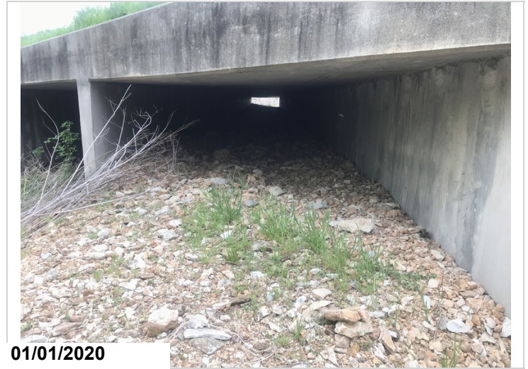
Barrel #2 has gravel accumulation restricting barrel by 60%.
