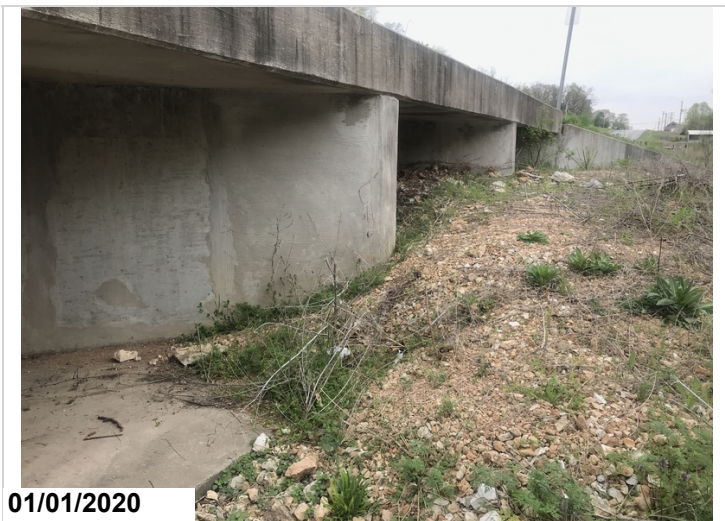
Barrels #1 & #2 left approximately 60% of gravel accumulation.
