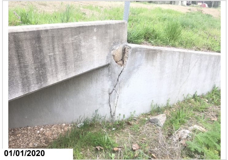
Northeast wingwall vertical cracking with basketball sized spall with steel exposed.
