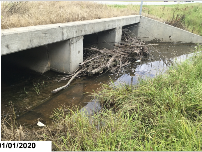
Drift accumulation at the inlet end of barrels #1,2.
