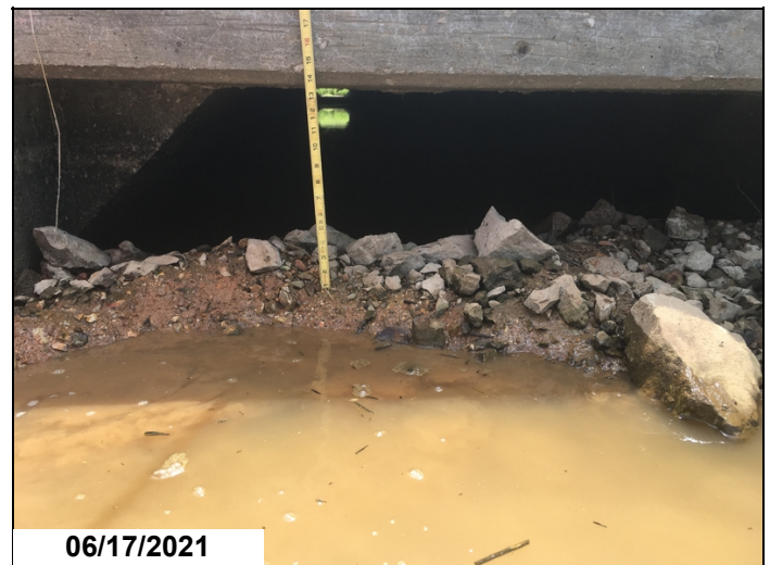
Barrel #3 has 2' of stream bed material build up at the outlet end.
