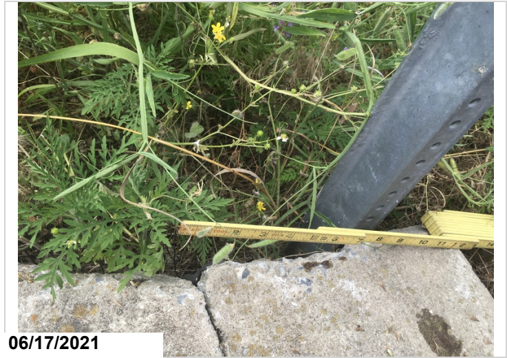
Shallow spill at the end of the left headwall.
