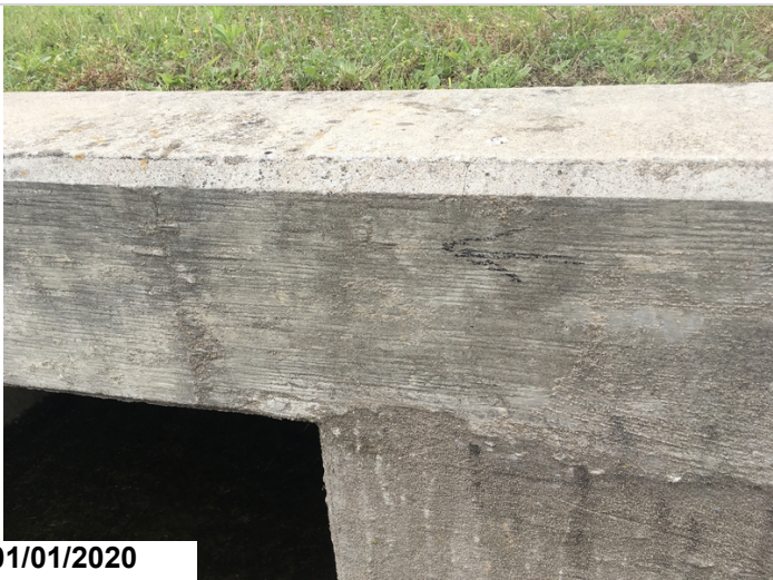
Typical cracking at the head walls.
