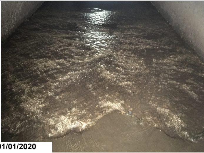
View of abrasion in barrel floor.
