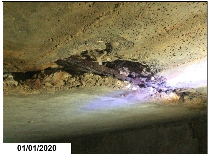
01/01/2020 Barrel #2, top slab-Exposed reinforcing steel at construction joint where culvert was widened.
