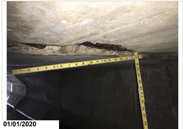
Barrel #2, top slab-Exposed reinforcing steel at construction joint where culvert was widened approximately 40' from inlet end.
