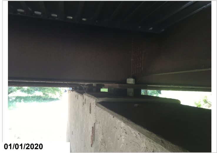
Bearing condition at bent #2. Typical of all 9 at this location.
