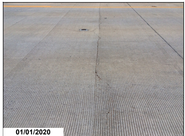
North approach slab-Transverse cracking.
