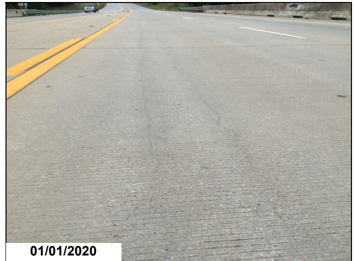
Longitudinal cracking inside Southbound lane.
