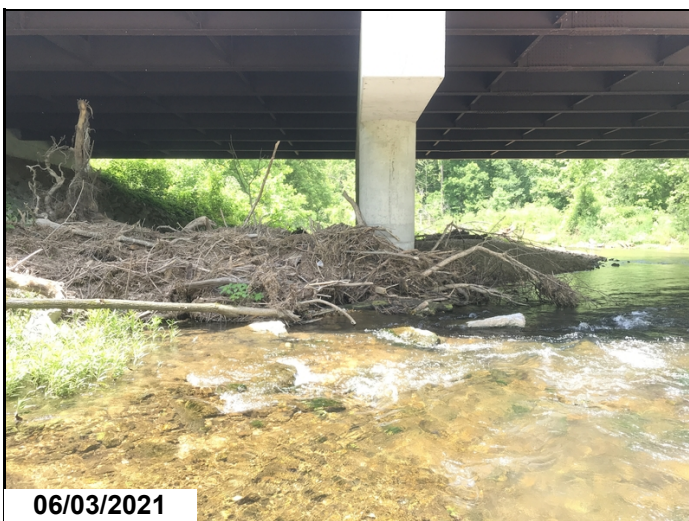
Heavy drift accumulation at bent #2
