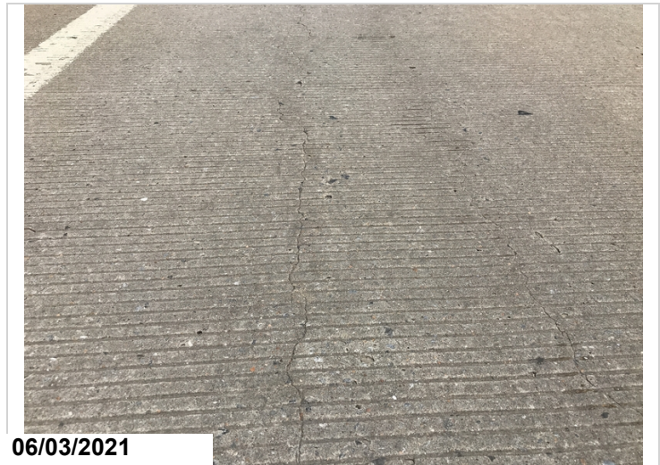
Typical view of longitudinal cracking.
