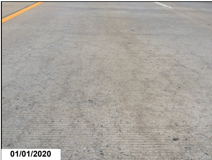
South approach slab, Southbound lanes-Mapcracking.
