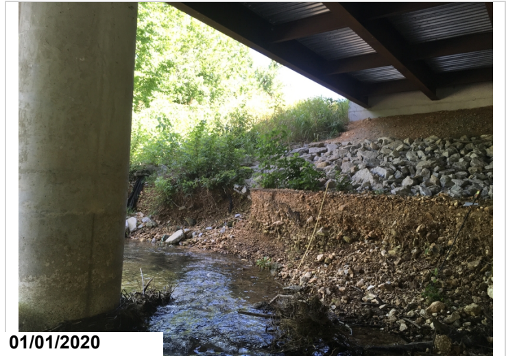
Embankment erosion at the abutment #1 slope. The width from bank is 14' 3" to column #3 at bent #1.
