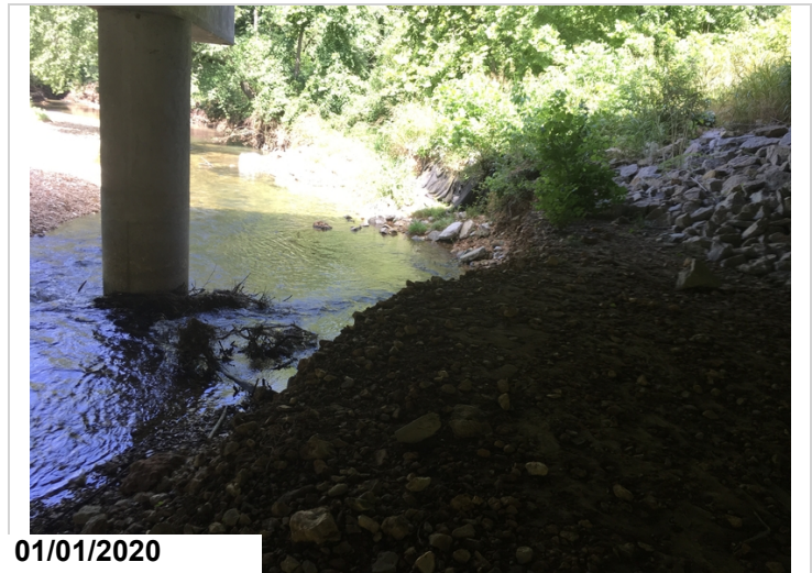
General view of abutment #1 embankment erosion.
