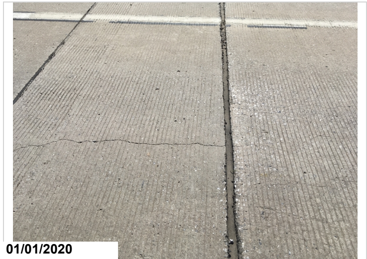
Pourable joint seal condition at the abutments.
