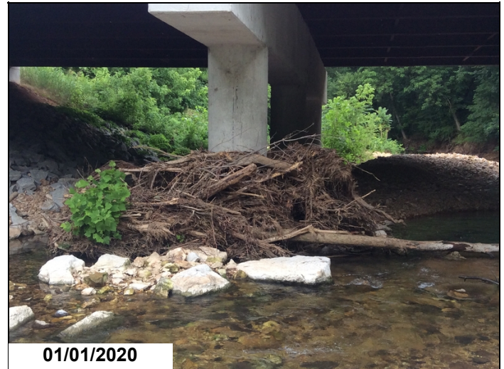
Channel-Drift accumulation at bent #2.
