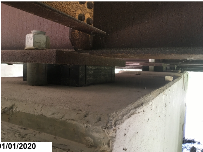
Bearing condition at bent #1. Typical of all 9 at this location.
