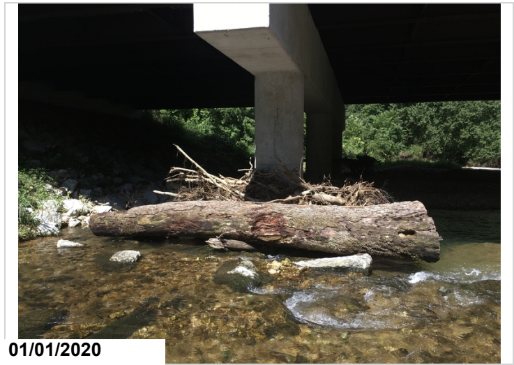
Drift accumulation at the upstream side of bent #2.
