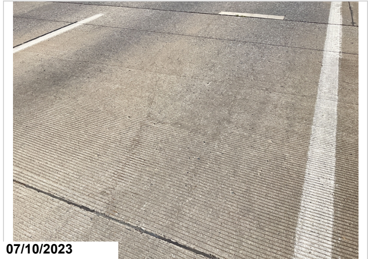
Typical view of deck cracking
