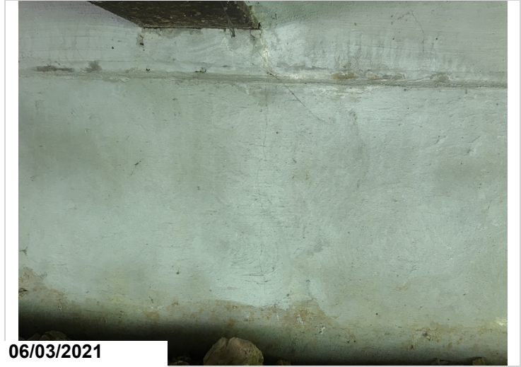
Vertical cracking at abutment #2.
