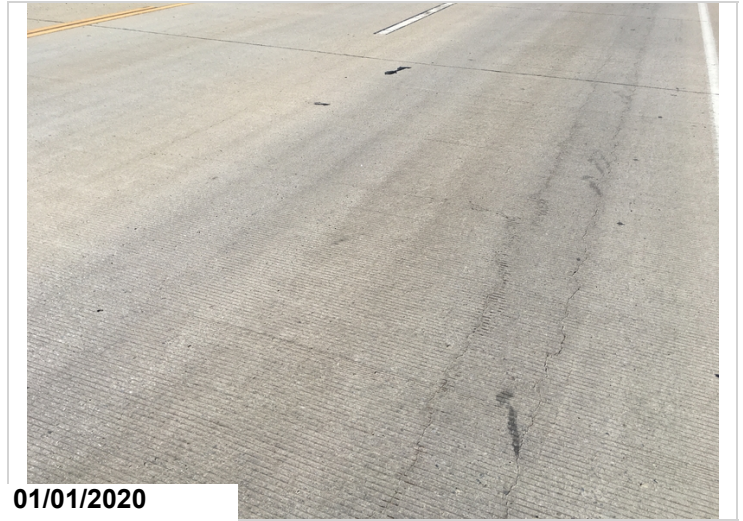
Typical view of driving surface. Note the longitudinal cracking.
