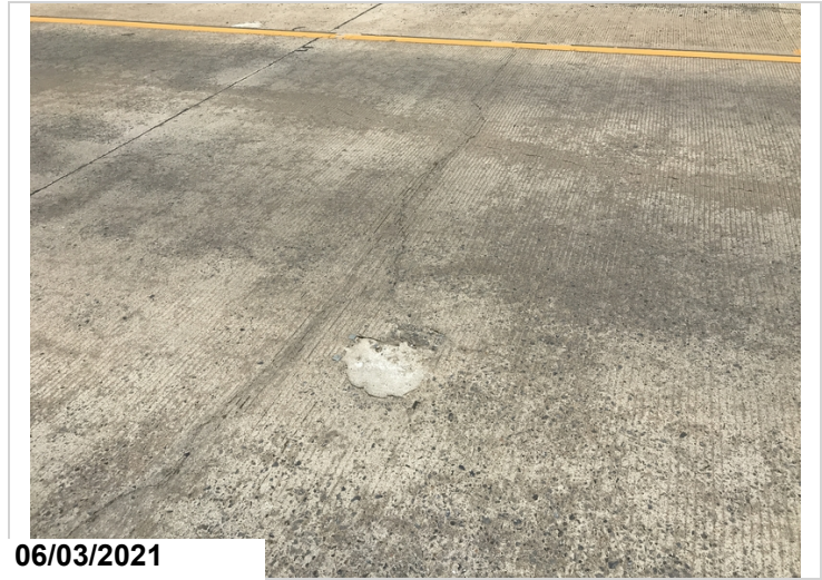
View of failing repairs in North abutment
