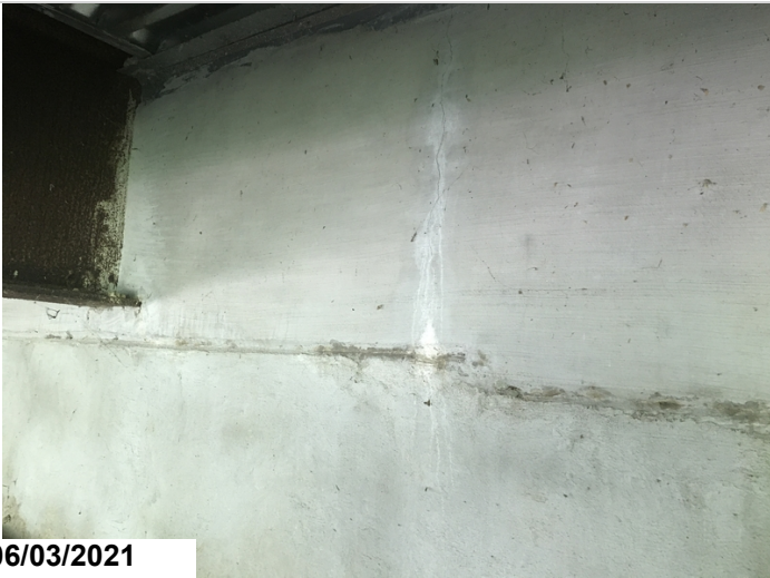
Vertical cracking with efflorescence at abutment #2.
