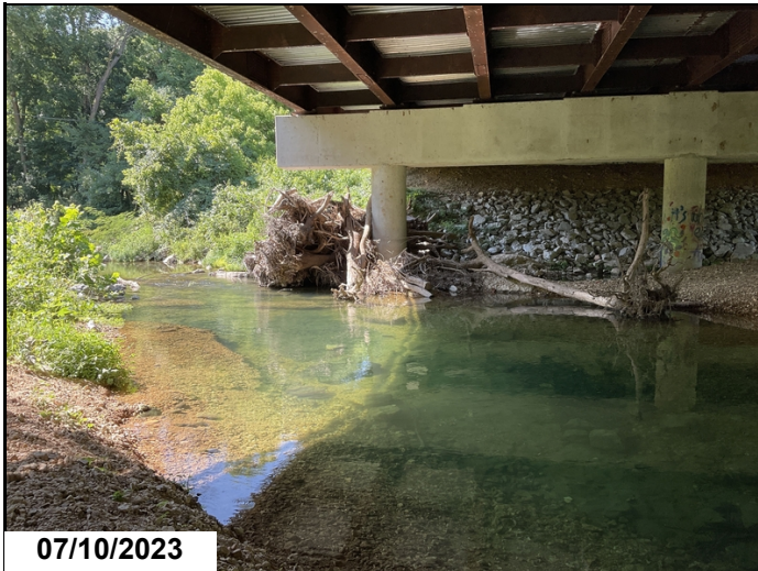
Bent #2 upstream large tree and drift is causing localized scour
