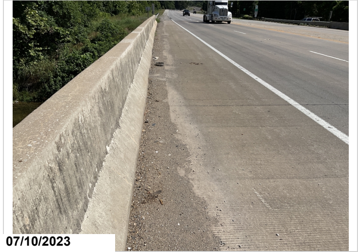
Typical debris in gutterline
