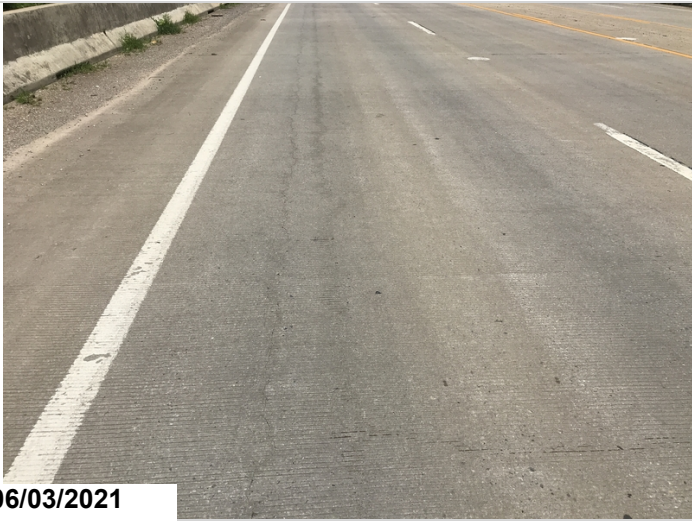
Typical view of longitudinal cracking.
