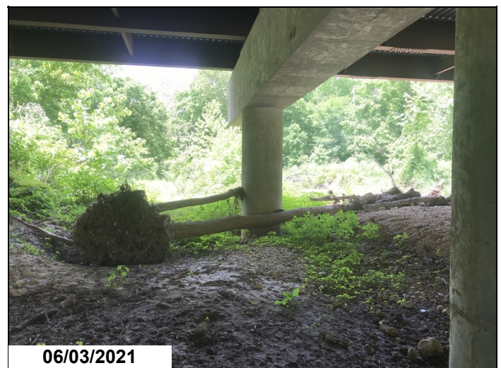
Large tree bent #2 column #3.
