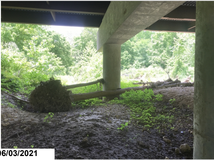
Large tree bent #2 column #3.
