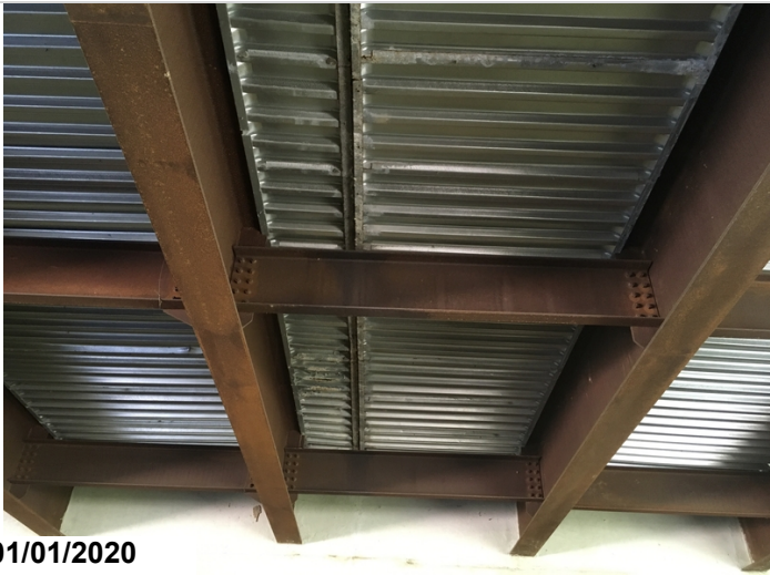
Sip corrosion in bay #4 at abutment #1. Typical of all 3 spans.
