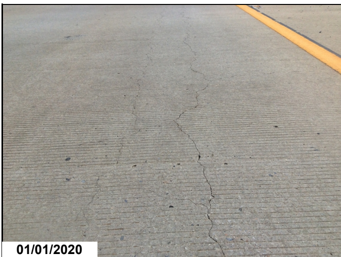
Span #3-Deck cracking.
