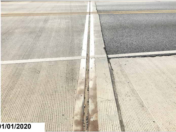
Abutment #1 joint material.
