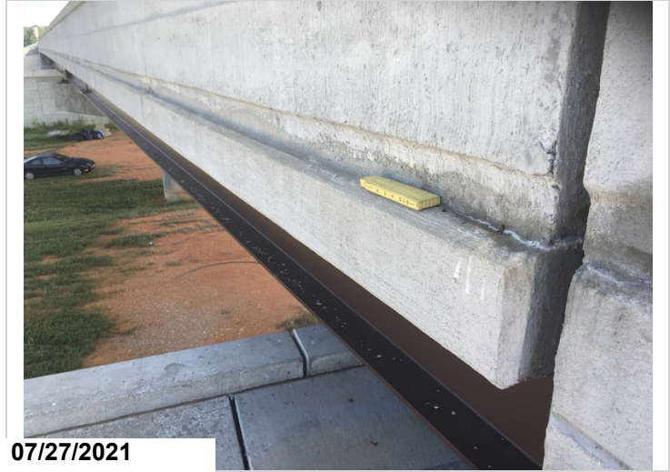
The beginning left deck edge of the exterior of span #1 has 1' of cs2 efflorescence.
