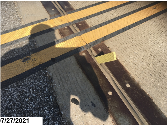
torn area in the abutment #1 pourable seal. right lane.
