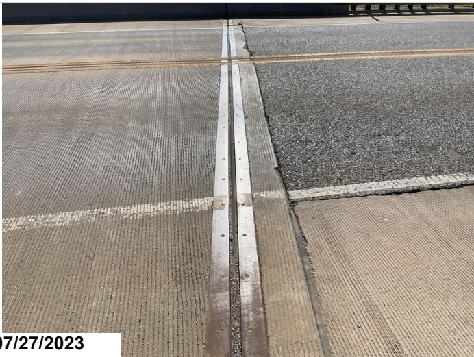
View of joint at abutment #1
