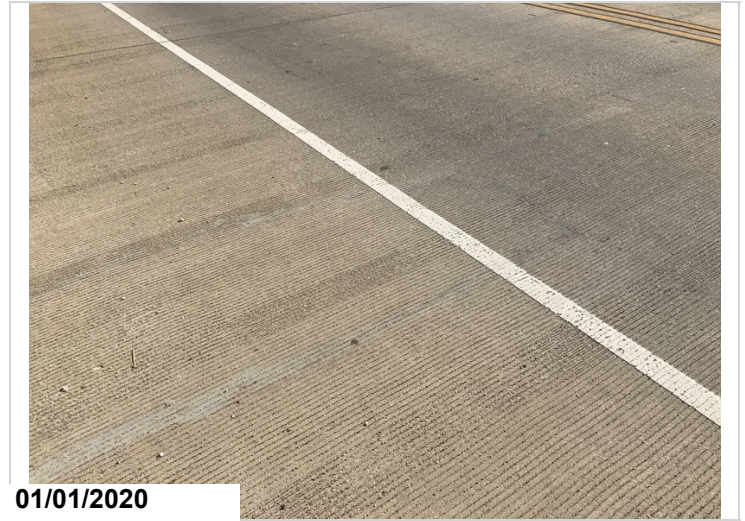
Contractor has made attempts to seal deck surface cracking.
