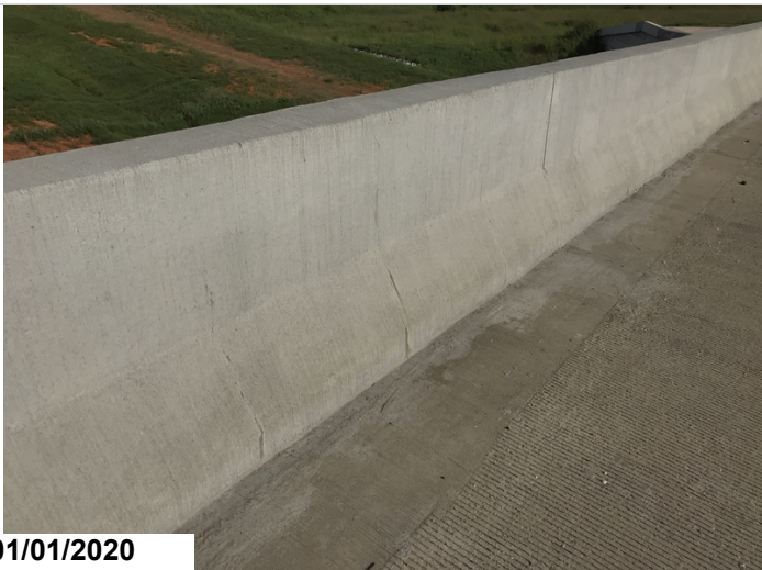
Typical cracking in parapet
