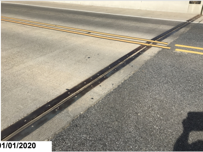
Contractor has placed sealant for longitudinal cracking on top of abutment #2 backwall.
