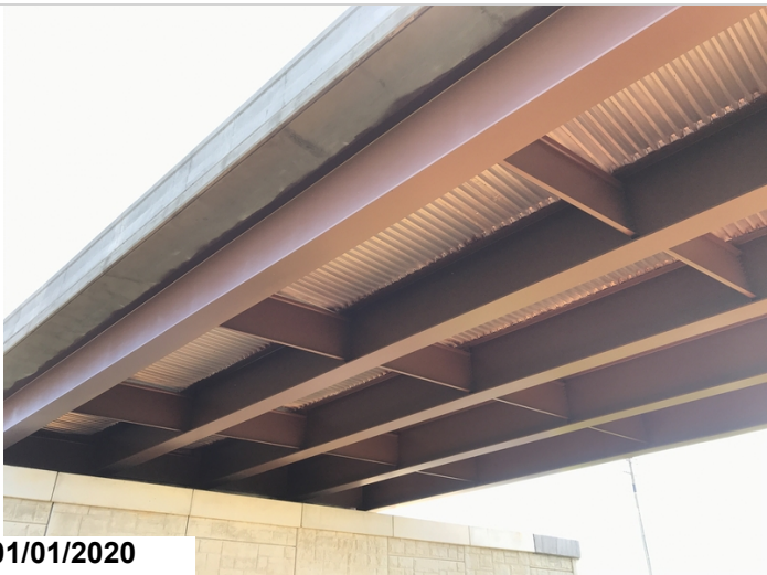
Typical view of final protective system applied to superstructure.
