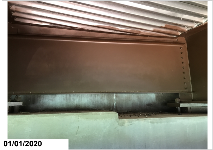
Abutment # 1 bay #2 efflorescence in abutment backwall
