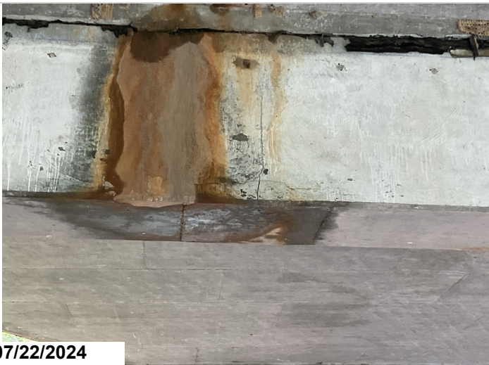
Bent 3, Center: Minor cracking. 2LF CS2
