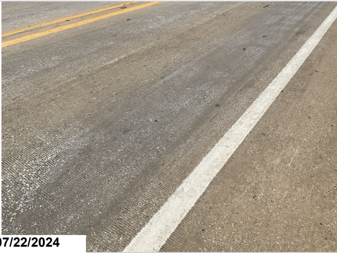
Span 1 - 9, Left: Map cracking. 630SF CS3
