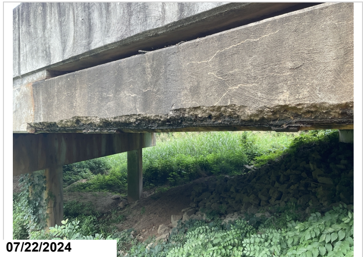
Spans 4 - 9: Spalling with exposed reinforcing steel with section loss. 115SF CS3
