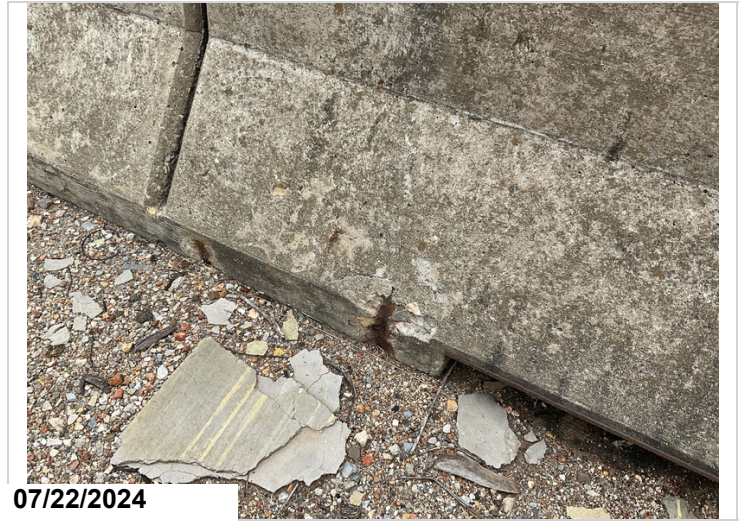
Spalling with exposed reinforcing steel with section loss. 5LF CS3
