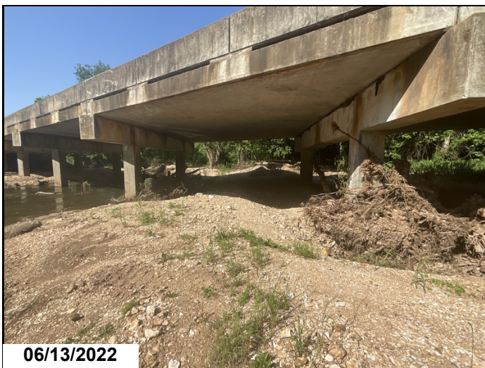
Large trees at bents 4-6 that are causing localized scour.
