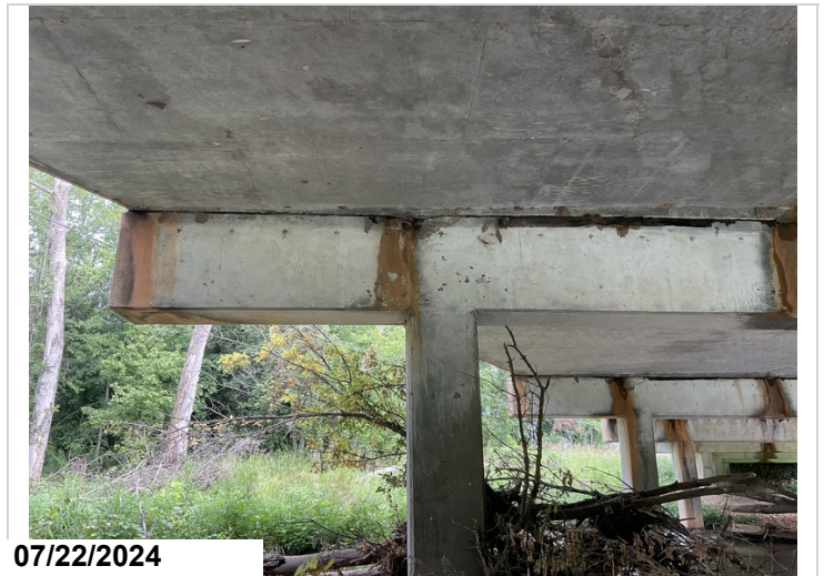
Bent 3, Left: Spalling with exposed reinforcing steel with section loss. 2LF CS3
