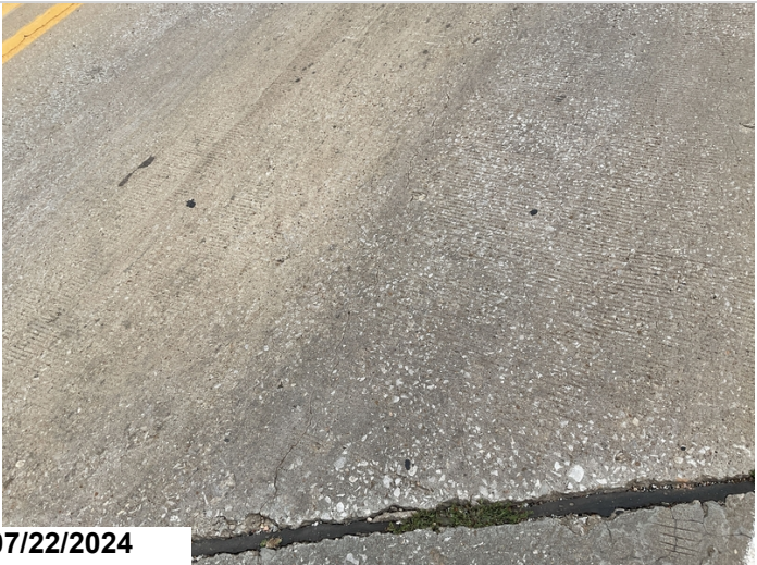
Span 4, Right: Longitudinal cracking. 10SF CS2
