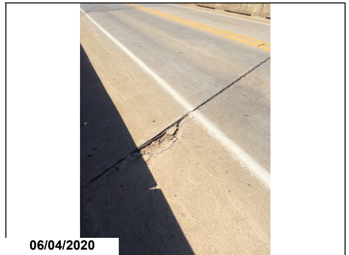
Deck surface Span 2 at bent 1 right spalled area.
