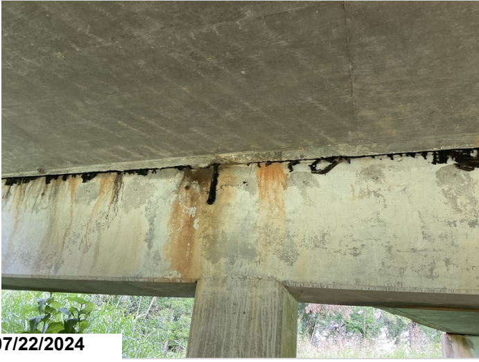
Bent 7, Left: Delam. 2 LF CS2
