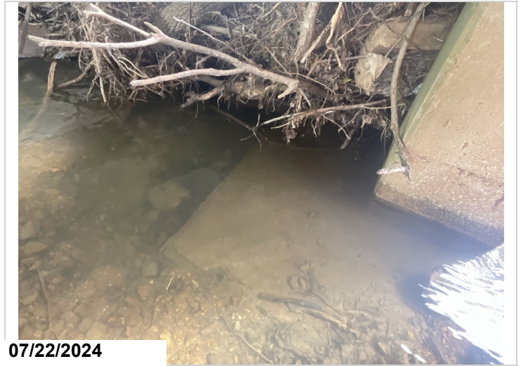
Bent 4, Column 1: Footing exposed with minor scour.
