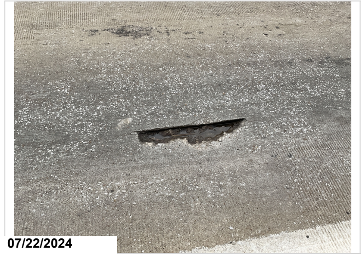
Span 9: Spalling with exposed reinforcing steel with section loss. 2SF CS3
