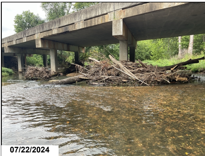
Bents 3 - 5: Large drift blocking channel. Localized scour at bent 4.
