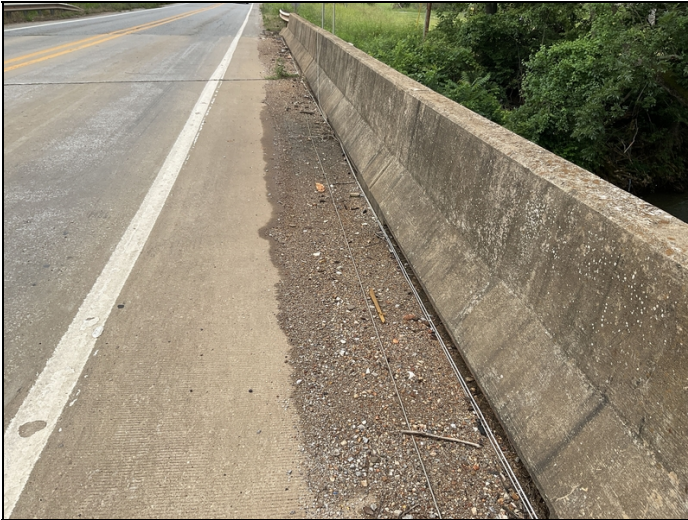
Typical debris in gutter lines.
