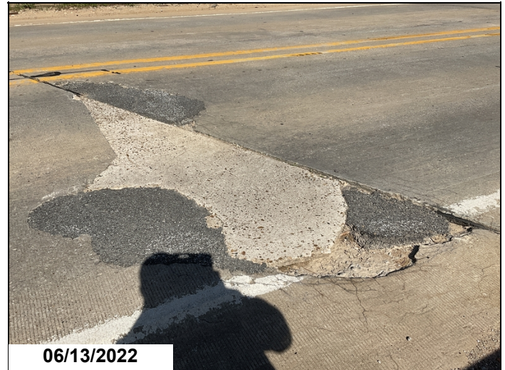
Deck surface over bent #2 concrete and asphalt patches right side. Some of the asphalt patching is failing at this inspection
