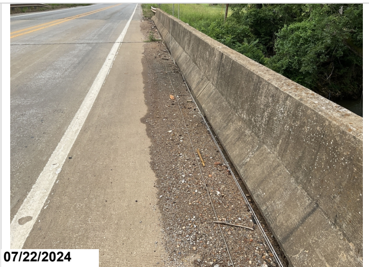
Typical debris in gutter lines.
