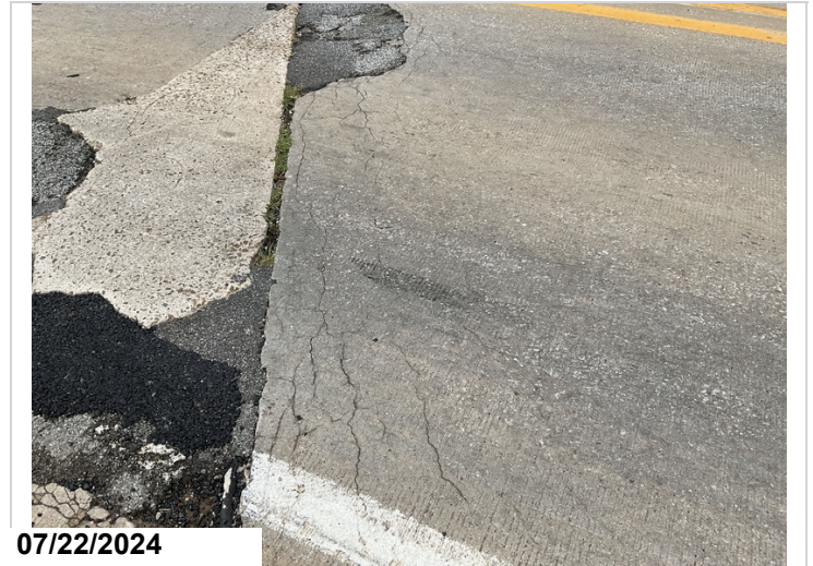
Span 3, Right: Cracking. 8SF CS3
