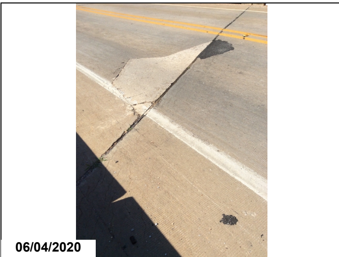
Deck surface Span 2 & 3 at bent 2 right side spalling patched areas.
