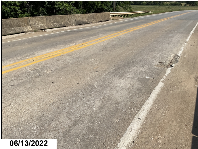
Deck surface span #8 spalling with steel exposed
