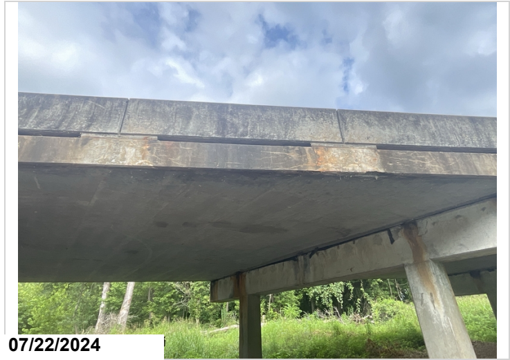
Span 5, Right: Cracking with efflorescence with build-up. 6SF CS3
