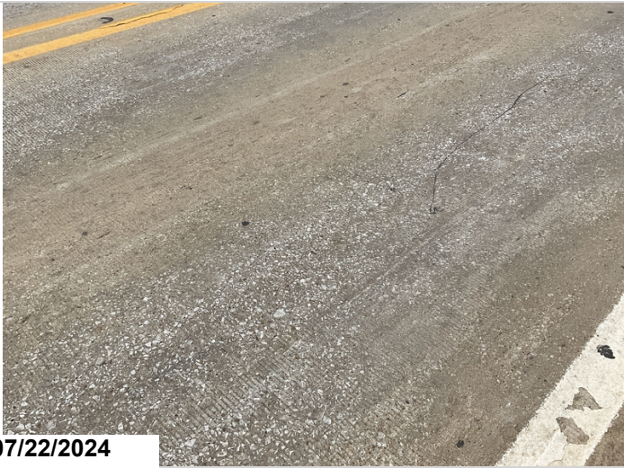
Typical abrasion & cracking in wheel paths.
