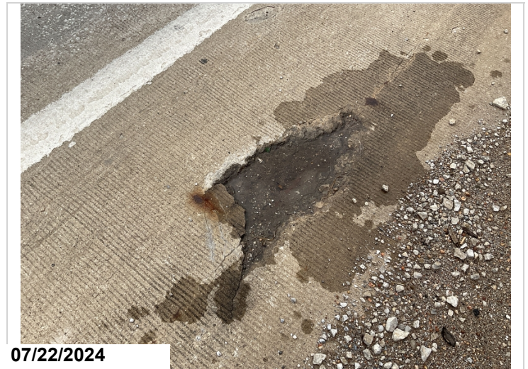
Span 8: Spalling with exposed reinforcing steel with section loss. 5LF CS3
