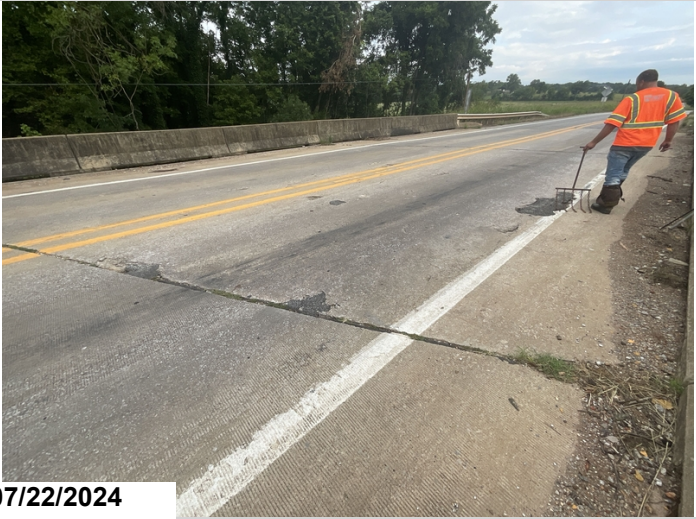
Span 8: Spalling with and without asphalt patches 17SF CS3 Span 8: Delam. areas 108SF CS2
