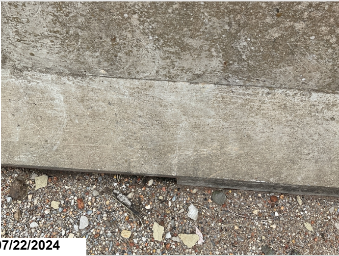
Cracking. 182LF CS2
