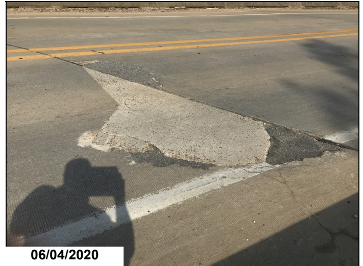
Deck span #2 right failing concrete and asphalt patches.
