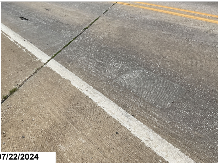
Span 8 & 9: Sound patches. 22SF CS2
