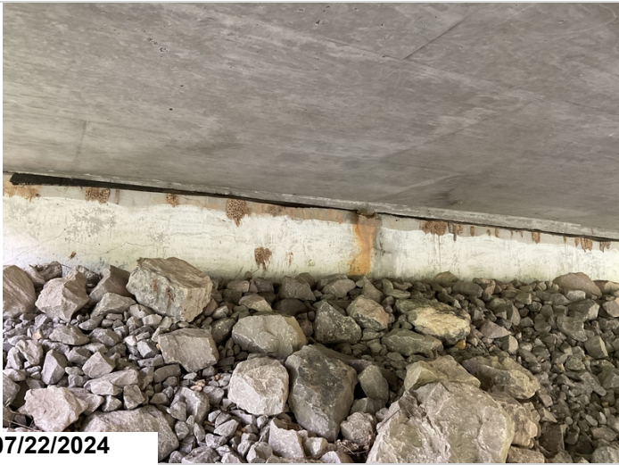
Abutment 1: Minor cracking. 41LF CS2
