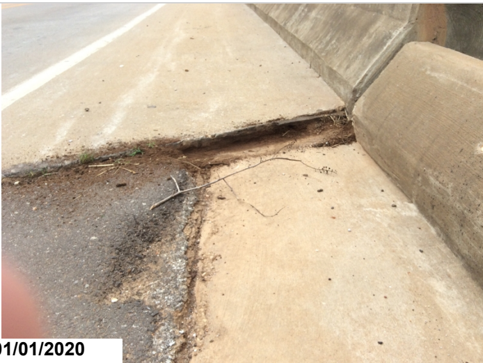
Abutment #2 right approach gutter has approximately 3" lip.
