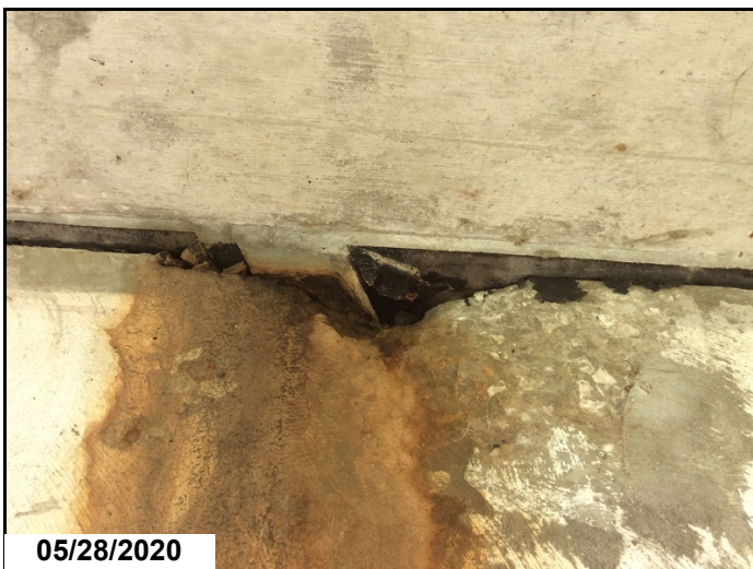
Spall with rebar exposed at top of cap at left side of bent 8.
