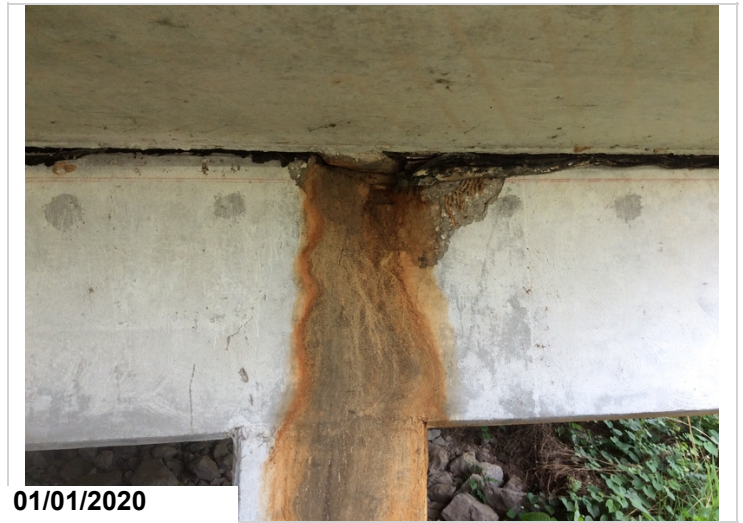
Spalling at key way bent 1 ahead side above column #1.
