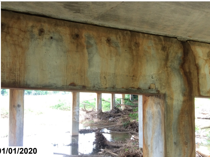
Horizontal cracking at bent #2 behind side.
