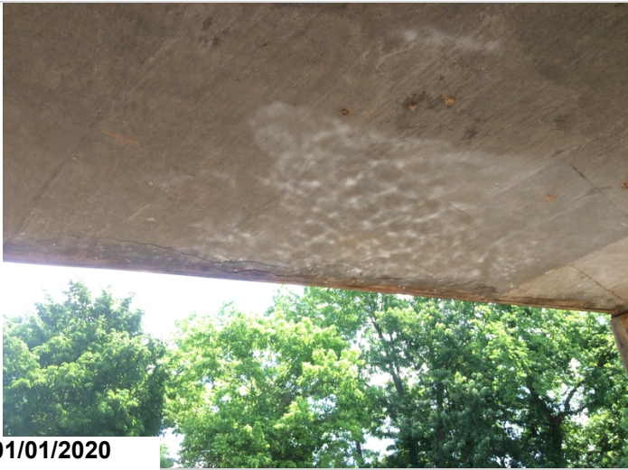
Cracking and delaminated areas typical to the right side of deck undersurface.
