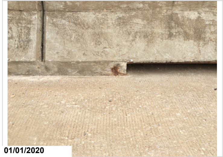
Span #6 railing right has spalling with steel exposed at the base of parapet.
