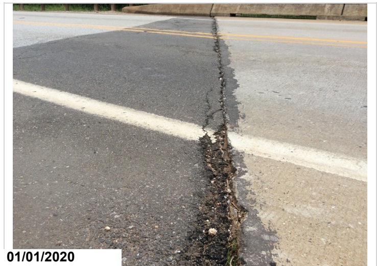
Abutment #2 has leveling at the approach roadway.
