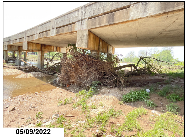
Large drift has wedge against substructure causing localized scour.
