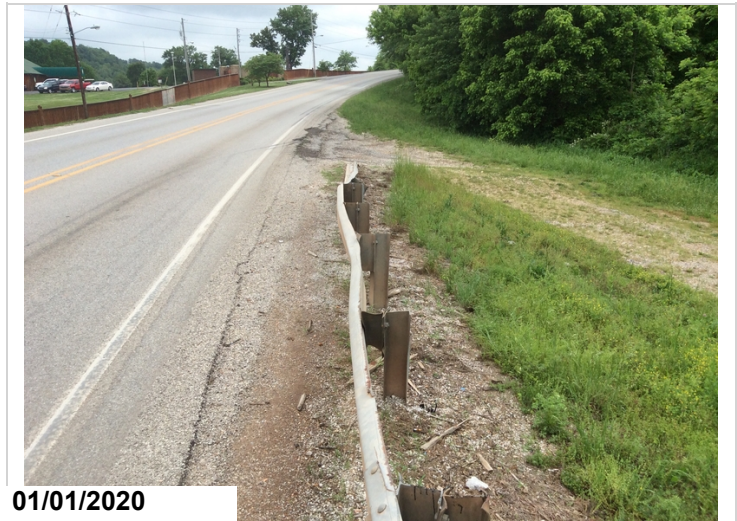
Abutment #2 right approach railing has vehicle damage.
