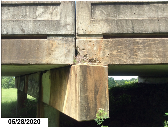
Typical spalling of deck over bent caps on the right side.
