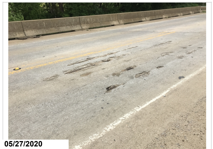
Span #3 spalling with steel exposed
