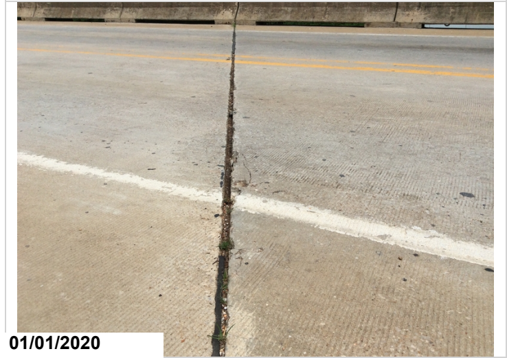
Deck bent #2 construction joint - joint material is missing.
