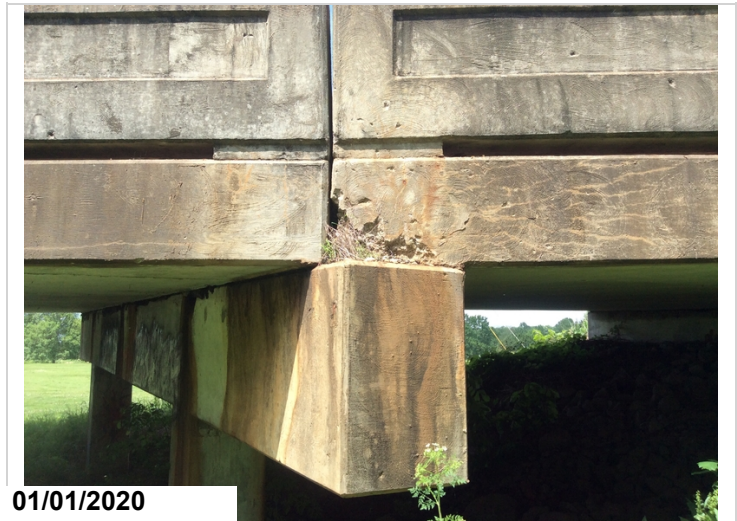
Typical spalling of deck over bent caps on the right side.
