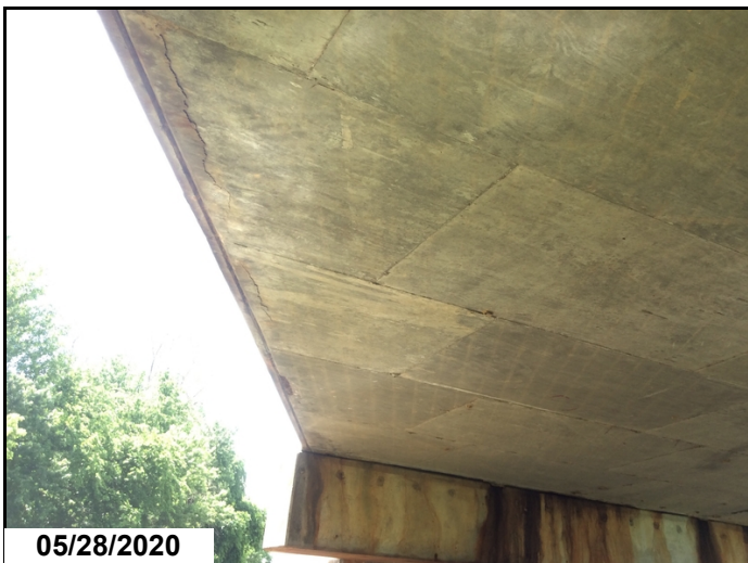
Typical view of right side undersurface of deck with cracking spalling and delaminations.
