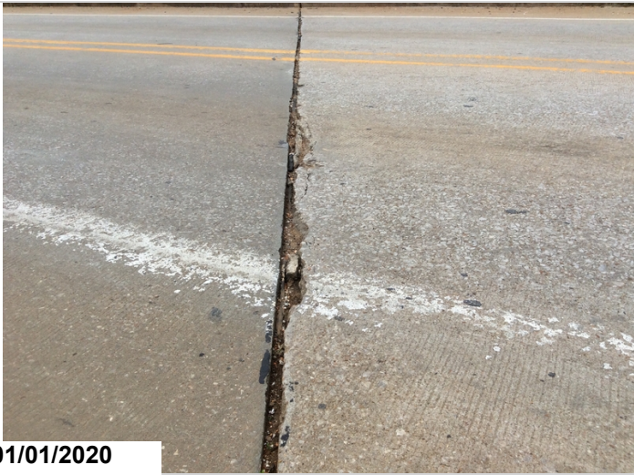
Bent #5 right spalling adjacent to construction joints.
