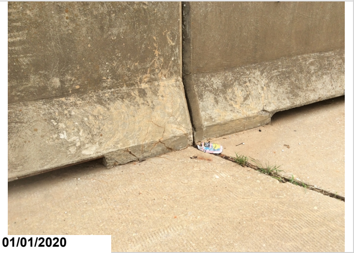
Bent #8 right deck and parapet - has area of map cracking.
