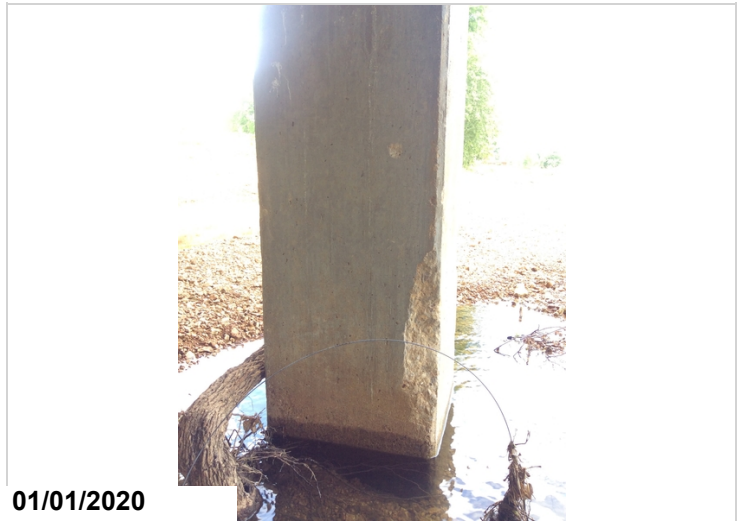
Bent #3 column #1 has spalling ahead side.
