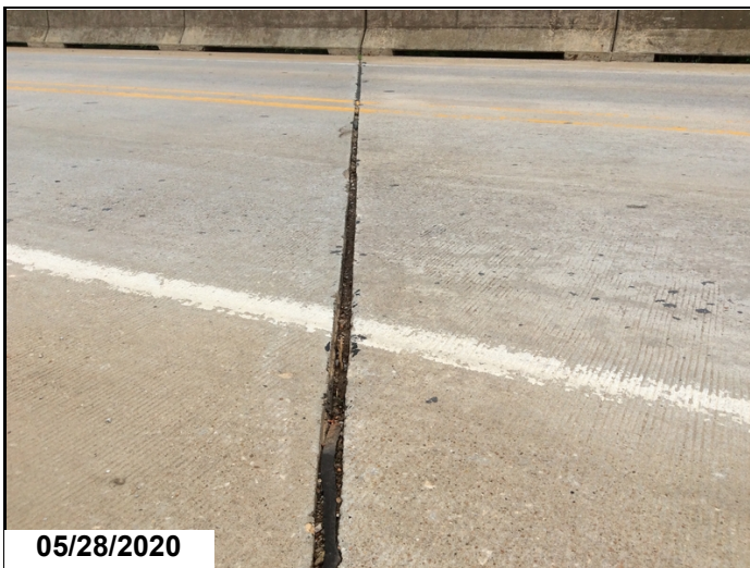
Bent #2 joint material missing.
