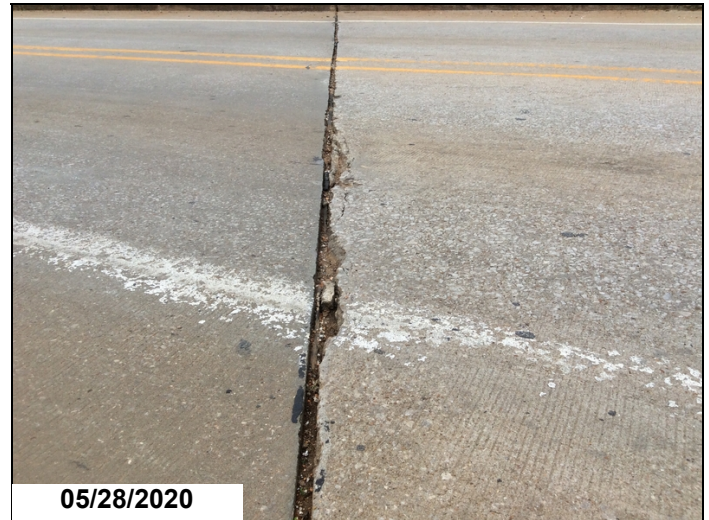
Bent #5 right spalling adjacent to construction joints.
