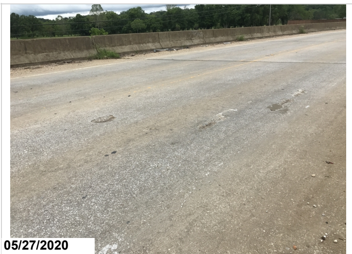
Spalling with steel exposed deck surface span #5.
