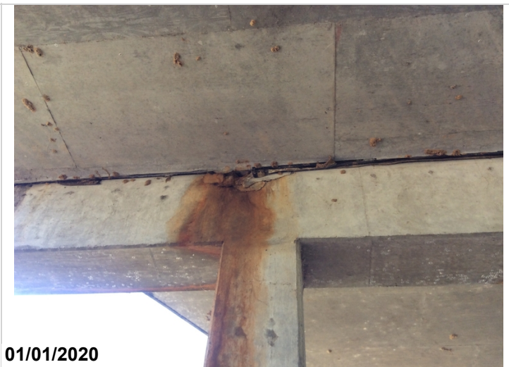
Bent #4 cap over column #1 behind side - spalling at keyway typical.
