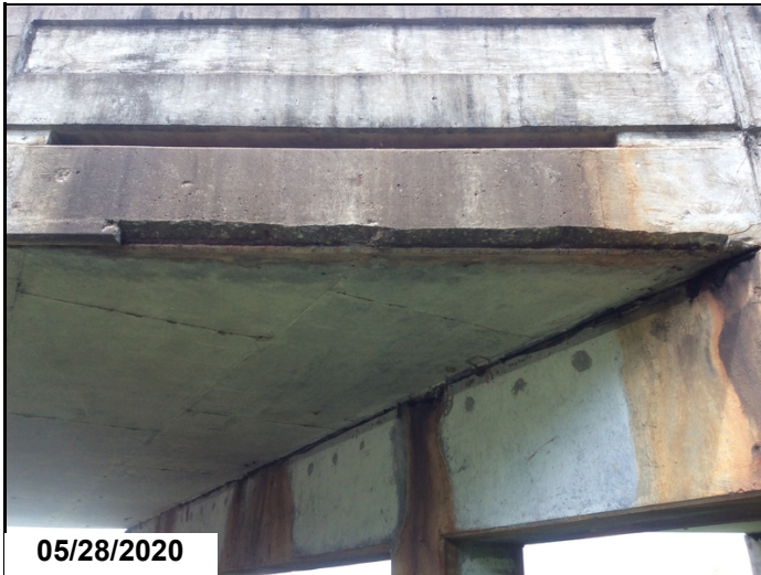
Span #7 right adjacent bent #7 spalling with steel exposed.
