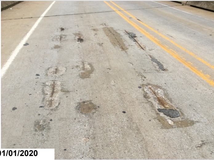
Span #3 left lane large spalls with steel exposed.
