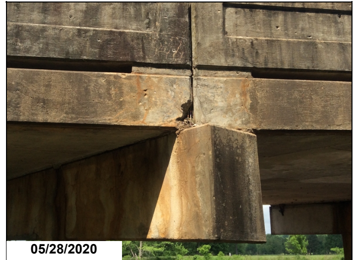
Spalling in side of deck above bent caps typical.
