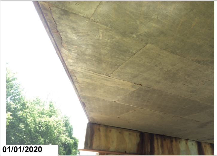
Typical view of right side undersurface of deck with cracking spalling and delaminations.
