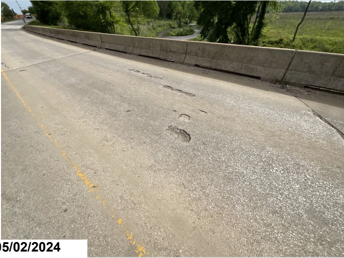
Span #5 right lane spalling with steel exposed
