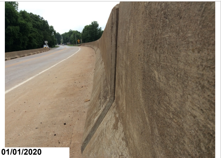
Parapet left railing has section that is not flush with rest of railing.
