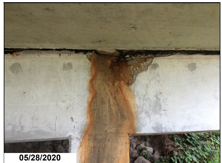
Spalling at key way bent #1 ahead side above column #1.
