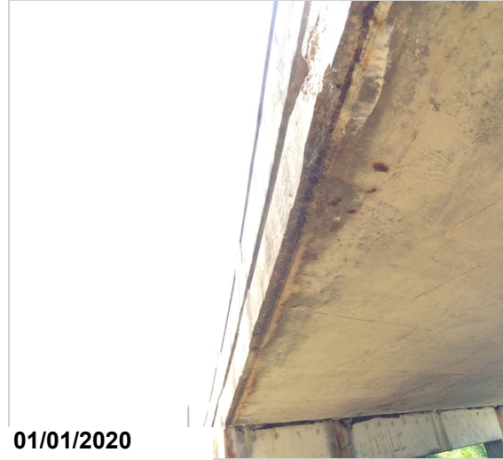
Deck span #2 right soffit has approximately 22' of spalling with steel exposed.
