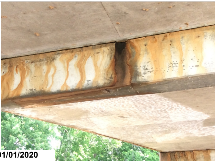
Bent #3 cap underneath spalling with steel exposed.
