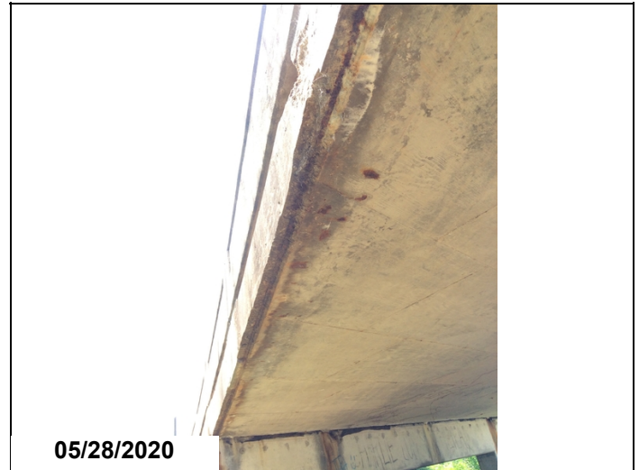
Deck span #2 right soffit has approximately 22' of spalling with steel exposed.
