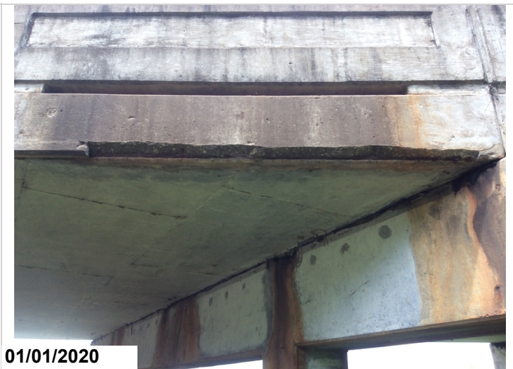
Span #7 right adjacent bent #7 spalling with steel exposed.
