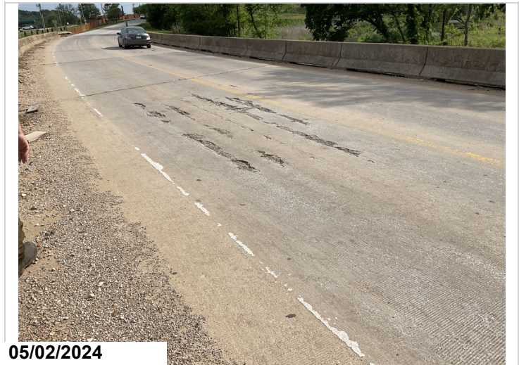
Span #3 spalling with steel exposed
