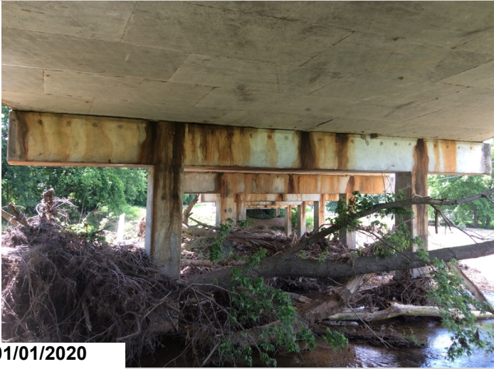
General view of bents leakage.
