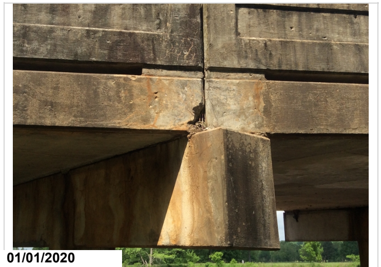
Spalling in side of deck above bent caps typical.
