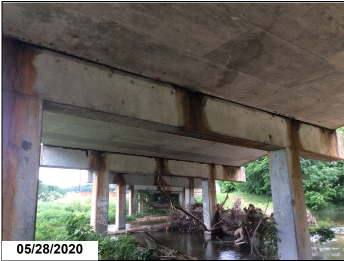
Exposed rebar at bent #3
