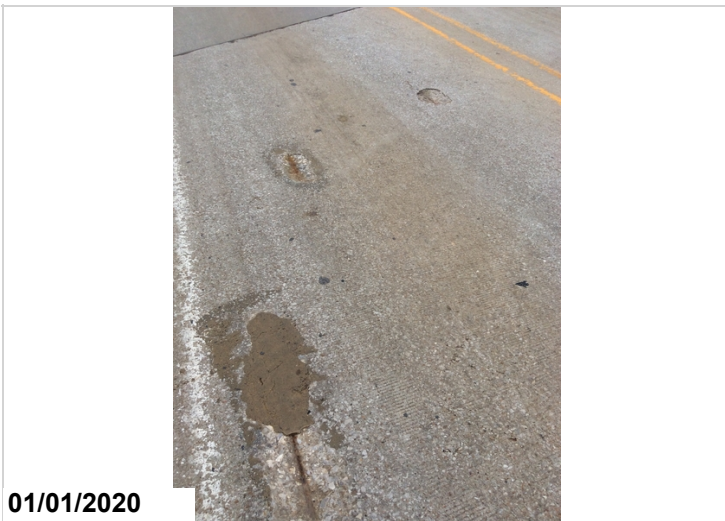
Span #5 right lane spalling with steel exposed.
