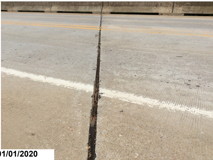
Bent #2 joint material missing.
