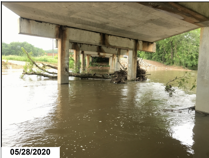
Span #5 channel has large trees causing localized scour.
