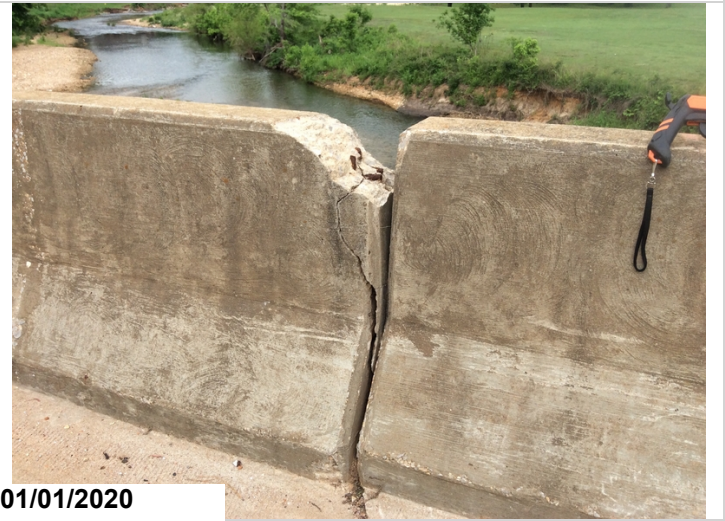
Deck railing left at bent #5 has large spall with steel exposed.
