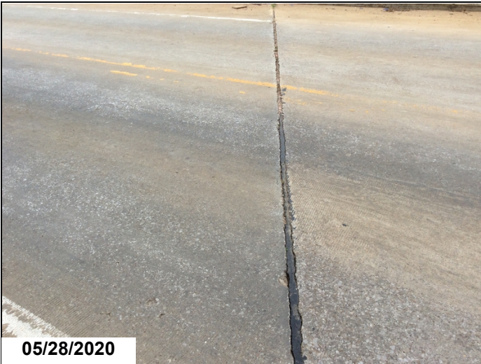
Joint seal condition over bent #1. Typical of all locations.
