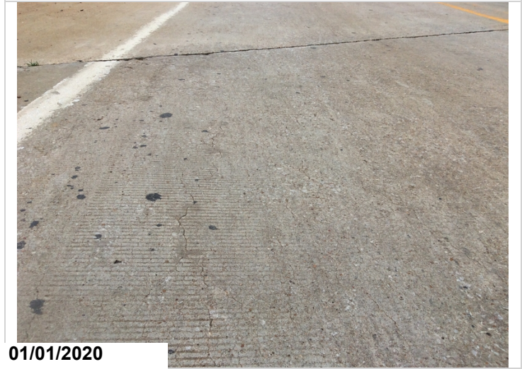
Span #1 deck cracking typical in wheel paths.
