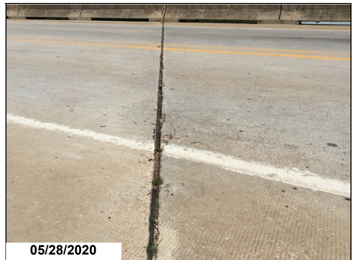
Deck bent #2 construction joint - joint material is missing.
